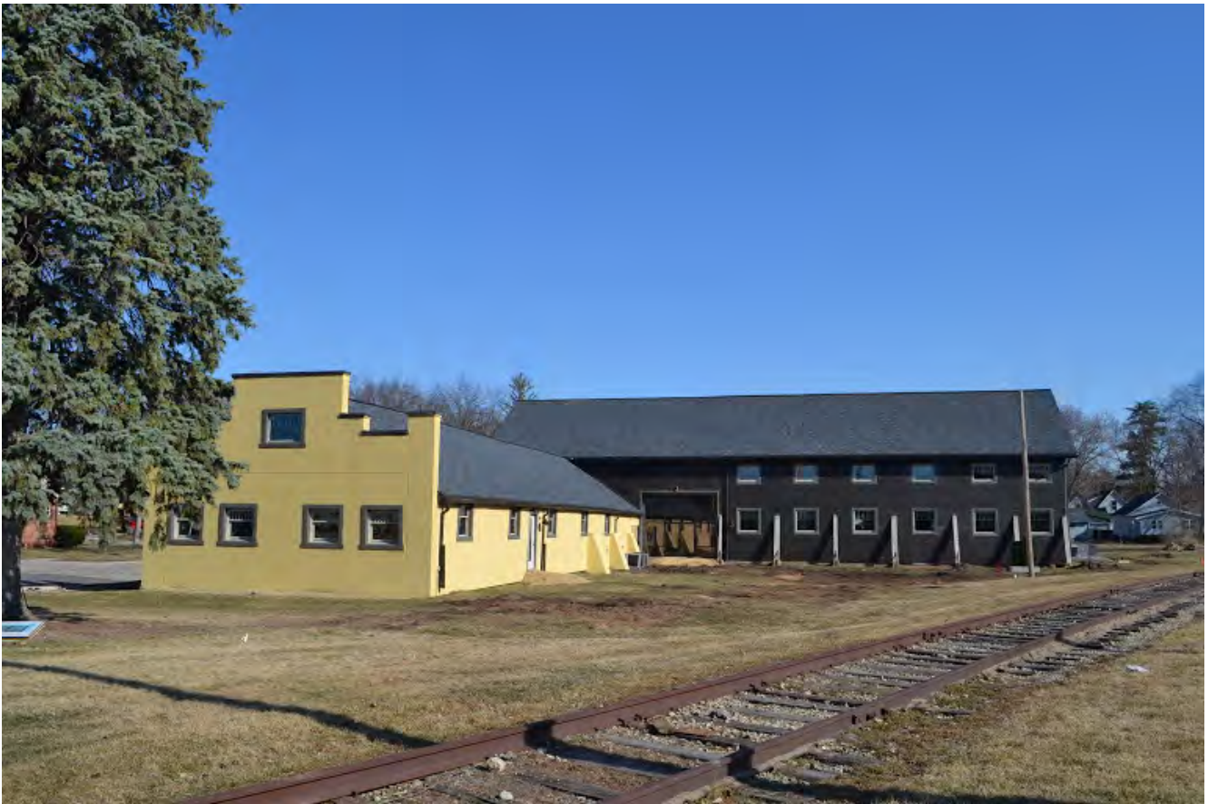
Figure 8 Rehabilitated south facades of showroom and workshop, 2015.
