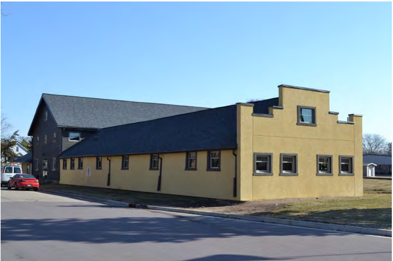
Figure 7 Rehabilitated south and west facades, 2015.
