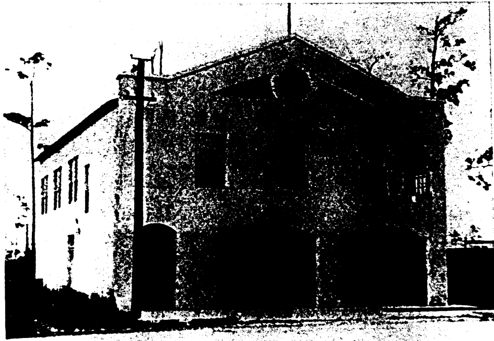
CIRCA 1915 HOMESTEAD FIRST POLICE AND FIRE STATION AND CITY HALL LOCATED ON THE CORNER OF N. E. 1st STREET AND EROCKE AVENUE.
