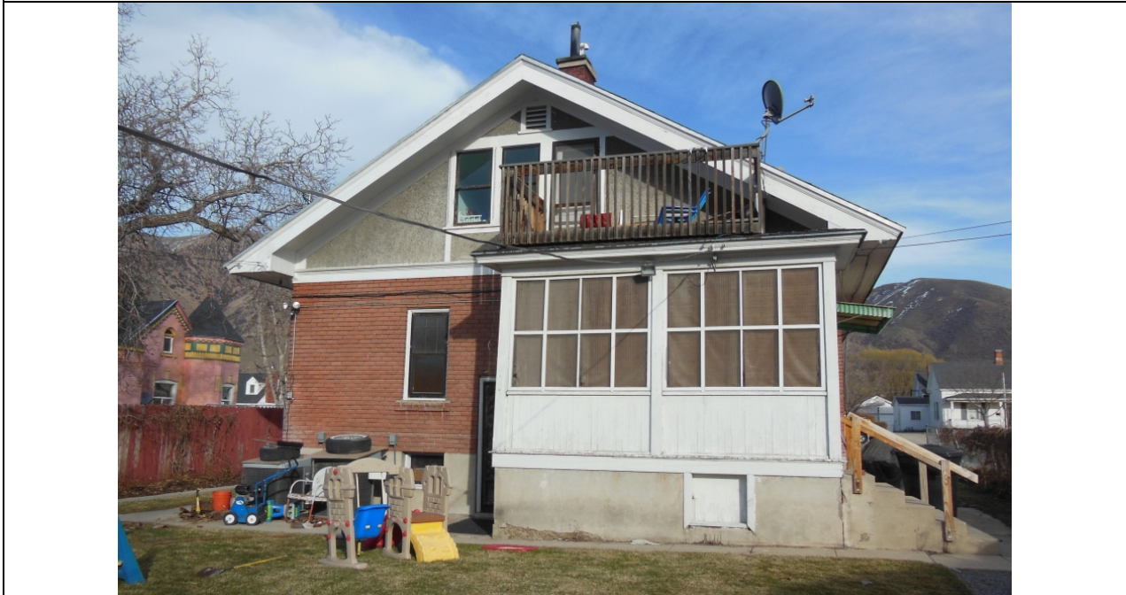
Photograph 4 West elevation, camera facing east. (photographed March 2014)
