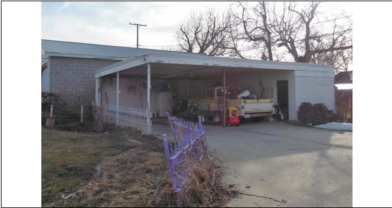
Photograph 5 Shed and carport, camera facing southwest. (photographed March 2014)
