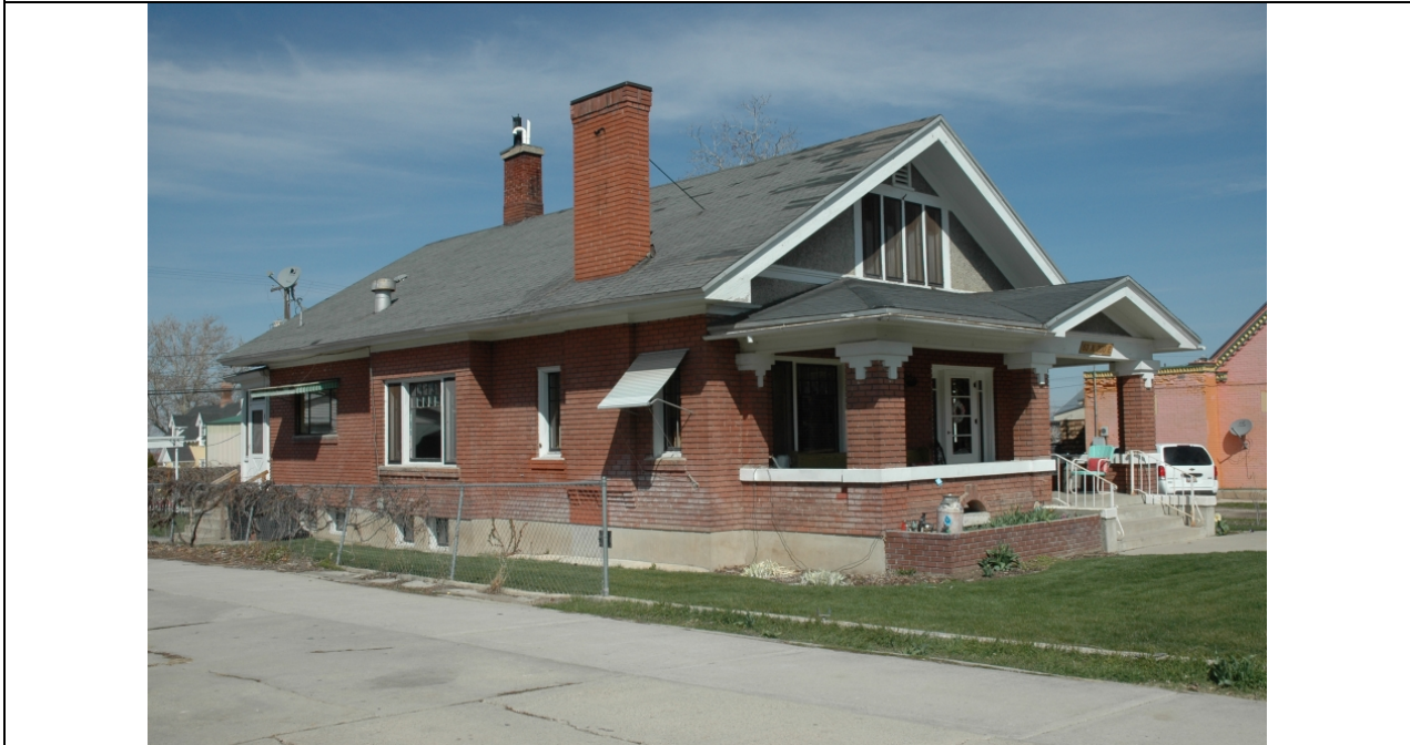
Photograph 2 East and south elevations, camera facing northwest. (photographed April 2014)
