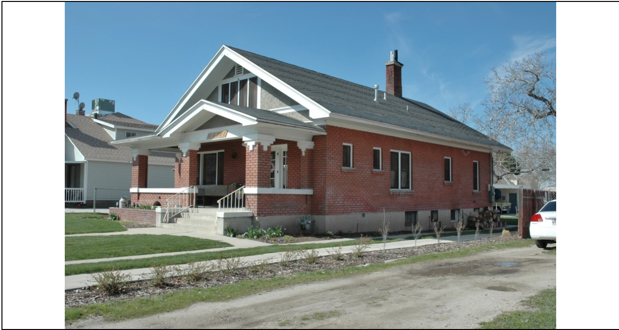
Photograph 3 East and north elevations, camera facing southwest. (photographed April 2014)
