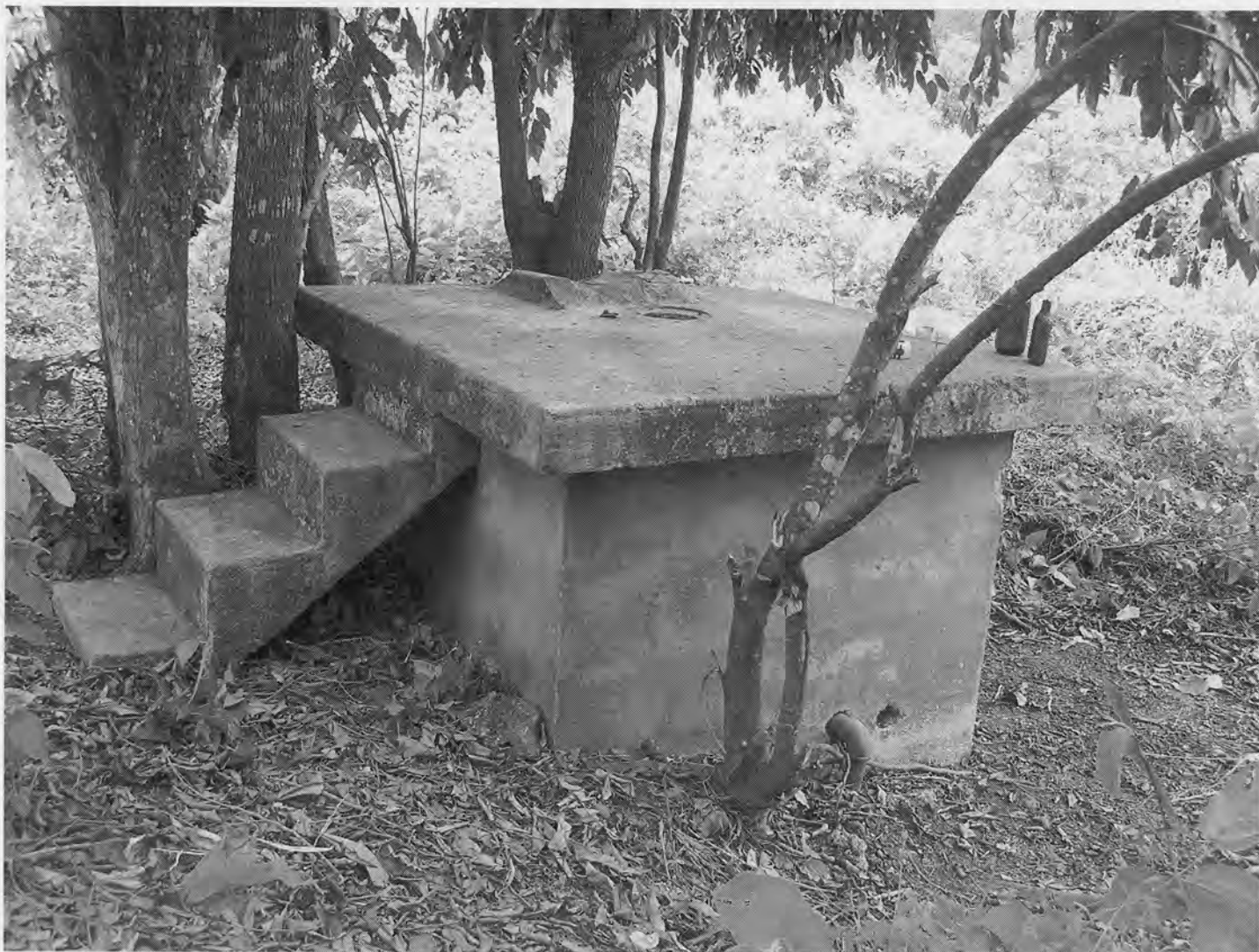
Cañada Well # 2 showing well house, platform, access steps, drain? pipe and artifacts (bottles). View is to the east.
