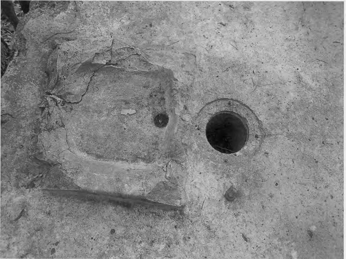
Cañada Well #2 showing details of platform: damaged basin, well casing and pump stand base plate impression, cleat.
