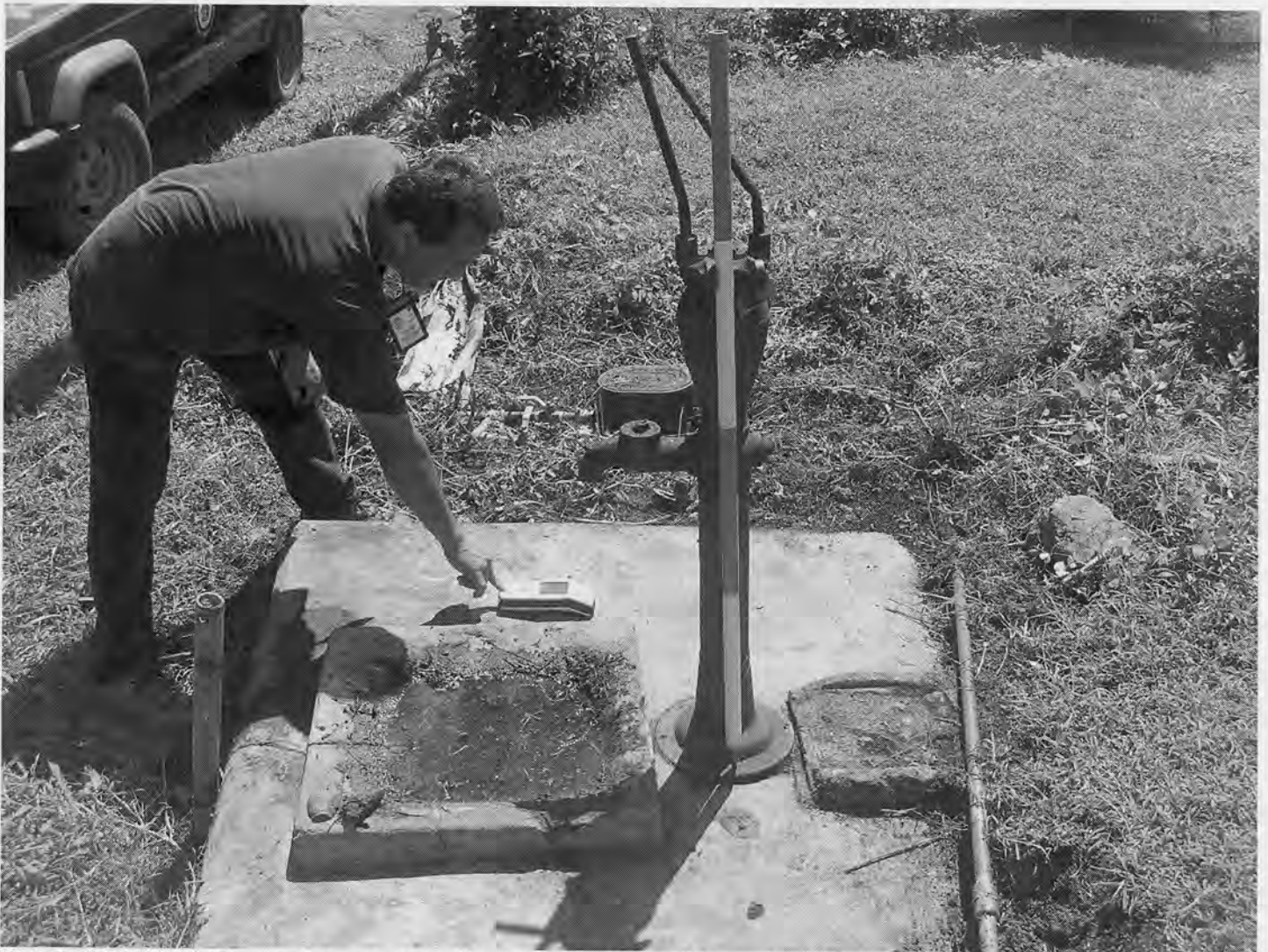
Cañada Well #1, platform and pump stand. Basin to left and possible mechanical pump foundation to right. View is to the northeast.
