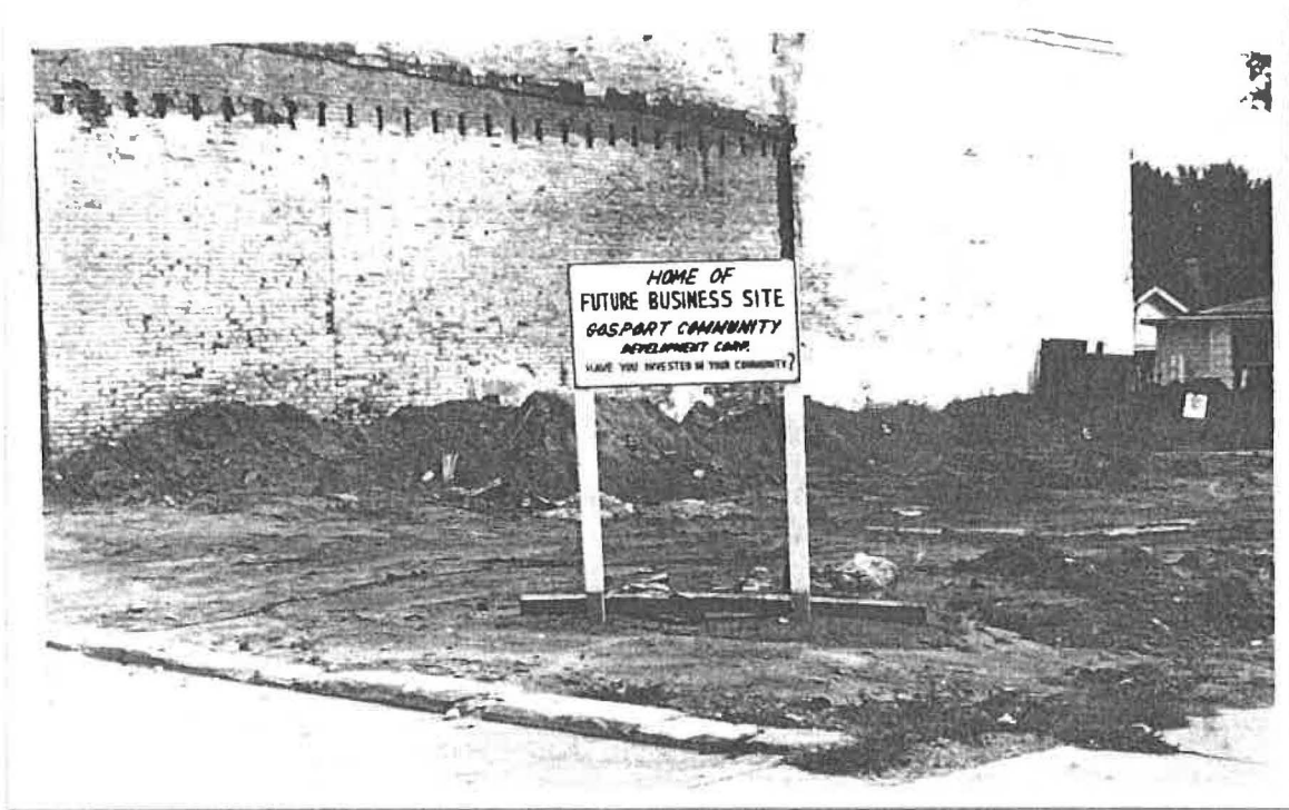
HP 16. Site where Value Market (resource 47) would be built, showing what remains of the east wall and rear portion of the former Dittmore store, 1970.
