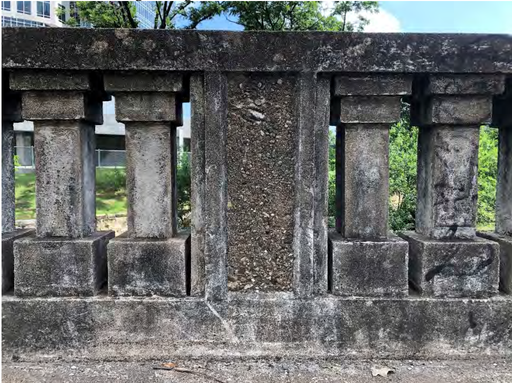
Photo 6: Detail of bridge railing. View north.
