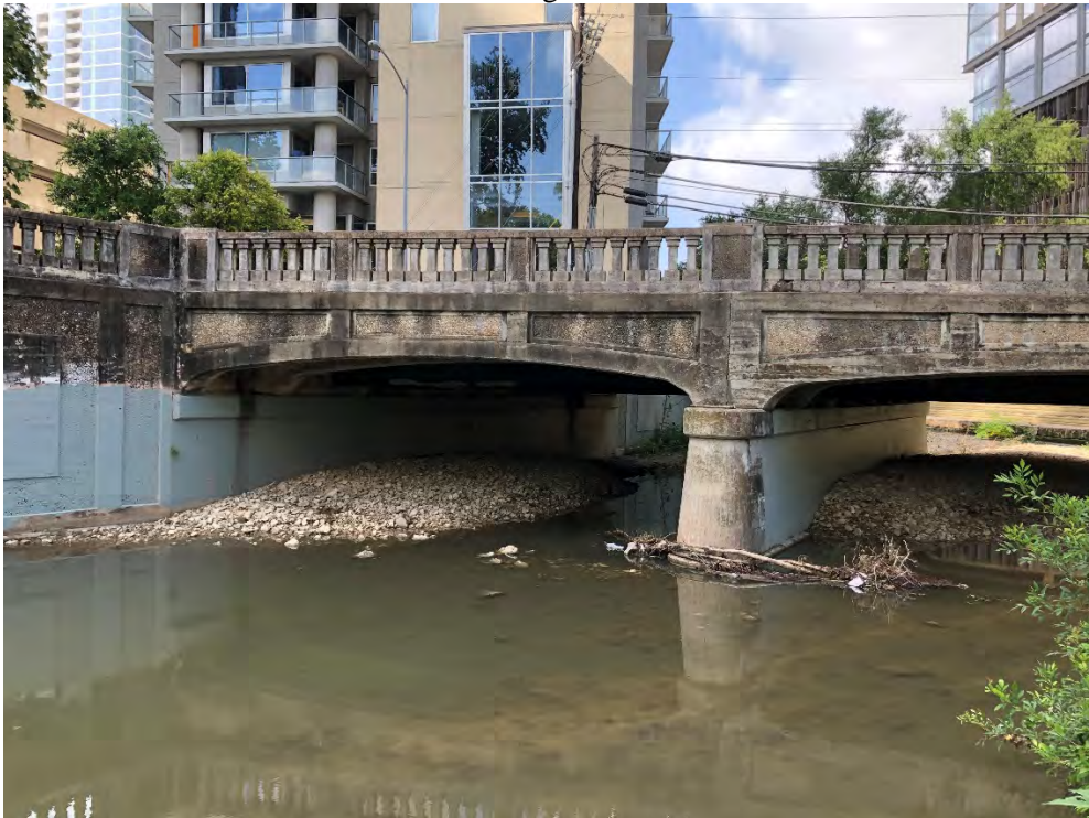
Photo 4: Partial view of north side of bridge. View south.
