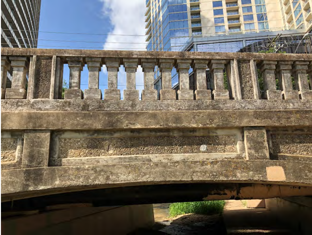
Photo 5: Detail, north side of bridge. View south.
