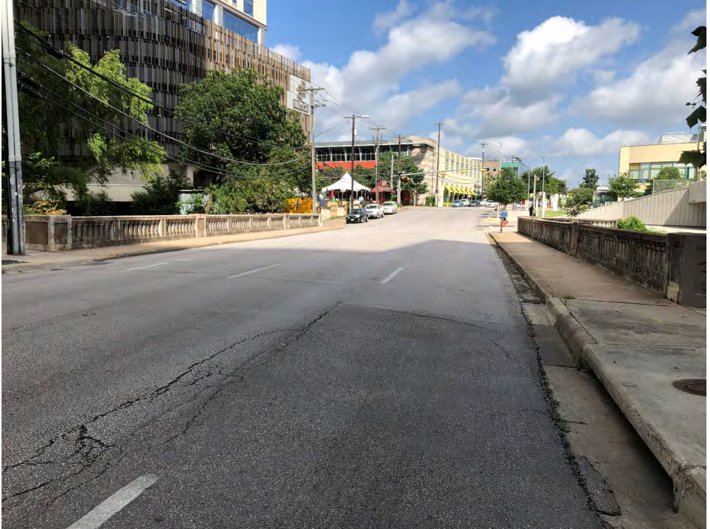
Photo 9: Roadway deck over West 5 th Street Bridge. View west.
