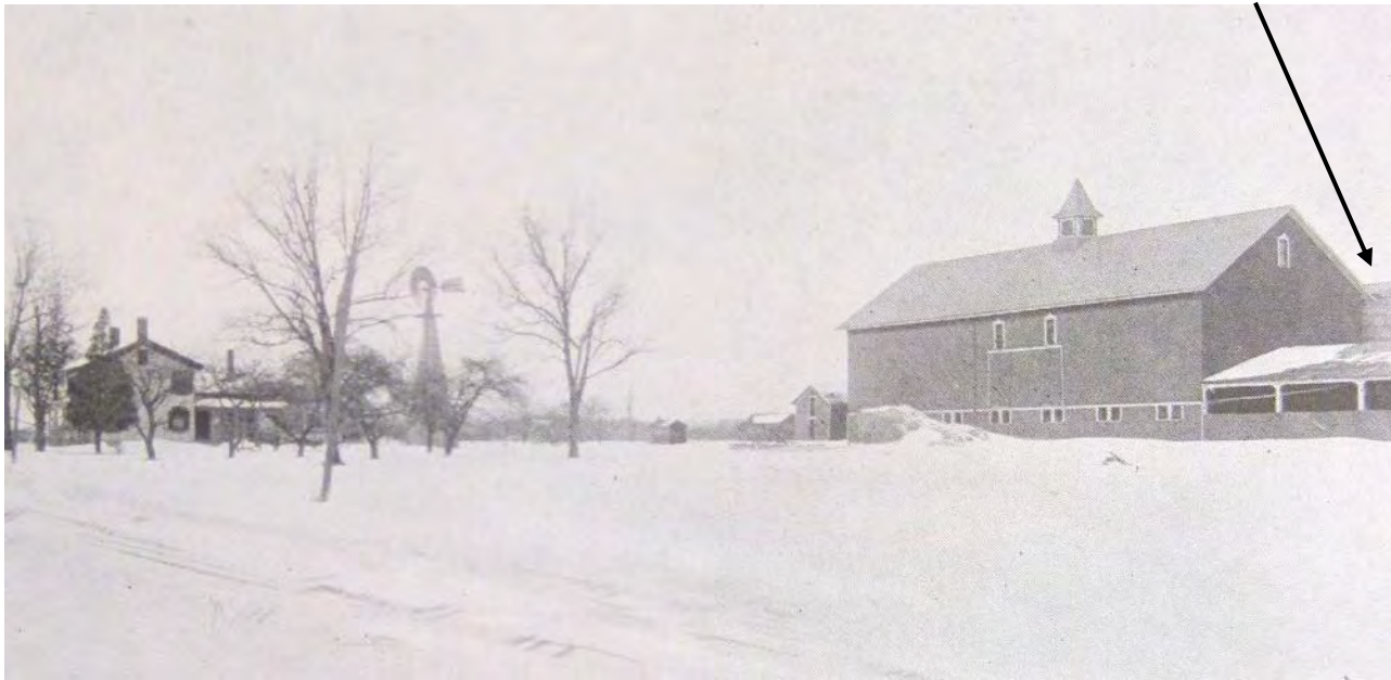
Figure 9. Case-Barlow Farm, Photo 1910 Concrete Stave Silo under construction, indicated by arrow
