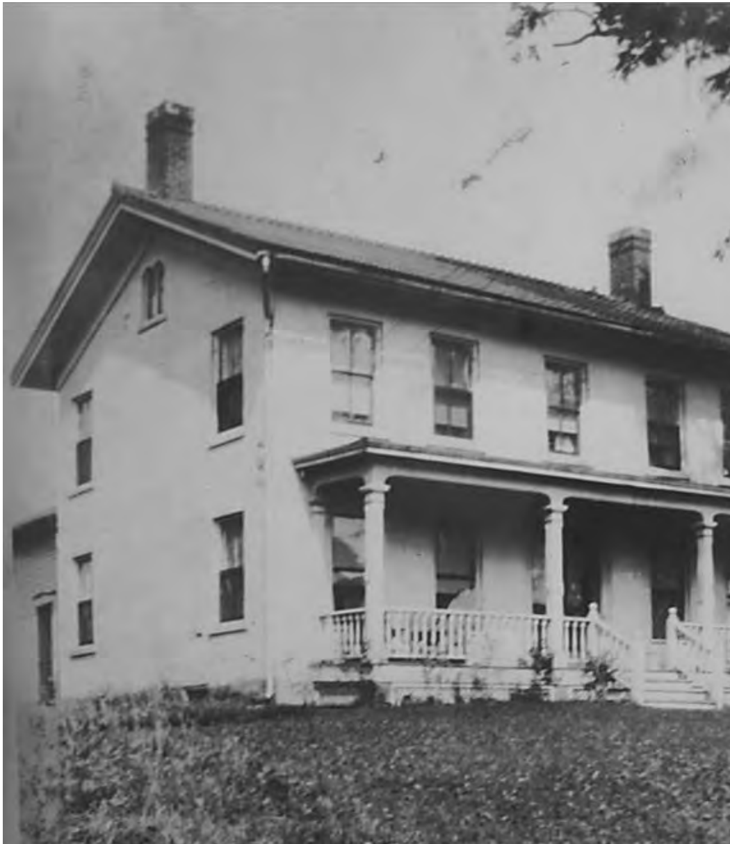
Figure 12. Case-Barlow Farm House, Photo ca. 1940
