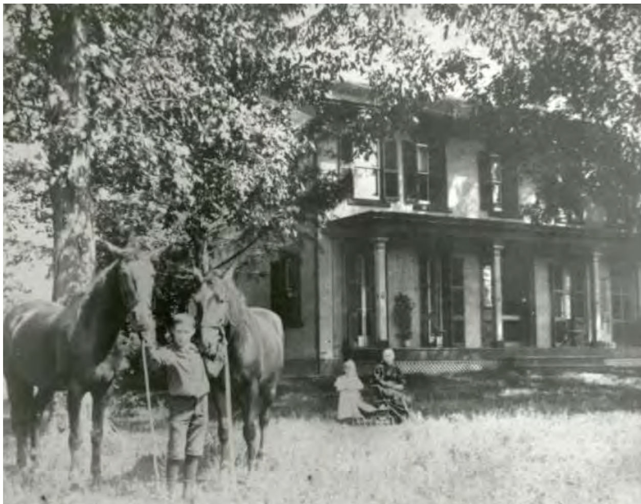
Figure 6. Case-Barlow Farm House, Photo ca. 1895
