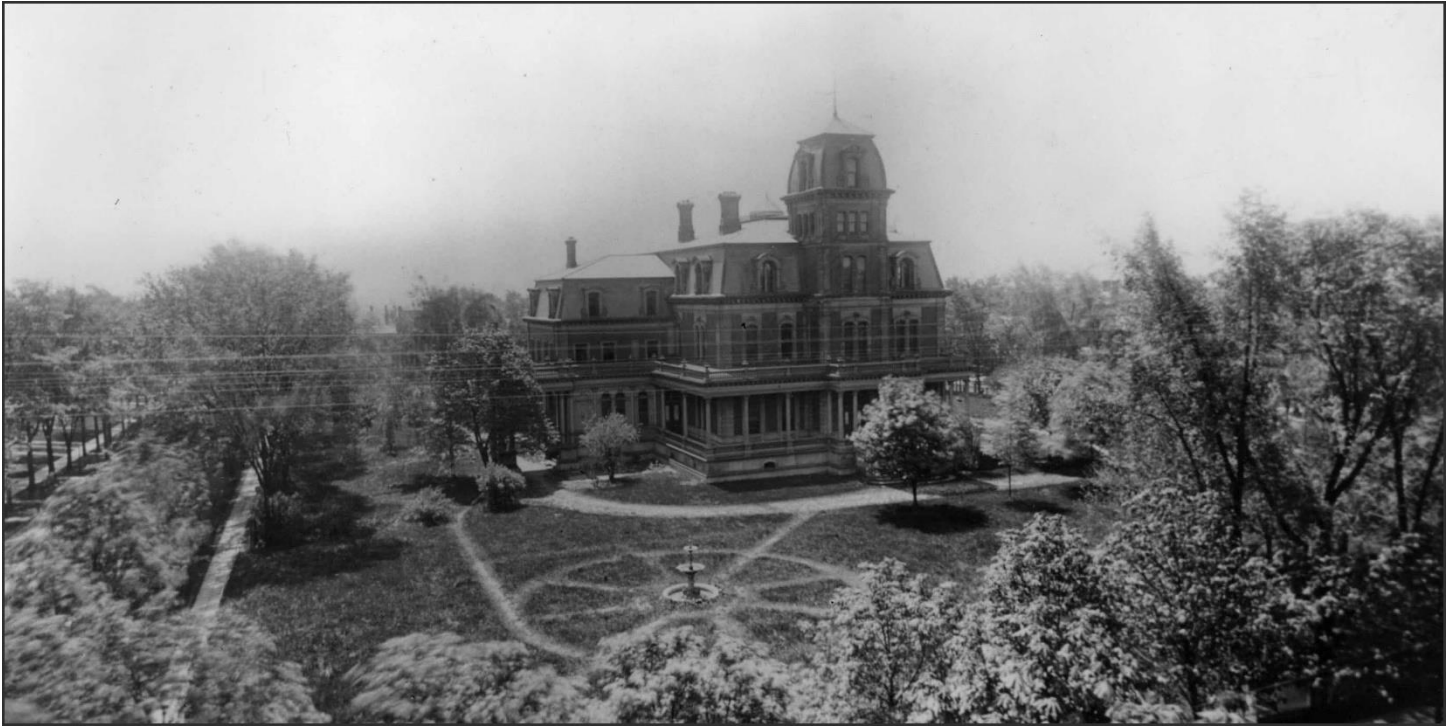
The William G. Fargo Estate (1868-1872), c. 1880 view from the north, looking south from the corner of Jersey Street and West Avenue (which is visible at left).
