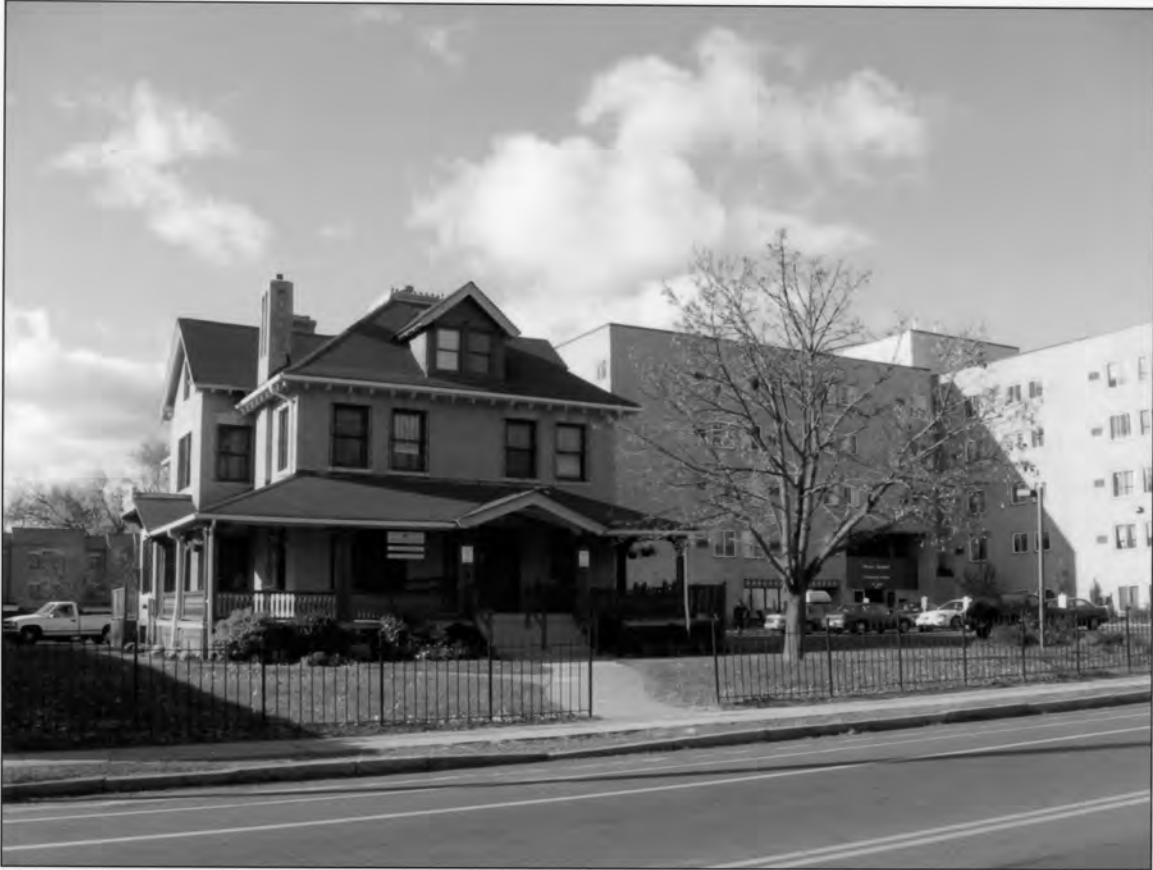
Photo 0016: View looking northwest from Vine St. between Albany Ave. & Mather St.
