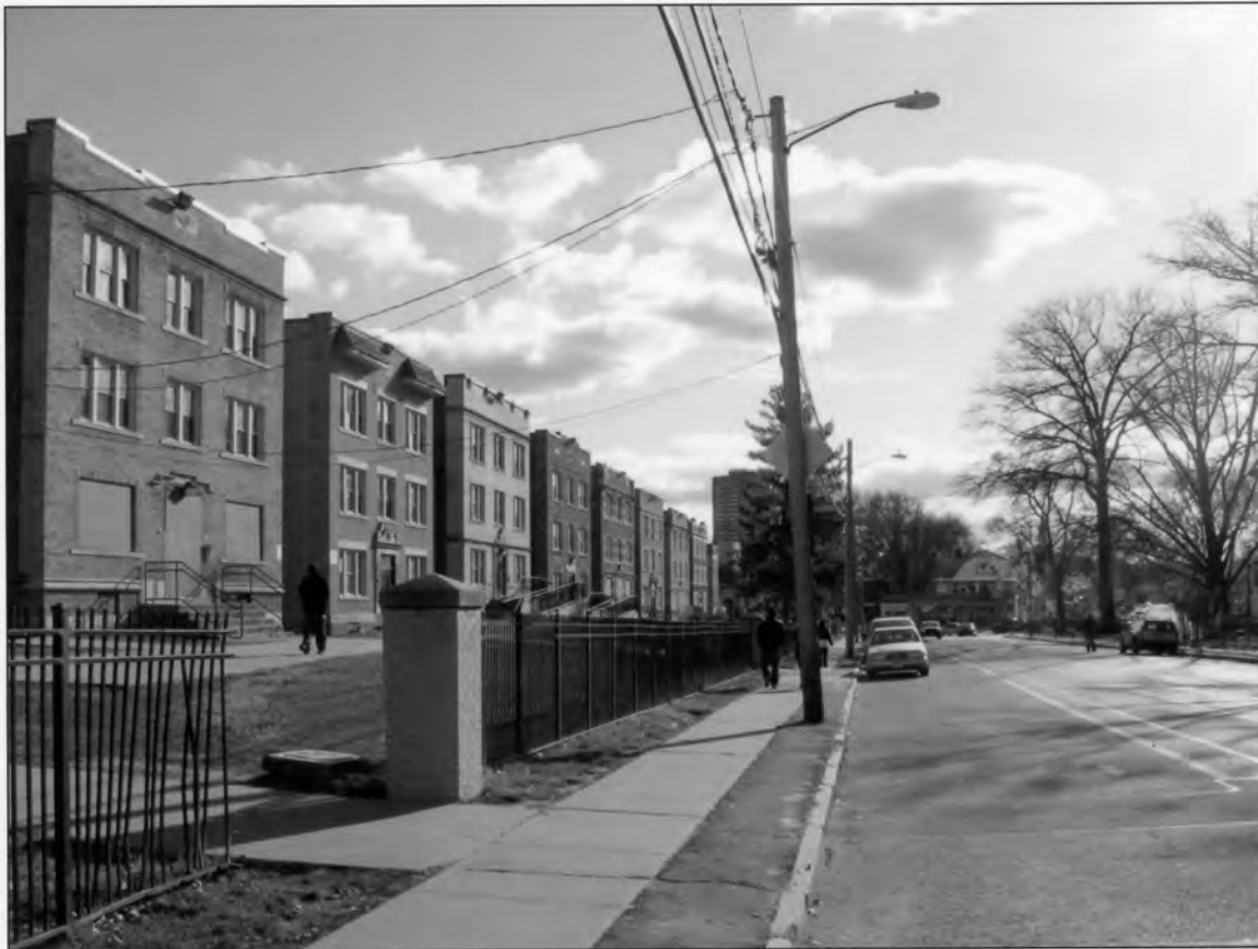
Photo 00002: View of Vine St. apartments blocks, Hartford, looking southwest (left to right: #32-24, #28-30, #24-26, #22-20, #16-18, 12-14, 8-10, #4-6)
