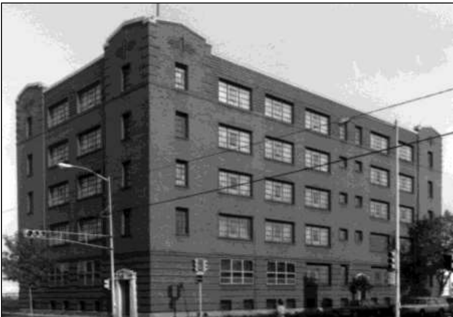
FIGURE 2: Klueter & Company Wholesale Grocery Warehouse, 1984 photograph.
