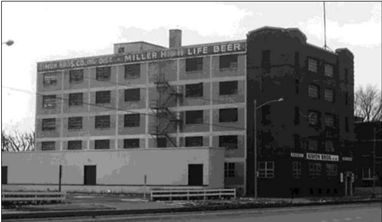
FIGURE 3: Klueter & Company Wholesale Grocery Warehouse, 1974 photograph.
