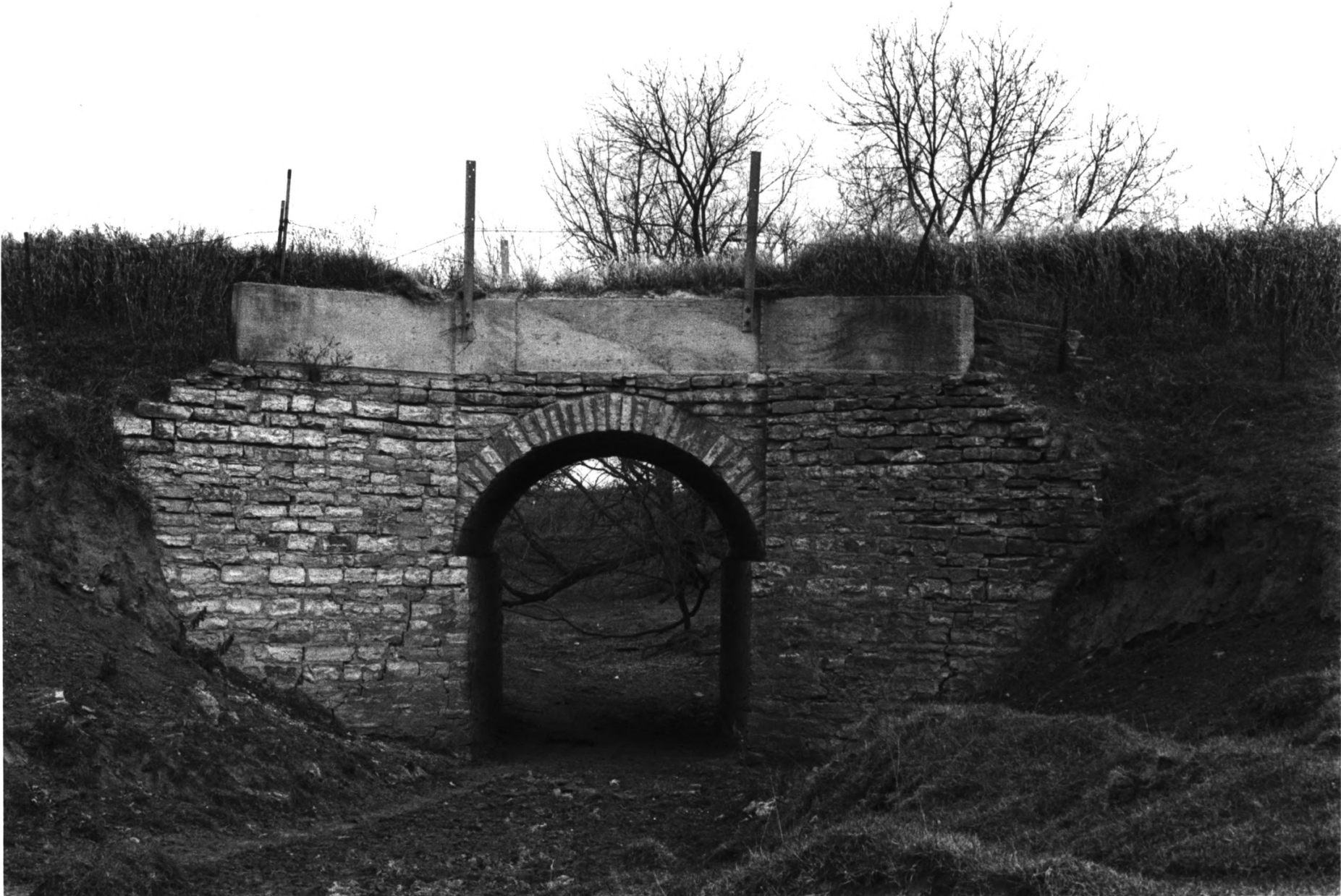
FOUNTAIN TOWNSHIP STONE-ARCH BRIDGE FILLMORE CO., MN PHOTO I.D. 09369#5
