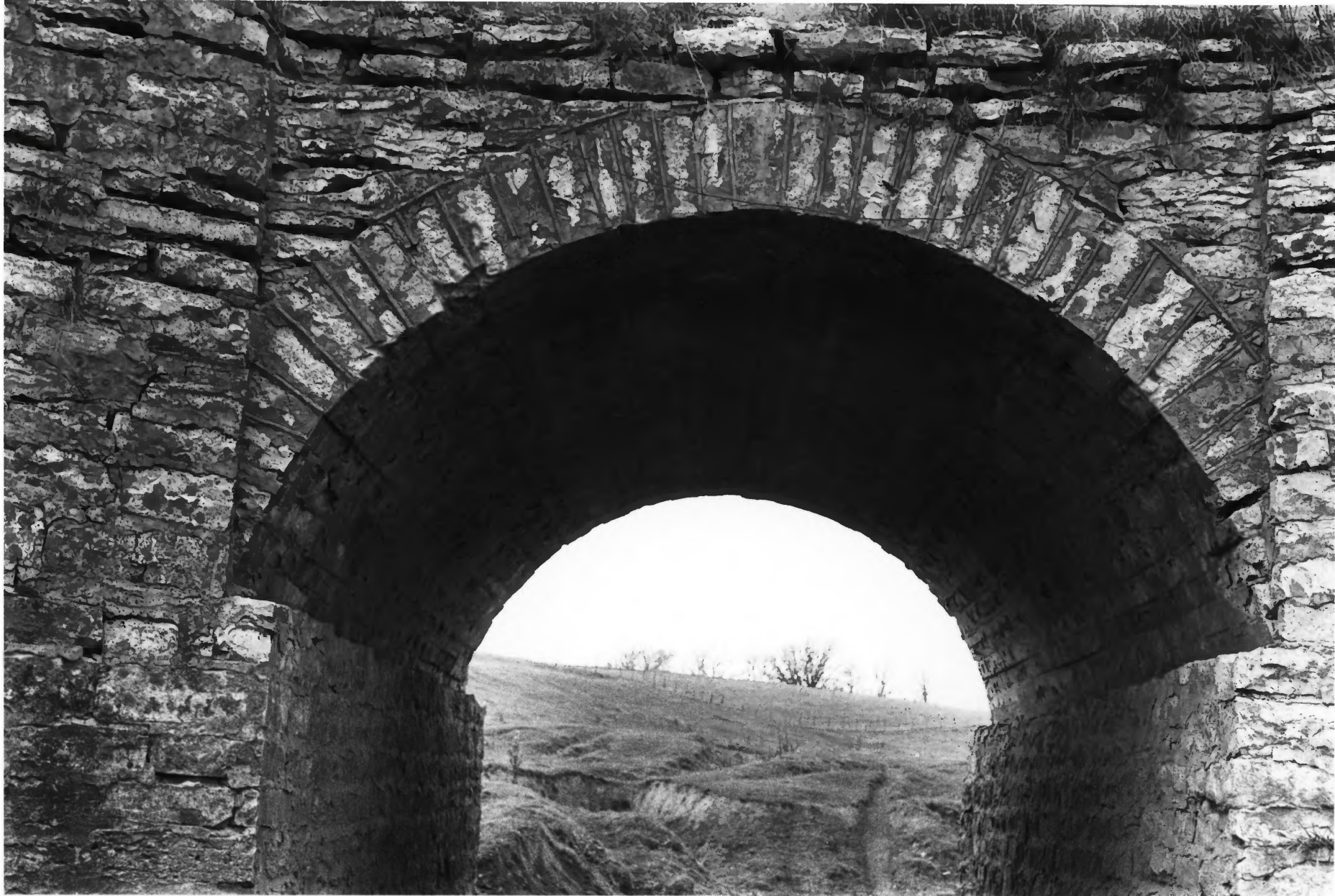
FOUNTAIN TOWNSHIP STONE-ARCH BRIDGE FILLMORE CO., MN PHOTO I.D. 09369 # 7
