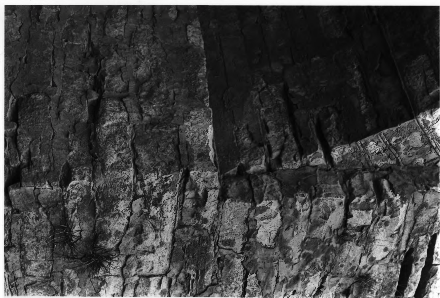
FOUNTAIN TOWNSHIP STONE-ARCH BRIDGE FILLMORE CO., MN PHOTO I.D. 09369#6
