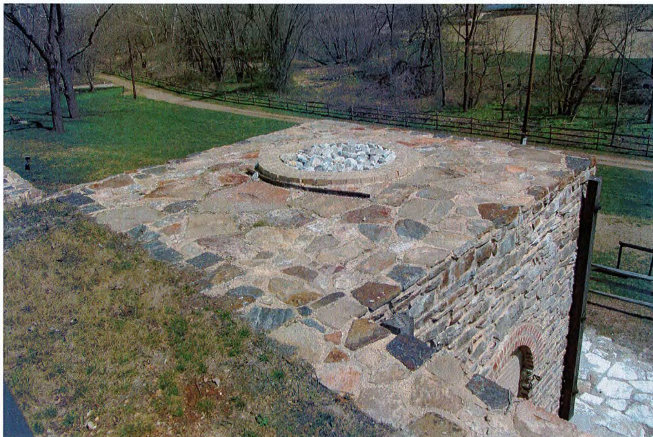
MD_BaltimoreCounty_LimeKilnBottom_0010.tif Kiln 3 – upper shaft showing infilled chimney, view from above (southeast)
