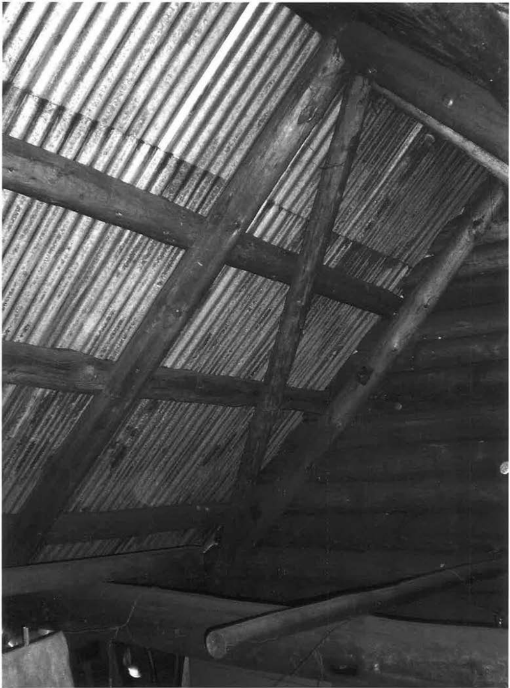
CA_Tuolumne County_Lake Vernon Snow Survey Shelter_0005
