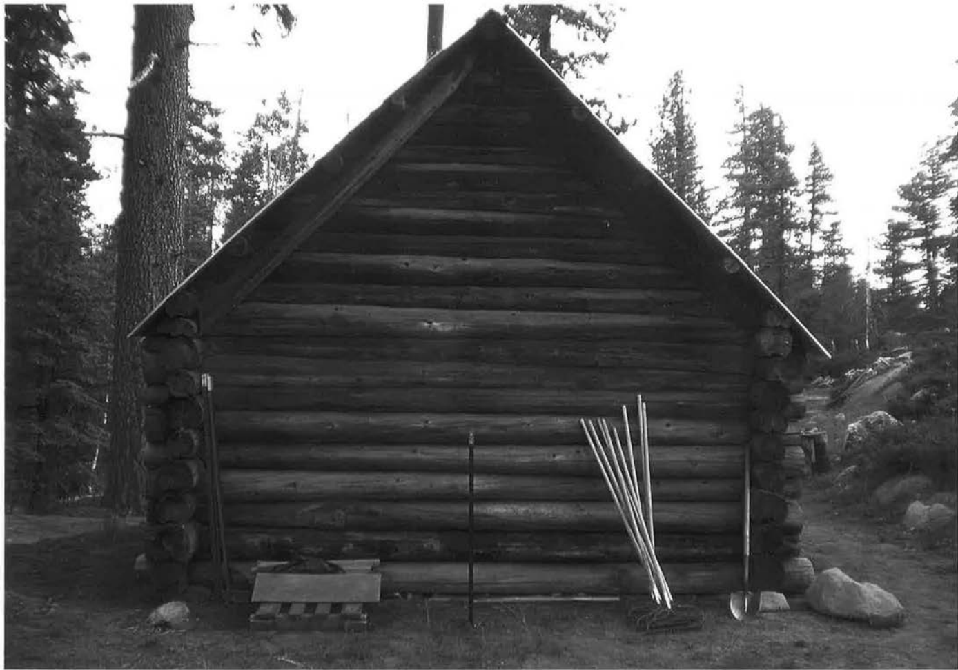
CA_Tuolumne County_Lake Vernon Snow Survey Shelter_0002
