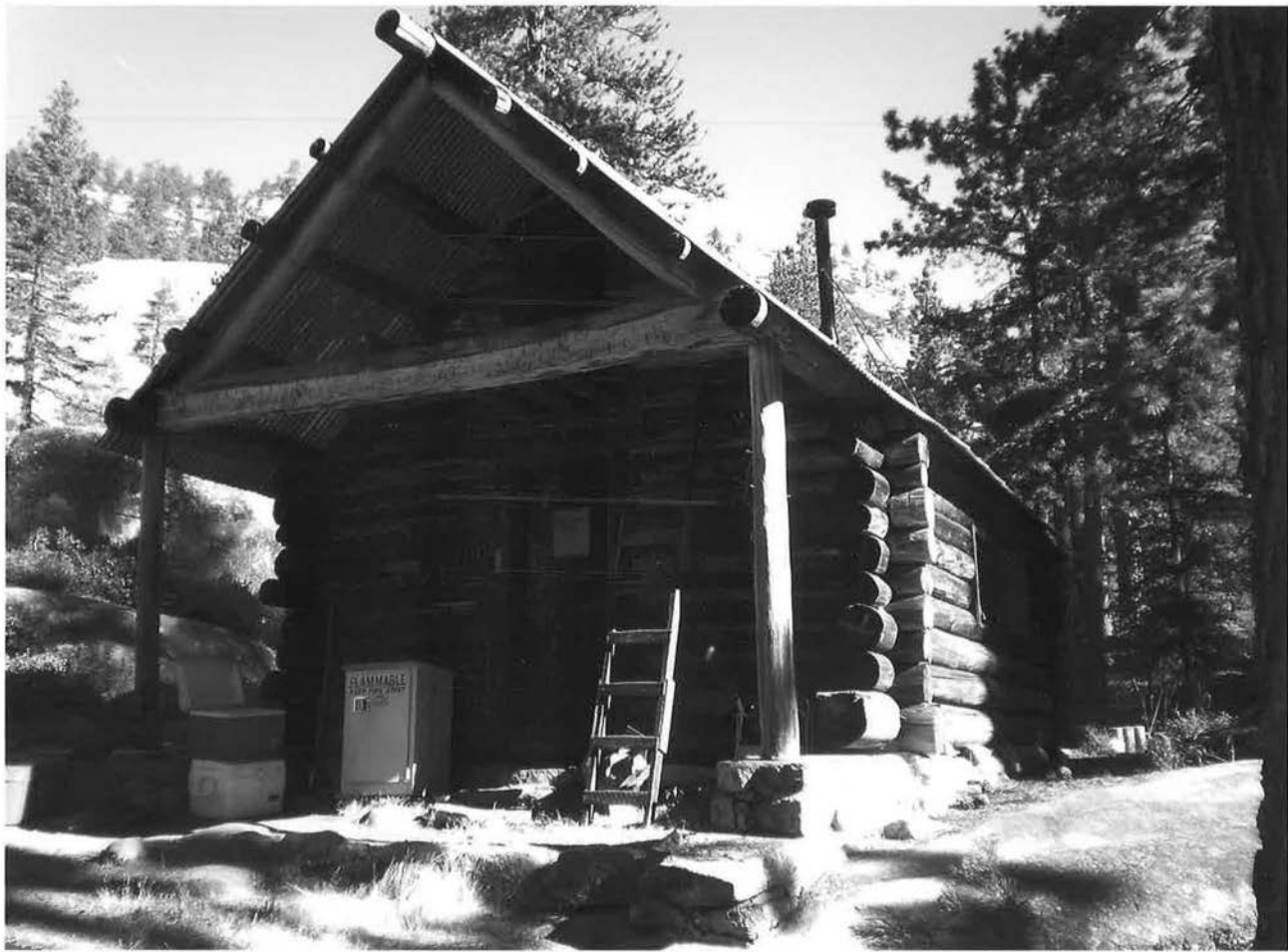
CA_Tuolumne County_Lake Vernon Snow Survey Shelter_0001
