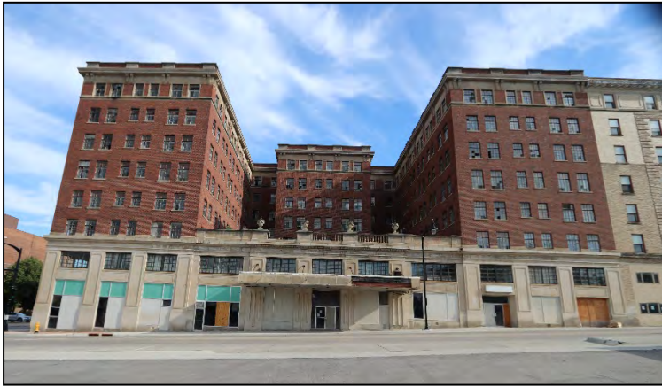
Figures 13 & 14: Contemporary views of the Warden Shops and Apartment Building (red brick). A portion of the Wahkonsa Annex can be seen to the right (buff brick). Note that the fenestration of the Warden is multi-paned industrial as opposed to the double-hung of the Wahkonsa Annex. Source: Strata Architecture, 2017
