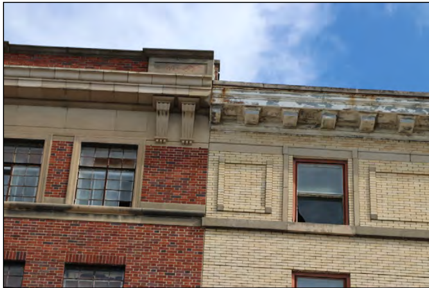
Figures 13 & 14: Contemporary views of the Warden Shops and Apartment Building (red brick). A portion of the Wahkonsa Annex can be seen to the right (buff brick). Note that the fenestration of the Warden is multi-paned industrial as opposed to the double-hung of the Wahkonsa Annex. Source: Strata Architecture, 2017
