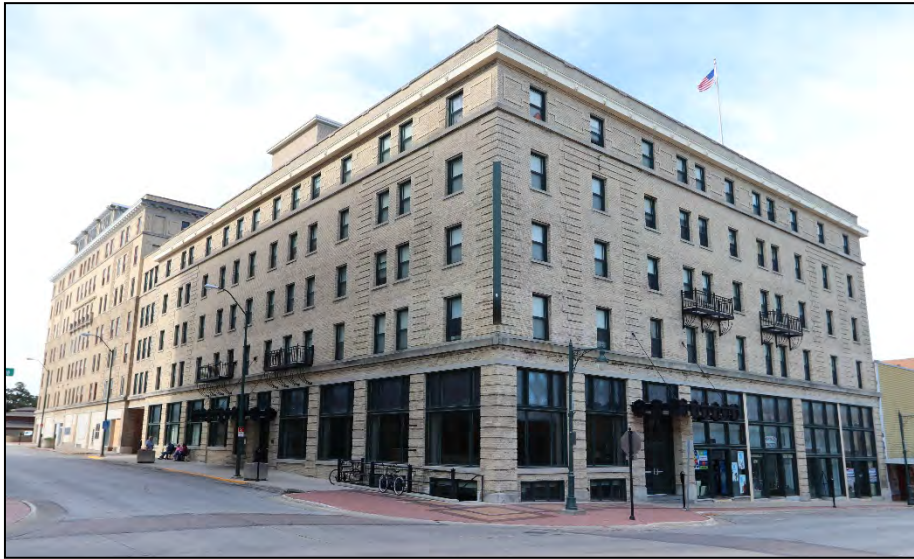
Figure 4: Contemporary view of The Wahkonsa (foreground) and the Wahkonsa Annex. Note that the fenestration of The Wahkonsa are replicated in the Annex.
