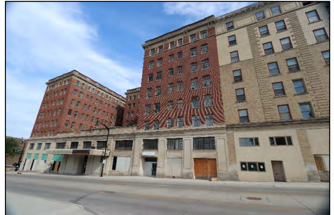
Figures 13 & 14: Contemporary views of the Warden Shops and Apartment Building (red brick). A portion of the Wahkonsa Annex can be seen to the right (buff brick). Note that the fenestration of the Warden is multi-paned industrial as opposed to the double-hung of the Wahkonsa Annex. Source: Strata Architecture, 2017
