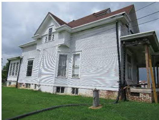
east facade along Lafayette Street
