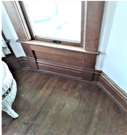
panels below all first-floor windows
