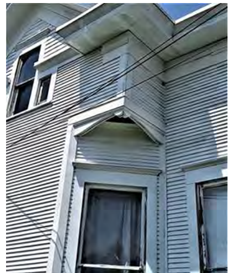
corner section over east side window
