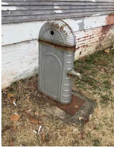
chain well pump – east side
