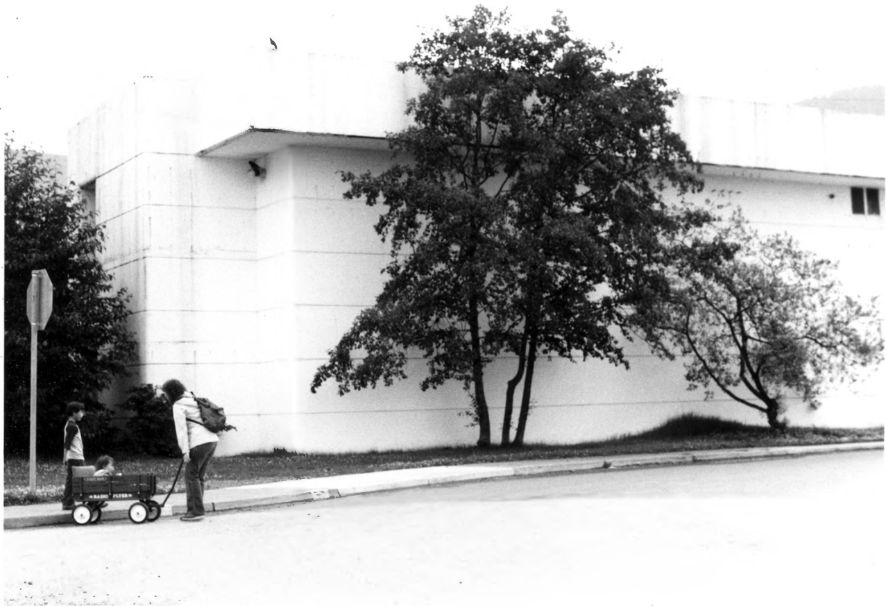
3. Sitka Naval Air Station. Bombproof power plant, similar to ones at naval bases at Kodiak and Dutch Harbor.
