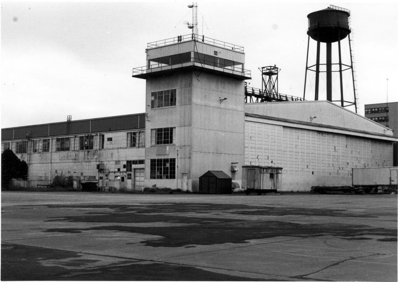
1. Sitka Naval Air Station. One of two hangars and control tower. The paved area in front was both aircraft parking and a short runway fitted out like an aircraft carrier's flight deck.
