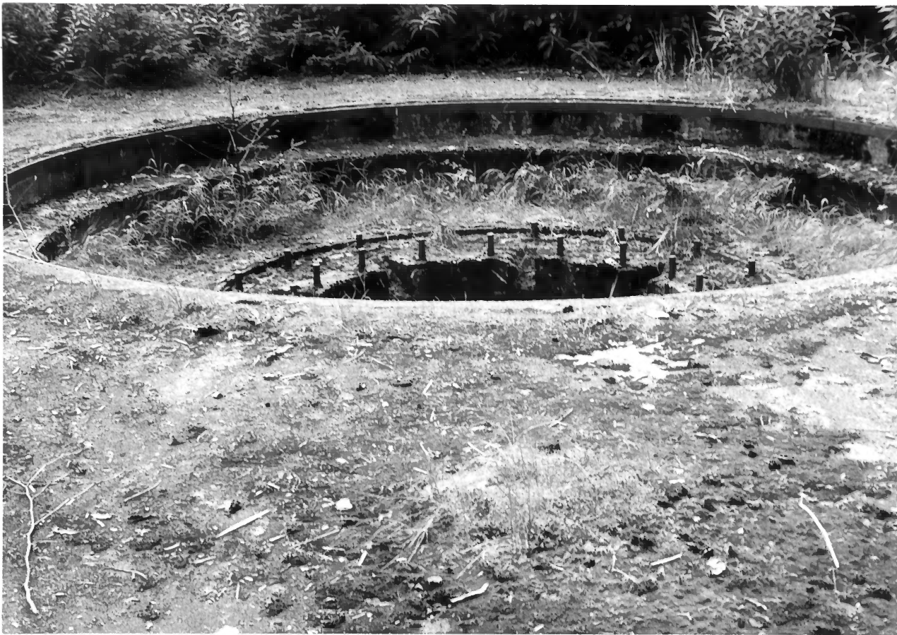
6. One of two 6-inch gun emplacements at Fort Rousseau, Makhnati Island. This was the only fixed 6-inch battery completed at Sitka.
