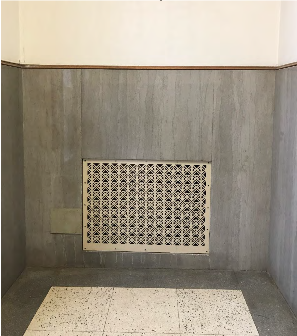
Photo 12: Marble wainscot in vestibule. Camera facing west.
