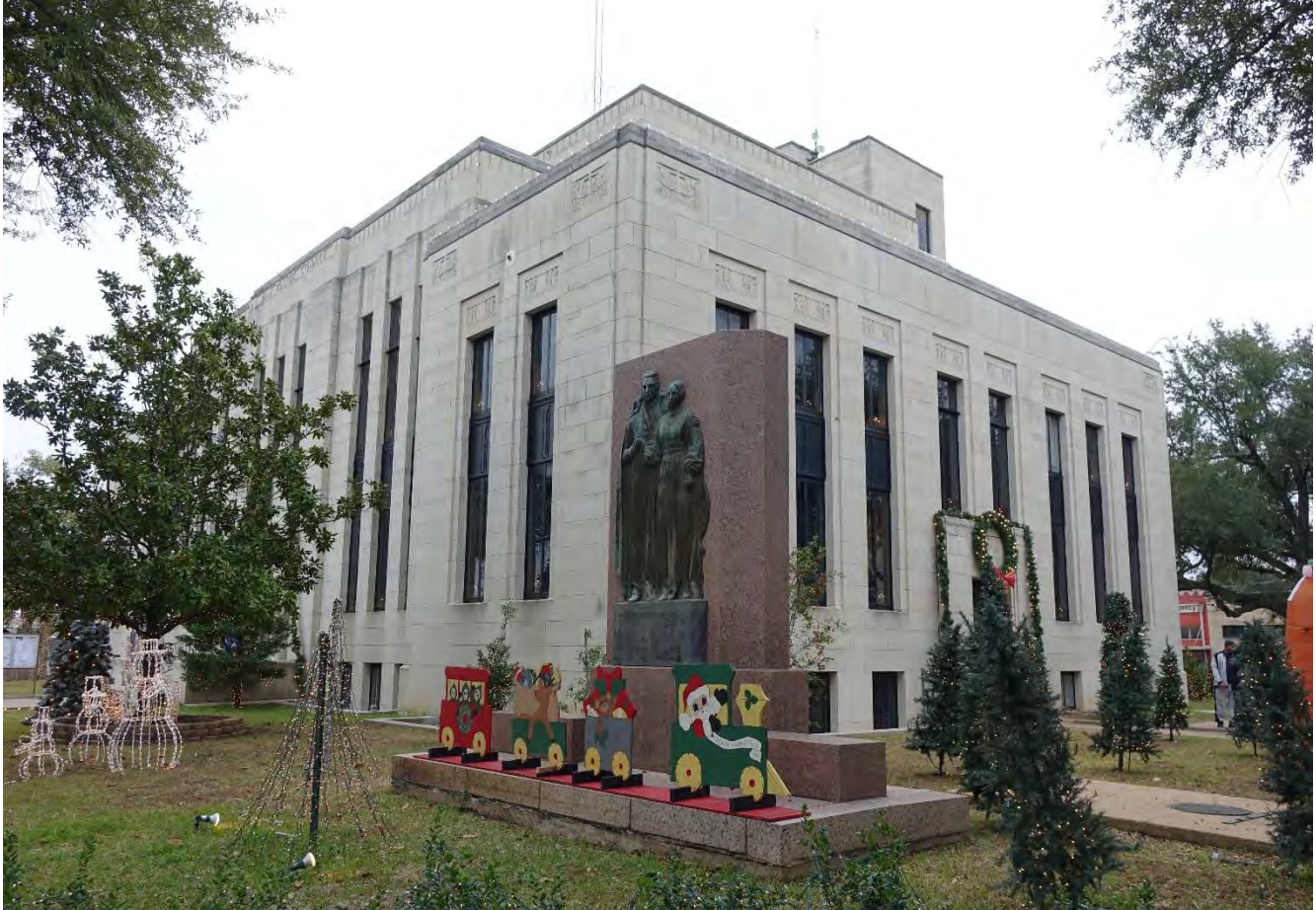
Photo 10: North and west elevations. Camera facing southeast.
