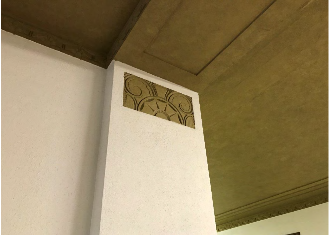
Photo 14: Coffered ceilings. Camera facing east.
