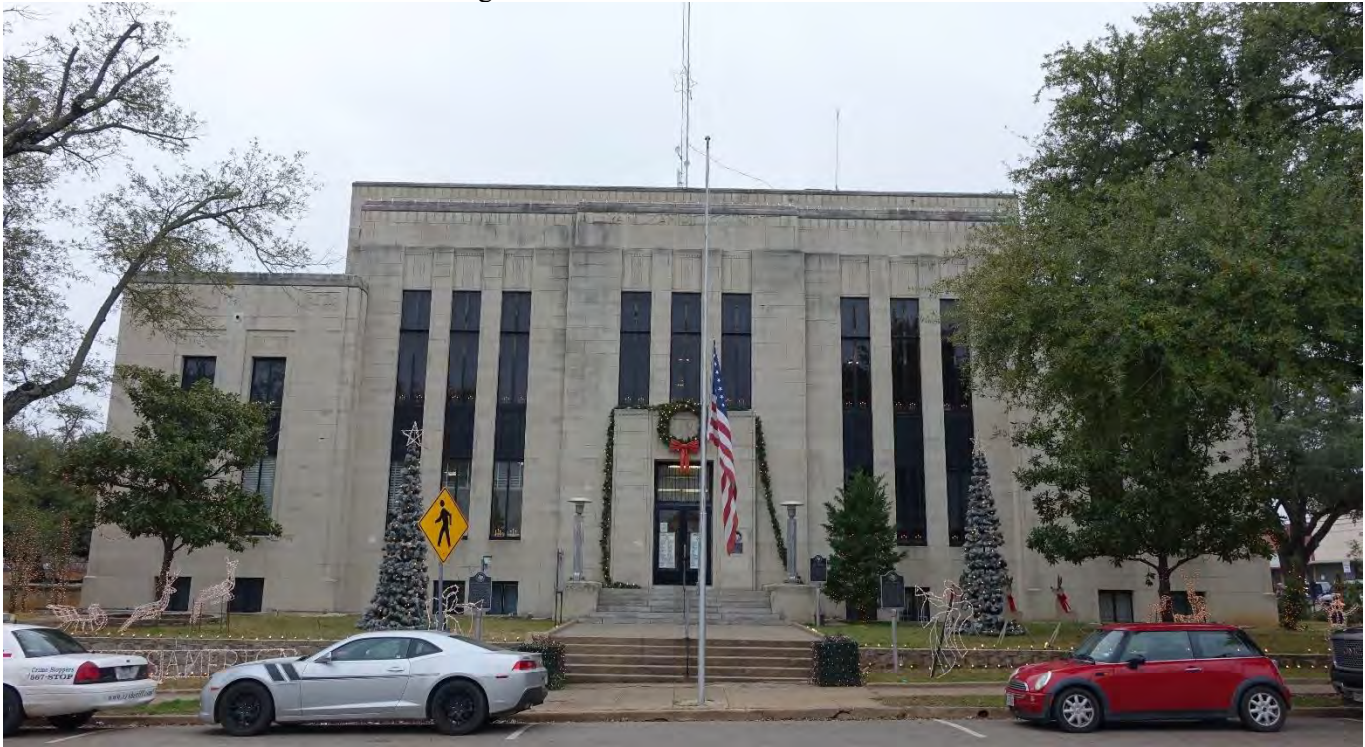
Photo 1: North elevation. Camera facing south.
