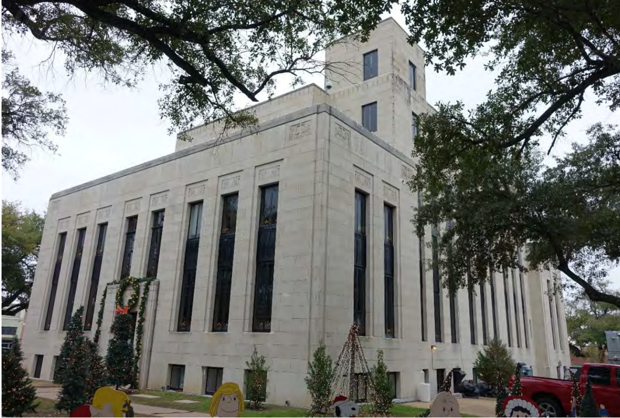
Photo 8: South and west elevations. Camera facing northeast.
