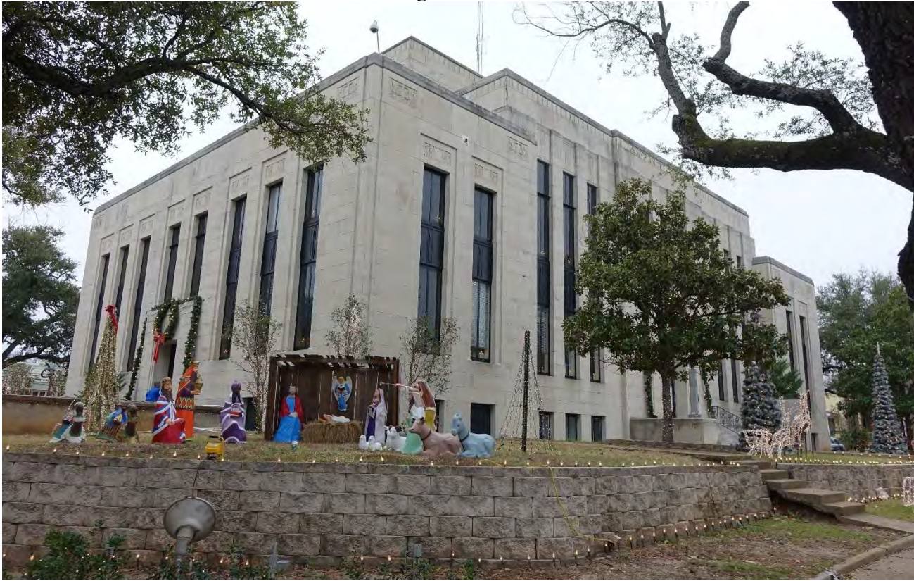
Photo 5: North and east elevations. Camera facing southwest.
