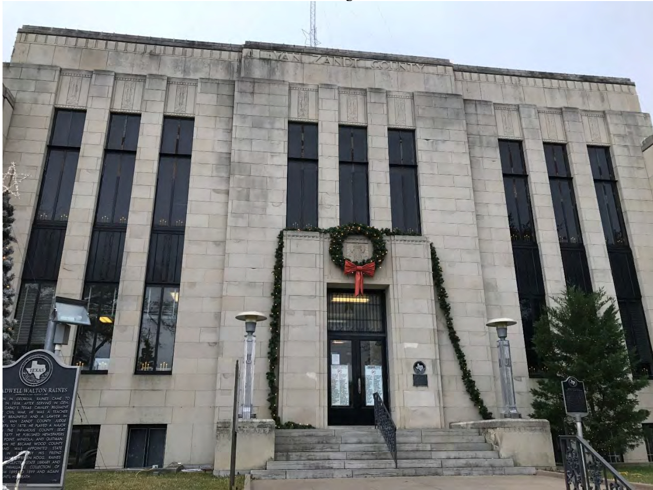
Photo 2: Main entrance on north elevation. Camera facing south.
