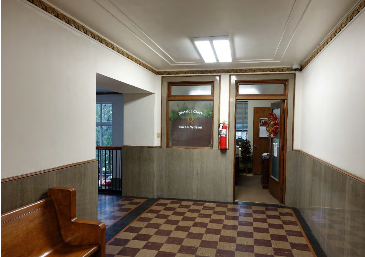
Photo 18: Third floor corridor. Camera facing east.
