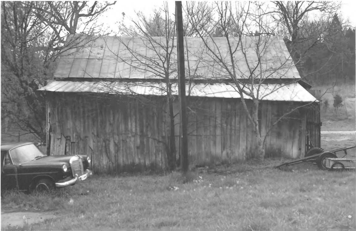
Griffitts, William H., House Loudon County Tennessee
