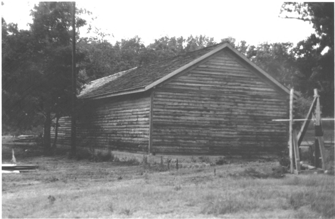
Griffitts, William H., House Loudon County Tennessee
