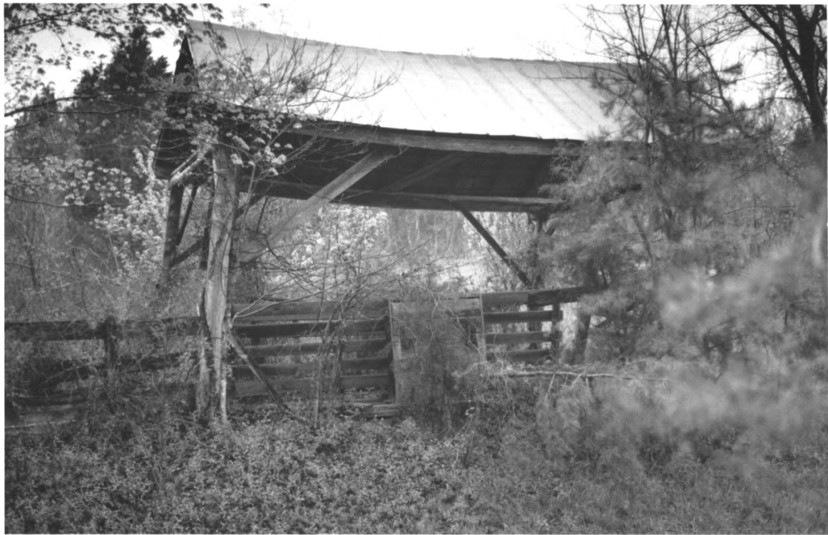
Griffitts, William H., House Loudon County Tennessee
