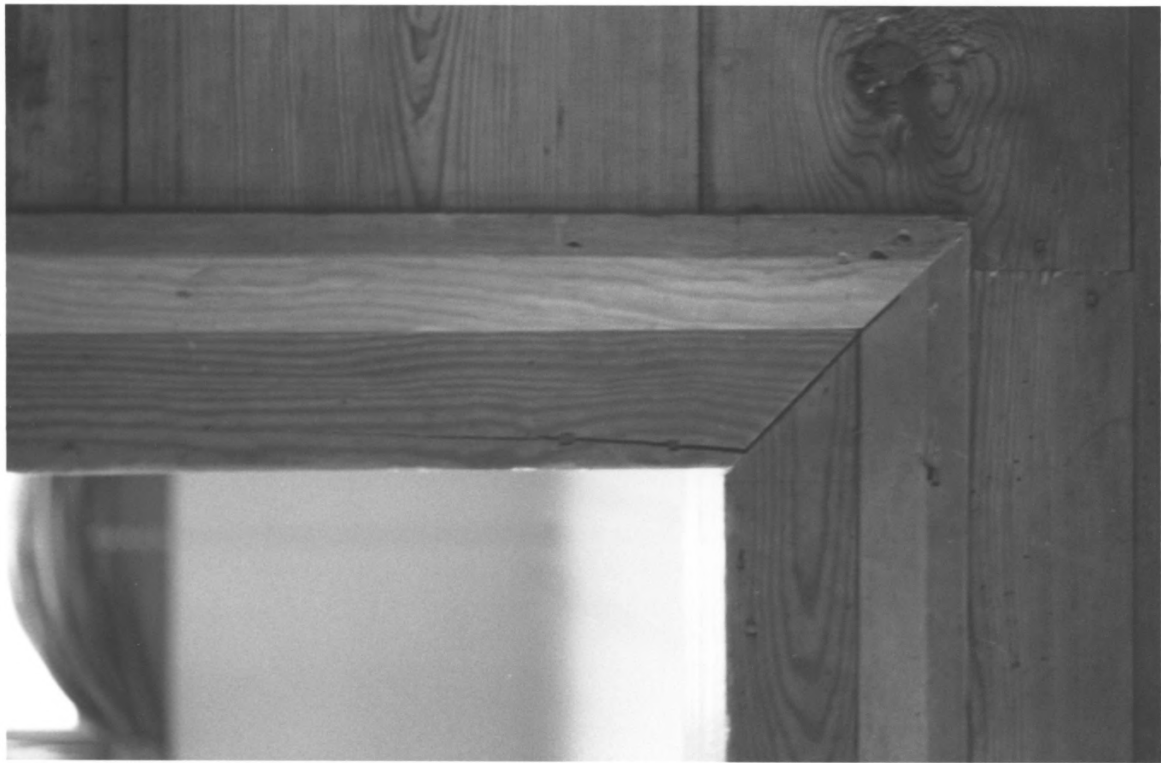
Griffitts, William H., House Loudon County Tennessee
