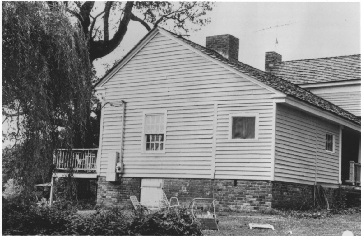
Griffitts, William H., House Loudon County Tennessee
