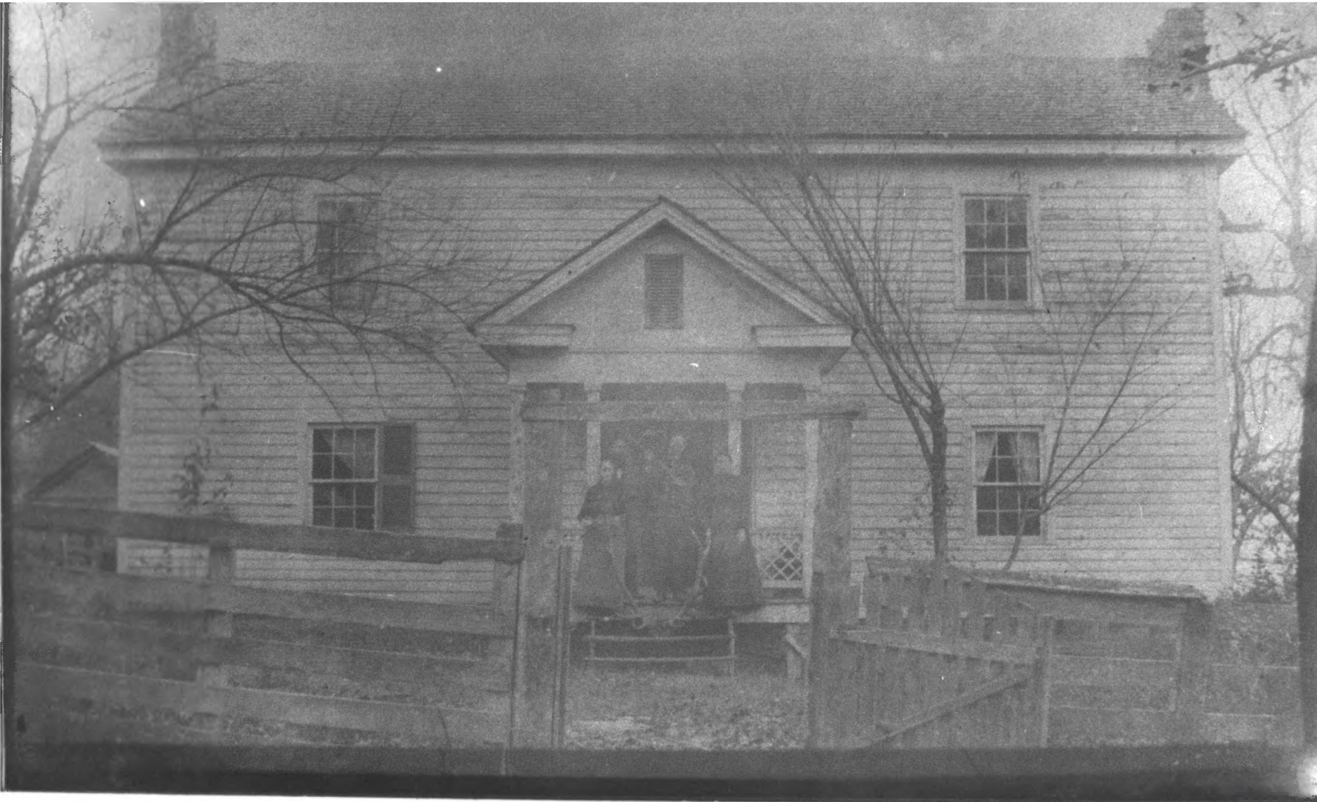
Griffitts William H., House Loudon County Tennessee
