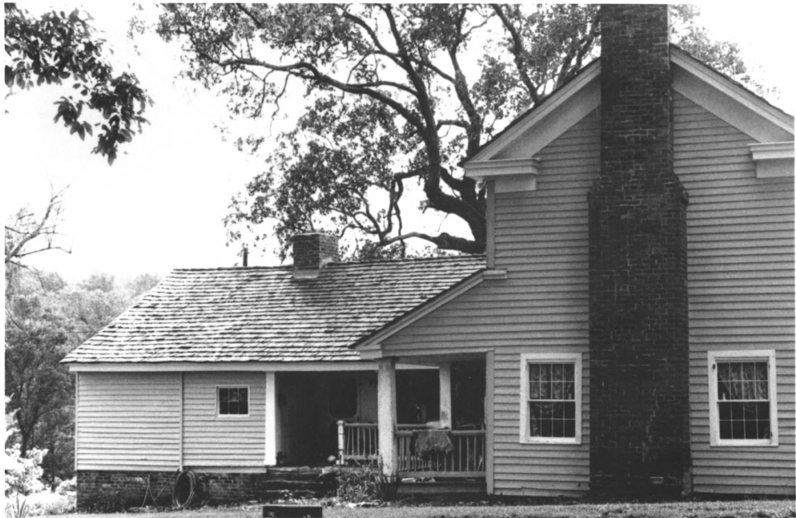
Griffitts, William H., House Loudon County Tennessee
