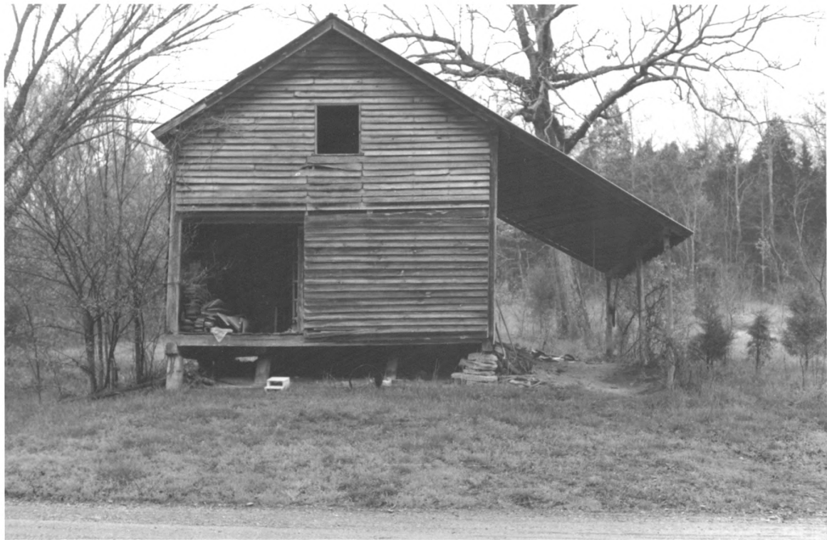
Griffitts, William H., House Loudon County, Tennessee
