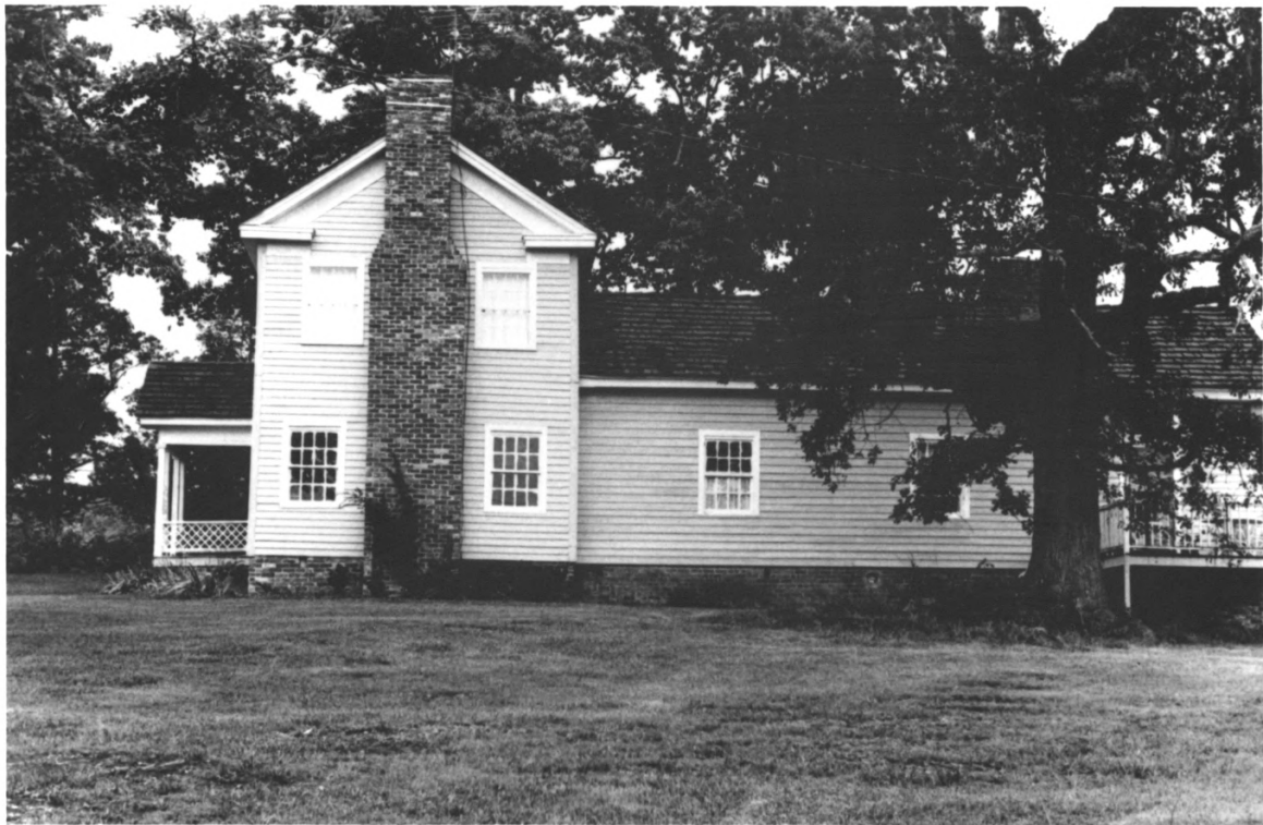
Griffitts William H., House Loudon County Tennessee
