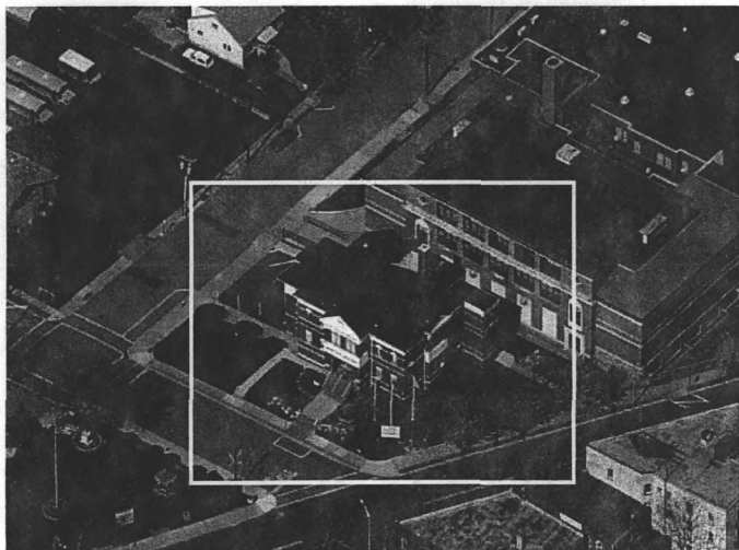
Bird's eye view of East Rutherford Municipal Building, view looking west, 2005. Microsoft Virtual Earth Web site: http://local.live.com .
