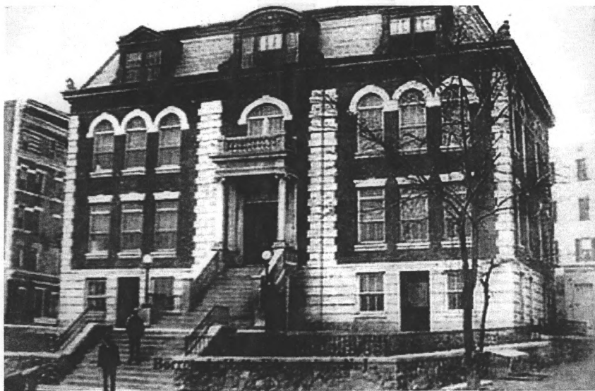
Edgewater Borough Hall, c. 1905. Photo taken soon after official opening as the horizontal tie supports have not yet been installed throughout the building. From Edgewater's Web site: www.edgewateronline.com/local.html
