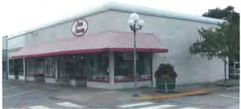
Figure 76: Building looking northwest (Jacobsen, 2017)
