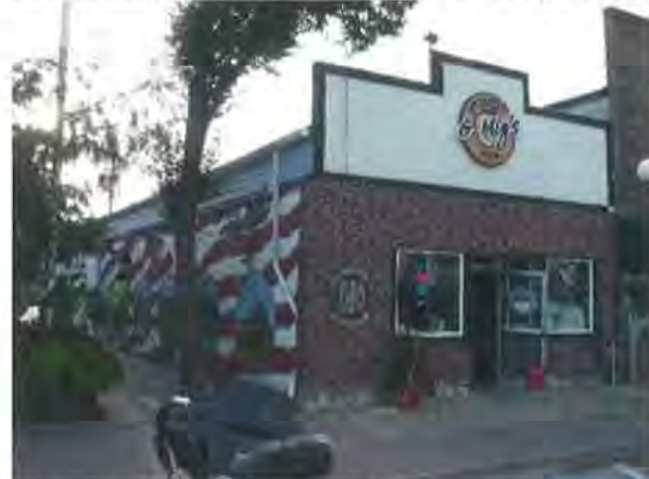
Figure 26: Building looking northwest (Jacobsen, 2017)
