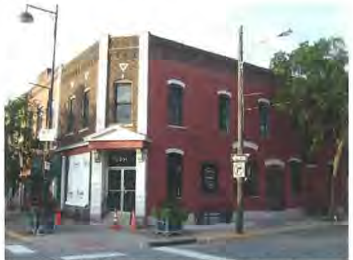
Figure 42: Building looking northeast (Jacobsen, 2017)
