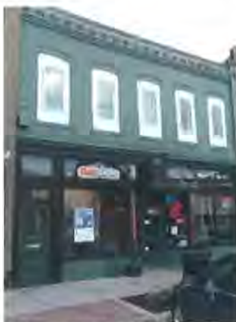
Figure 22: Building looking northwest (Jacobsen, 2017)
