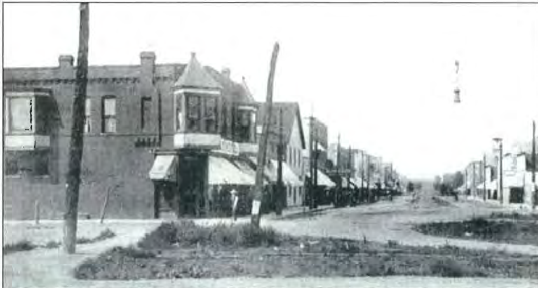
Figure 98: Lower Fifth Street looking northwest from Railroad Avenue, ca. 1914 (Jordan House Library and Archives)
