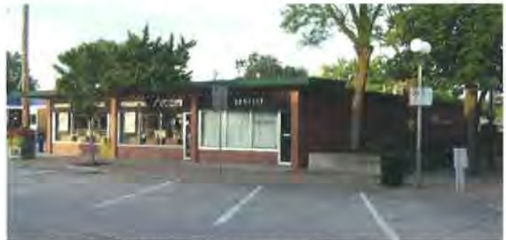
Figure 70: Building looking northeast (Jacobsen, 2017)
