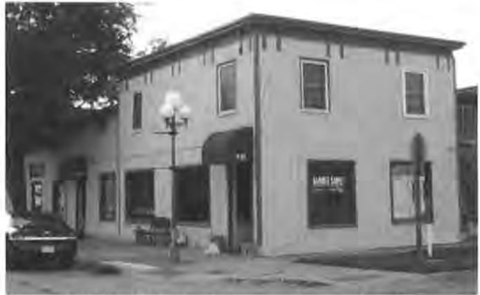
Figure 80: Building looking northwest (Jacobsen, 2017)
