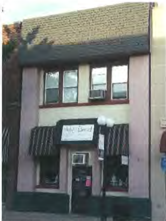
Figure 58: Building looking northeast (Jacobsen, 2017)
