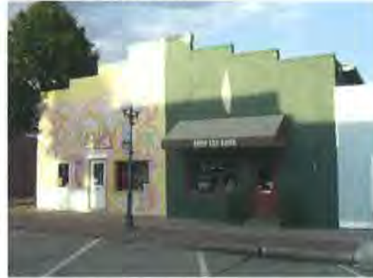
Figure 25: Building looking northeast plus the alleyway of 126 Fifth Street (Jacobsen, 2017)
