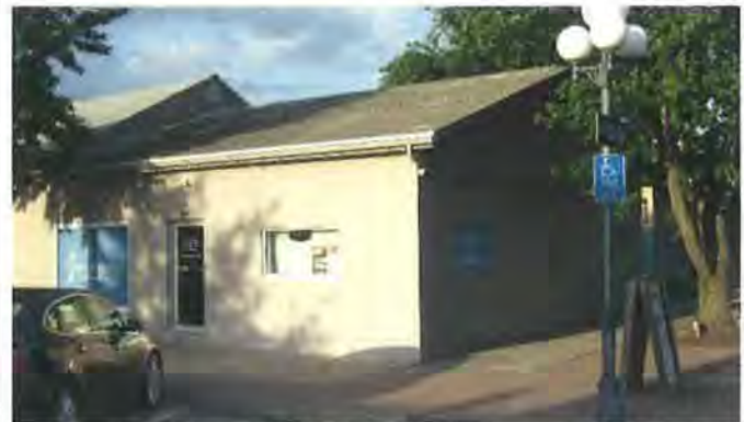
Figure 14: South part of the building looking northeast (Jacobsen, 2017)
