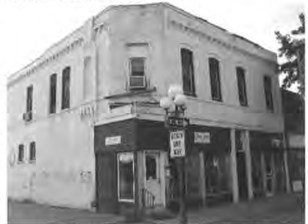
Figure 8: Building looking northwest (Jacobsen, 2017)
