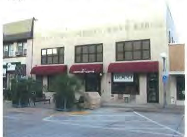
Figure 57: Building looking northeast (Jacobsen, 2017)
