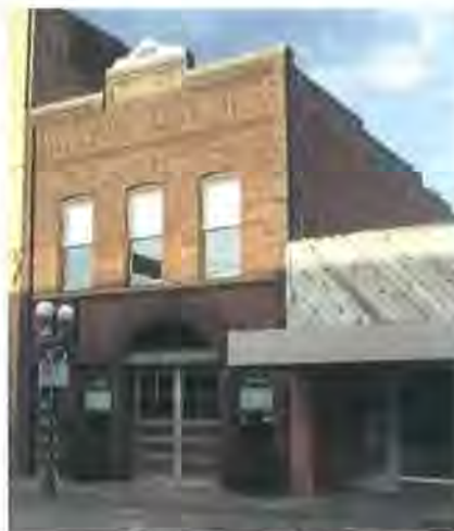
Figure 33: Building looking northeast (Jacobsen, 2017)
