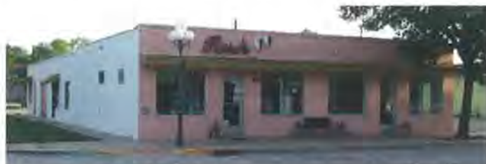
Figure 79: Building looking southwest (Jacobsen, 2017)
