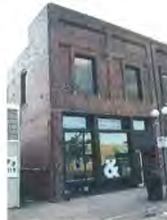
Figure 15: Building looking northwest (Jacobsen, 2017)
