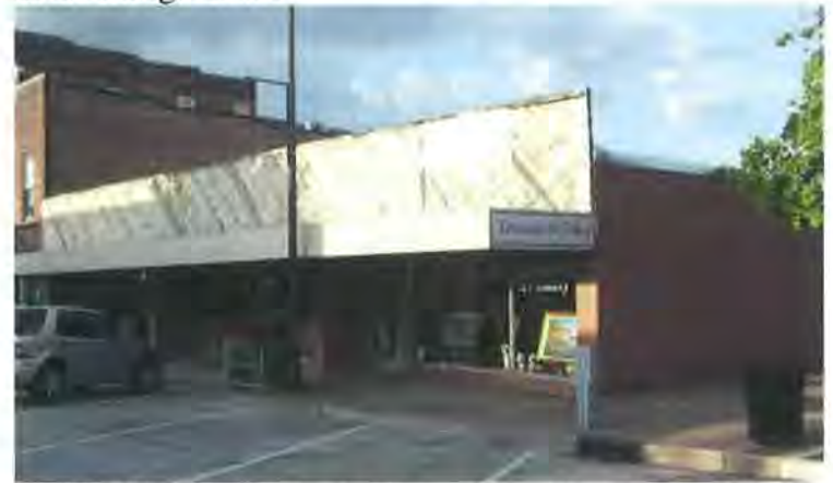
Figure 28: Building looking northeast (Jacobsen, 2017)
