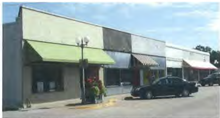
Figure 77: Building looking northeast (Jacobsen, 2017)
