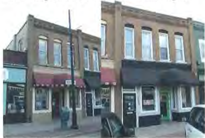
Figures 20-21: North part of the building looking northwest (Jacobsen, 2017)
