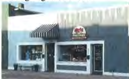
Figure 23: Building looking northeast (Jacobsen, 2017)
