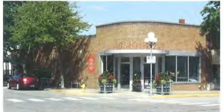
Figure 40: Building looking northwest (Jacobsen, 2017)
