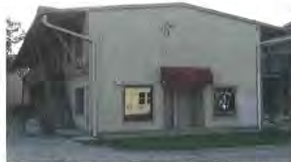
Figure 5: Building looking northwest (Jacobsen, 2017)
