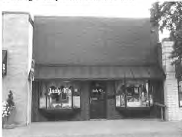
Figure 68: Building looking west (Jacobsen, 2017)
