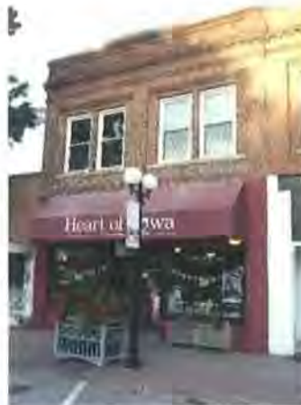
Figure 53: Building looking northeast (Jacobsen, 2017)
