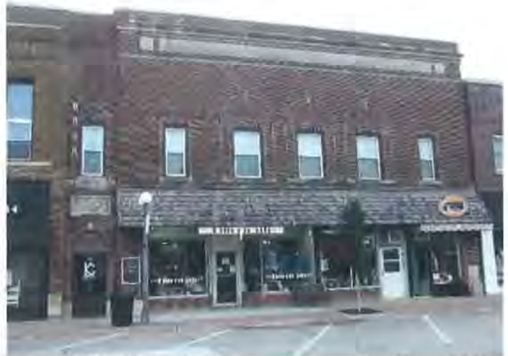
Figure 59: Building looking northwest (Jacobsen, 2017)
