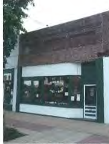
Figure 10: Building looking southwest (Jacobsen, 2017)
