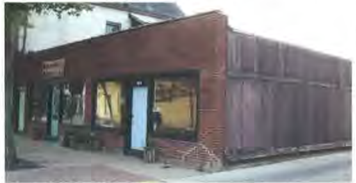
Figure 84: Building looking northwest (Jacobsen, 2017)
