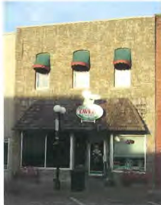
Figure 47: Building looking northeast (Jacobsen, 2017)
