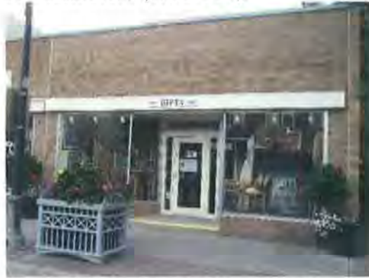
Figure 52: Building looking southwest (Jacobsen, 2017)
