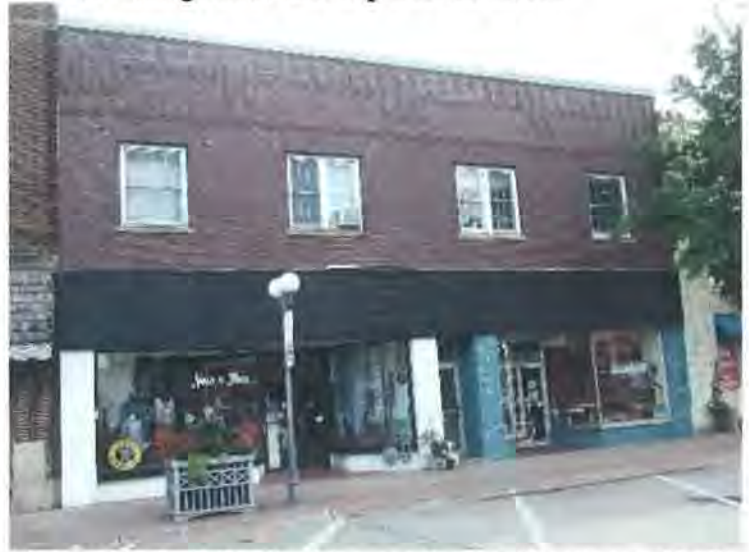
Figure 60: Building looking northwest (Jacobsen, 2017)
