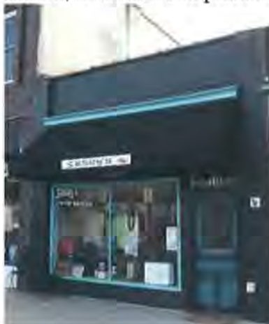
Figure 18: Building looking southwest (Jacobsen, 2017)
