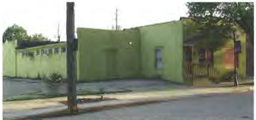
Figure 81: Building looking southwest (Jacobsen, 2017)
