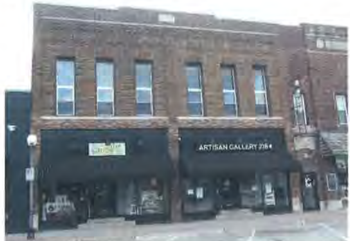
Figure 56: Building looking northwest (Jacobsen, 2017)
