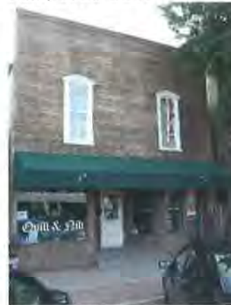
Figure 27: Building looking northwest (Jacobsen, 2017)
