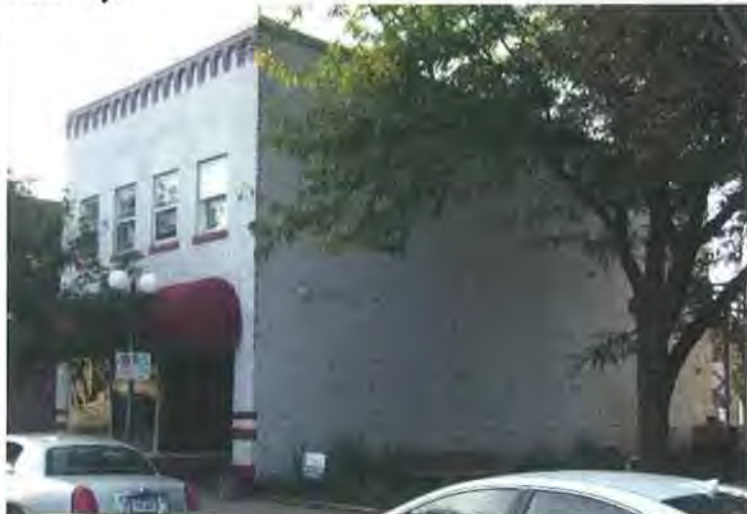
Figure 82: Building looking northwest (Jacobsen, 2017)
