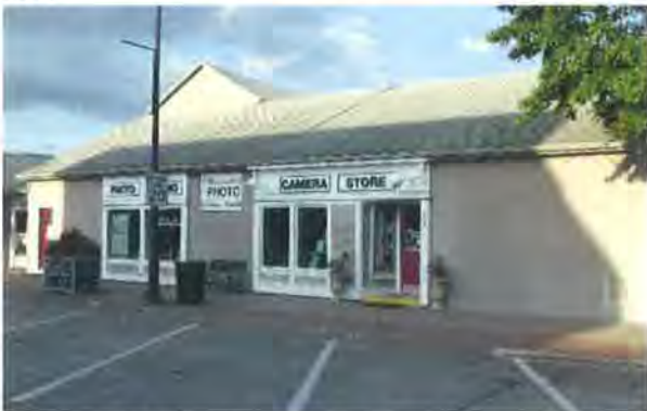
Figure 13: North part of the building looking northeast (Jacobsen, 2017)
