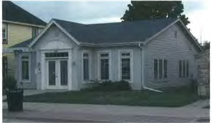
Figure 72: Building looking southwest (Jacobsen, 2017)
