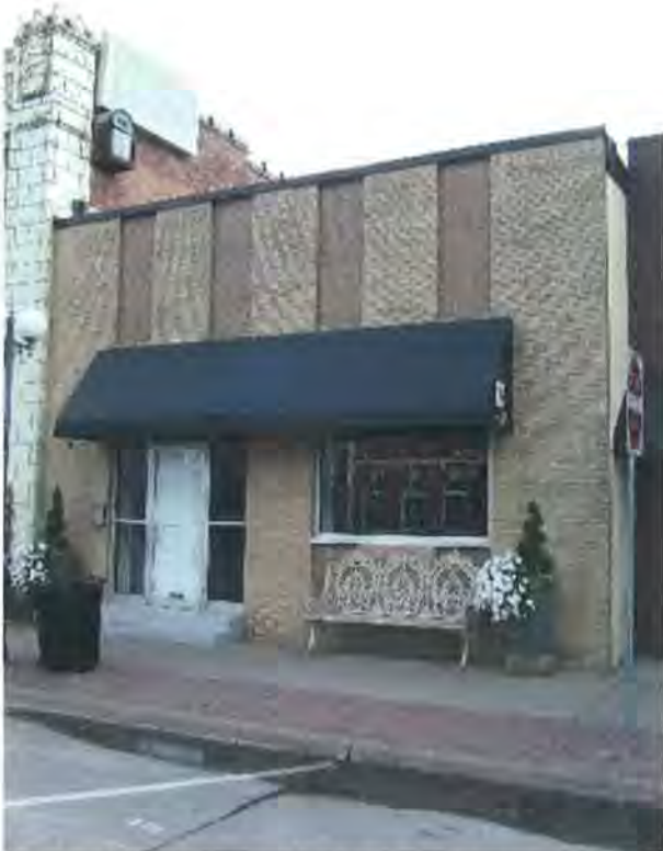
Figure 67: Building looking southwest (Jacobsen, 2017)
