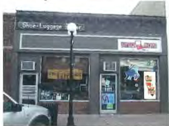
Figure 46: Building looking northwest (Jacobsen, 2017)
