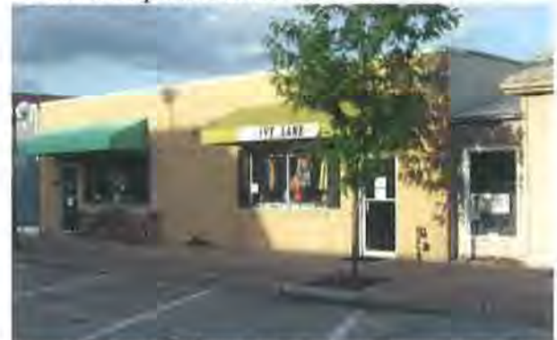
Figure 17: Building looking northeast (Jacobsen, 2017)
