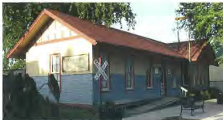
Figure 86: Building looking northeast (Jacobsen, 2017)
