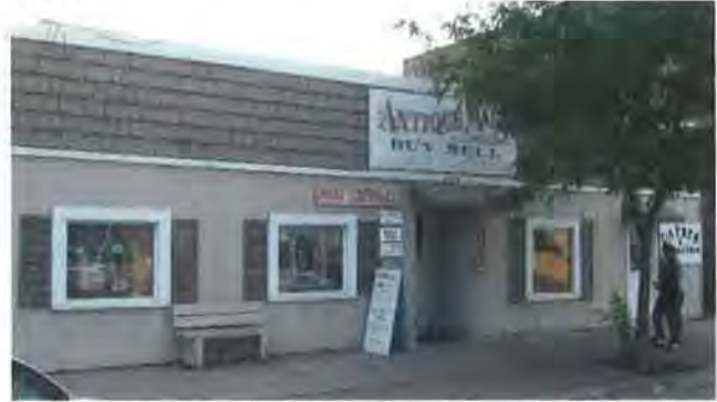
Figure 12: Building looking northwest (Jacobsen, 2017)
