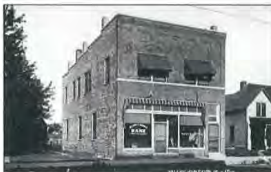
Figure 62: Newly completed 221 Fifth, looking southeast, 1900 (Jordan House Library and archives)
