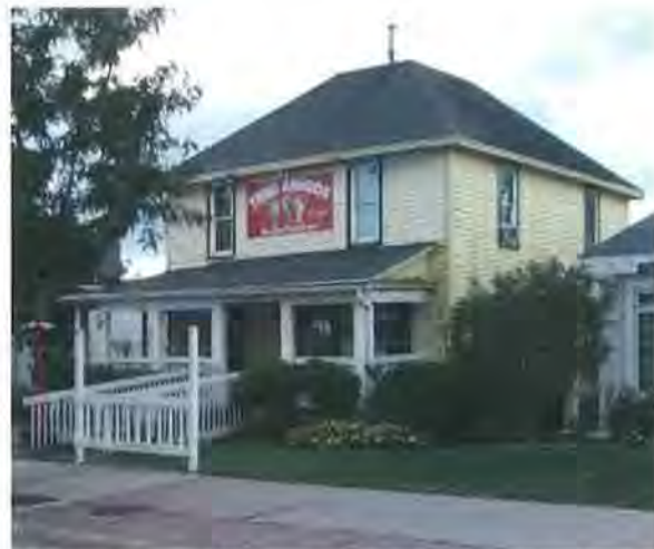
Figure 71: Building looking southwest (Jacobsen, 2017)
