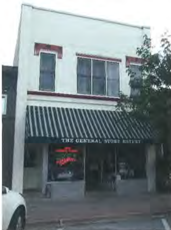
Figure 48: Building looking west (Jacobsen, 2017)
