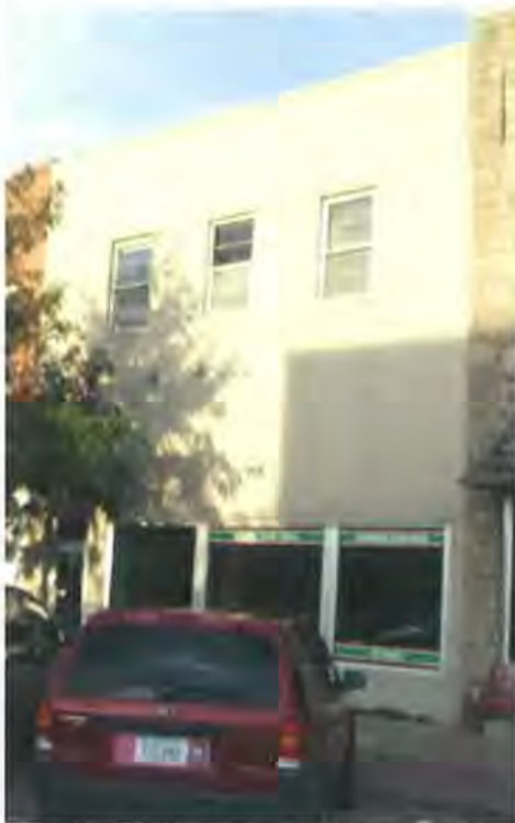
Figure 49: Building looking northeast (Jacobsen, 2017)
