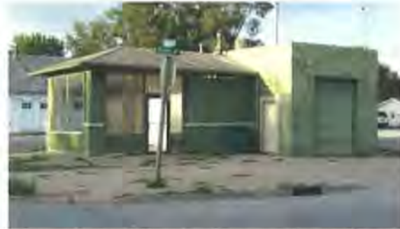
Figure 4: Building looking northeast (Jacobsen, 2017)
