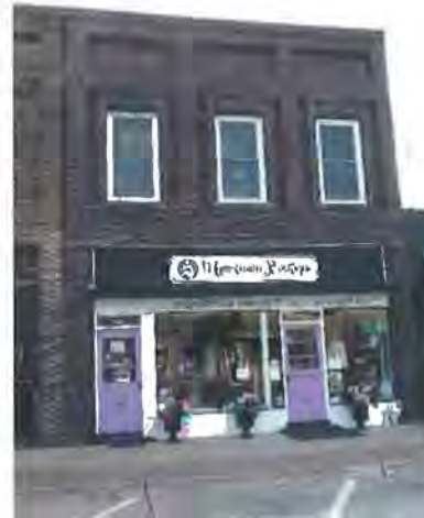
Figure 16: Building looking northwest (Jacobsen, 2017)
