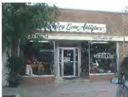
Figure 50: Building looking northwest (Jacobsen, 2017)
