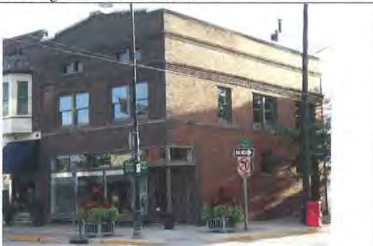
Figure 35: Building looking southwest (Jacobsen, 2017)
