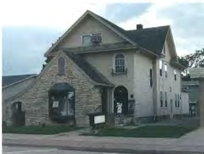
Figure 73: Building looking southwest (Jacobsen, 2017)
