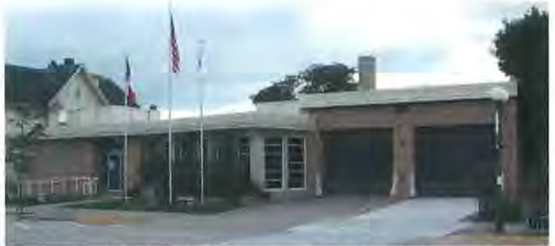
Figure 75: Building looking southwest (Jacobsen, 2017)
