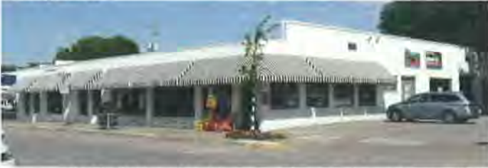
Figure 6: Building looking northwest (Jacobsen, 2017)
