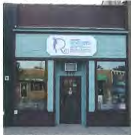
Figure 19: Building looking west (Jacobsen, 2017)
