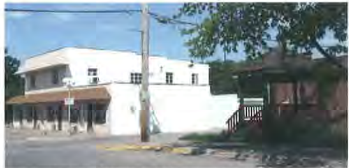
Figure 85: Building looking northwest (Jacobsen, 2017)
