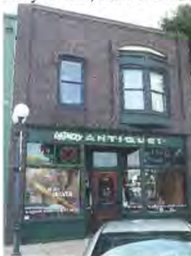
Figure 24: Building looking northwest (Jacobsen, 2017)
