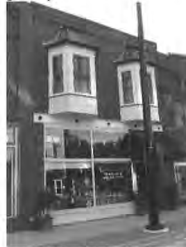
Figure 32: Building looking northwest (Jacobsen, 2017)
