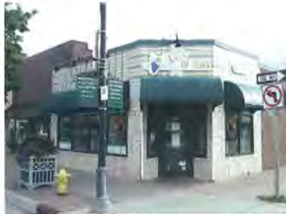
Figure 69: Building looking southwest (Jacobsen, 2017)
