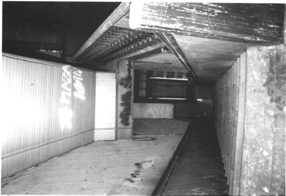
Central Black Building Hamilton Co. TN
