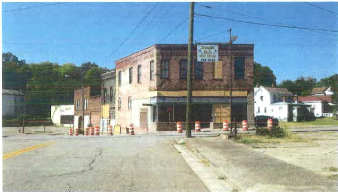
Photo 2: Five Forks commercial area after non-historic cladding removed, view SW
