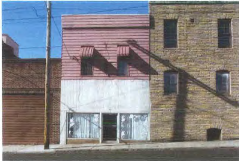
Photo 9: 400 Jefferson Street, facade (before)
