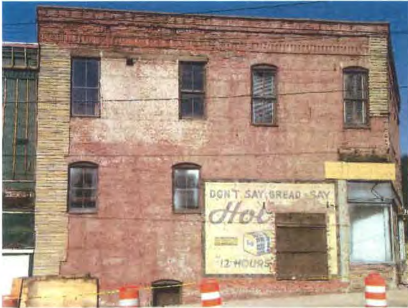
Photo 7: 254 Jefferson Avenue, East Elevation (after)
