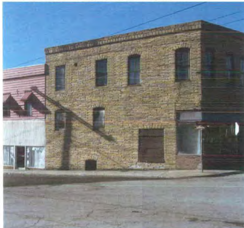
Photo 6: 254 Jefferson Avenue, East Elevation (before)
