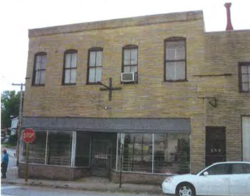
Photo 4: 254 Jefferson Avenue, North Elevation (before)
