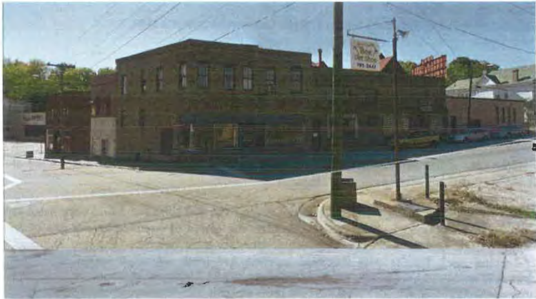
Photo 1: Five Forks commercial area before non-historic cladding removed, view SW
