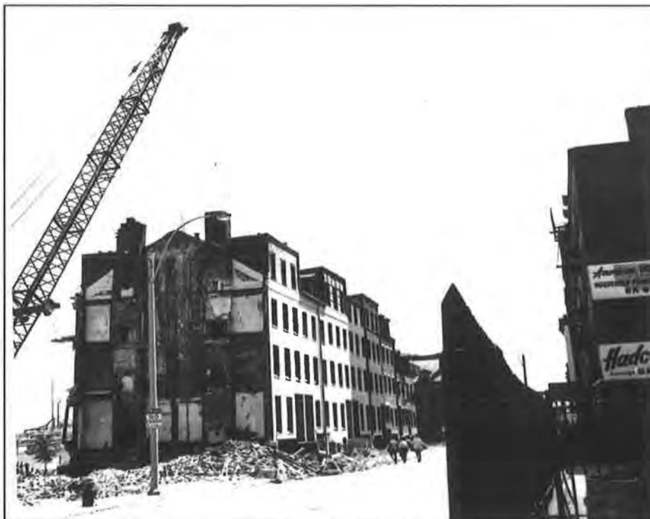
Fig.14: Demolishing houses on west side of Hudson Street for Mass Pike. From City of Boston Archives.
