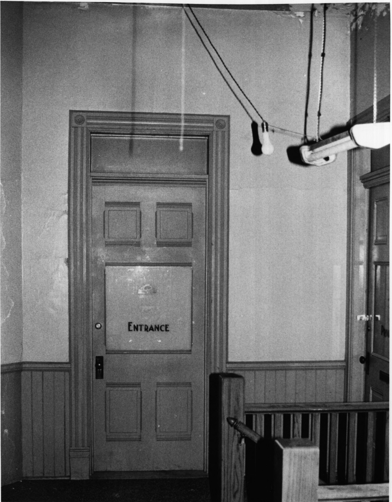
Central Block, Hughes County, South Dakota, No. 9
