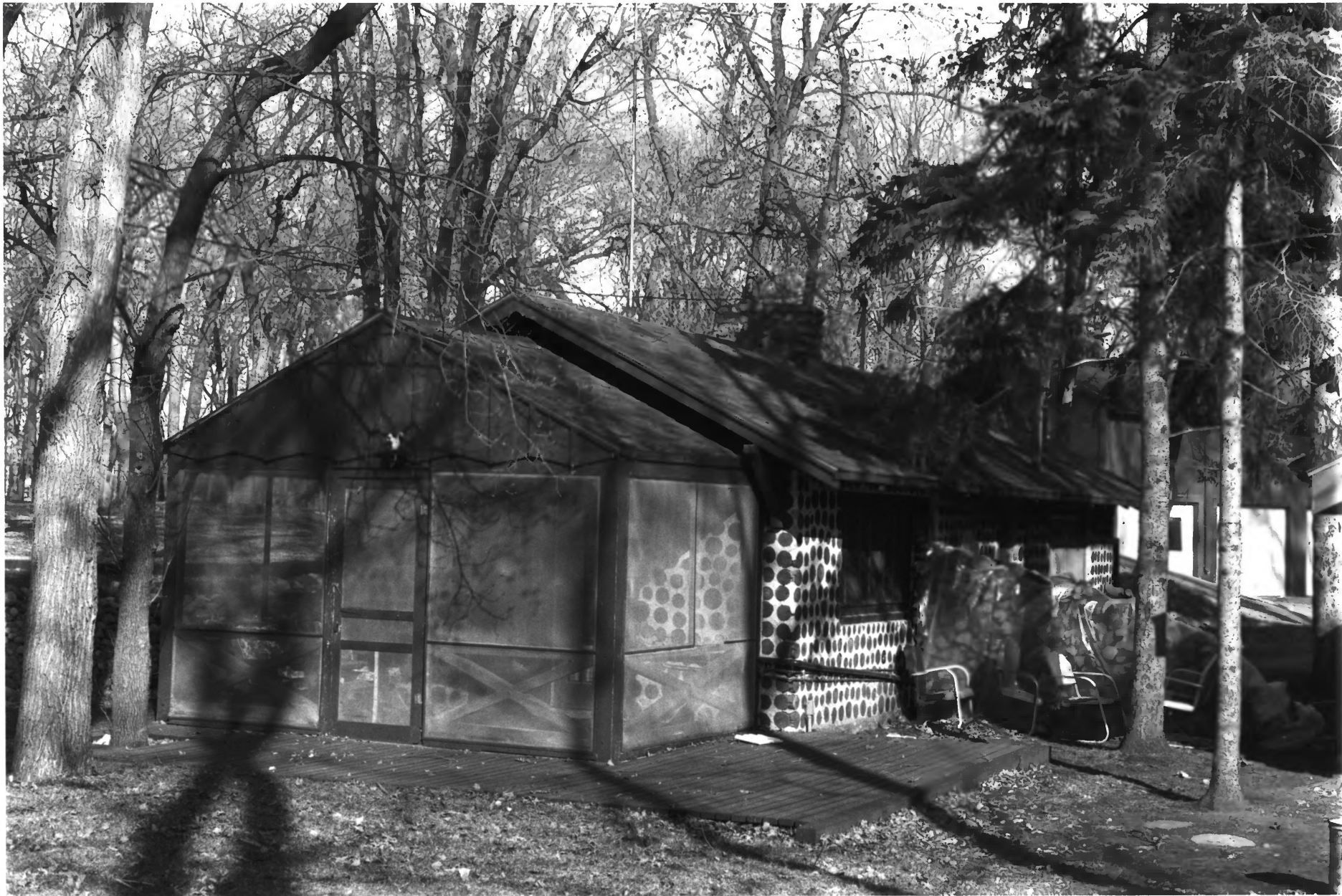
Edgewater Beach Cottages, Cottage 3 Detroit Lakes, Becker Co, MN 09229/0A
