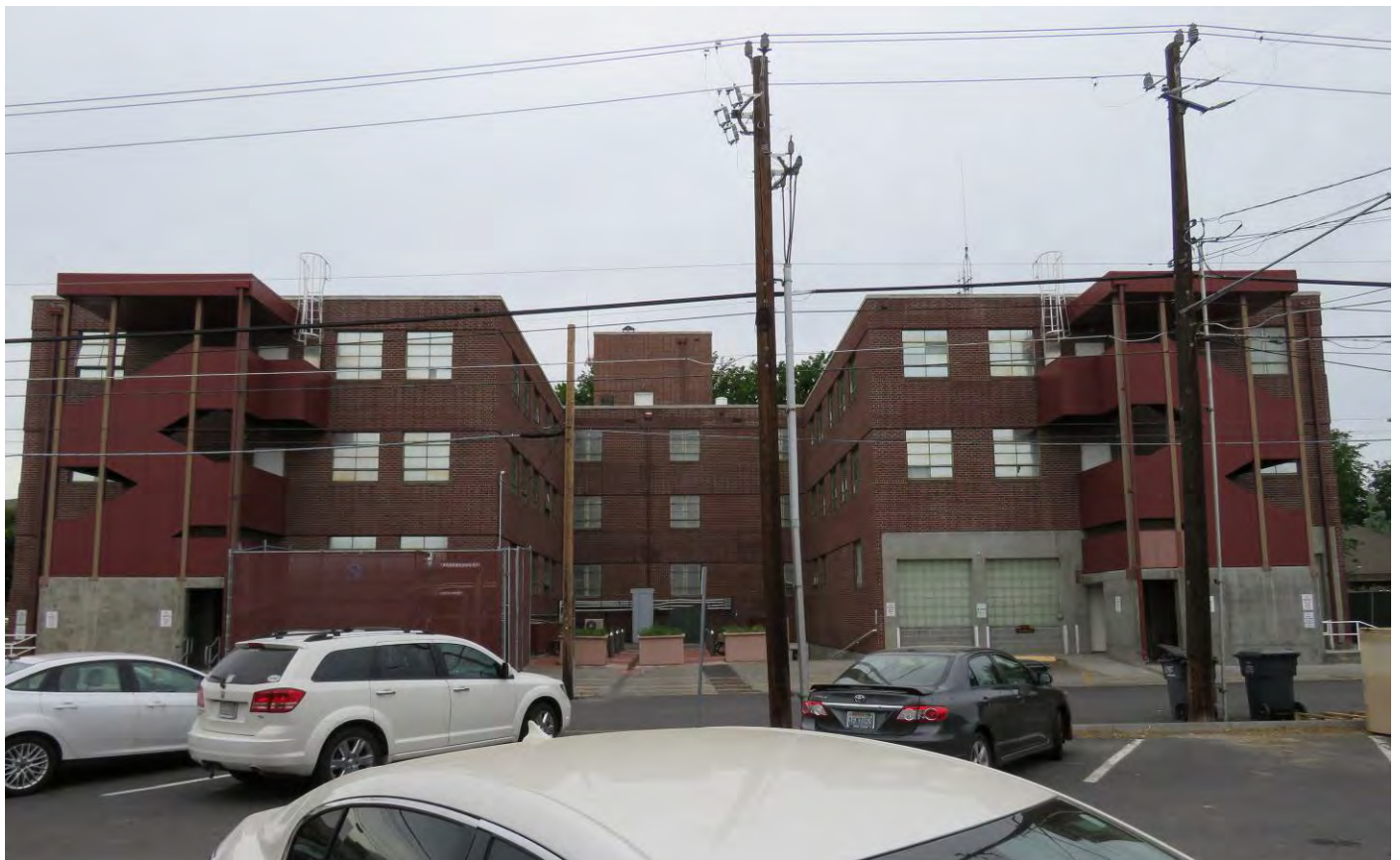
Photo No. 5 – Columbia Basin Project Irrigation Division Headquarters Office – Rear Elevation.
