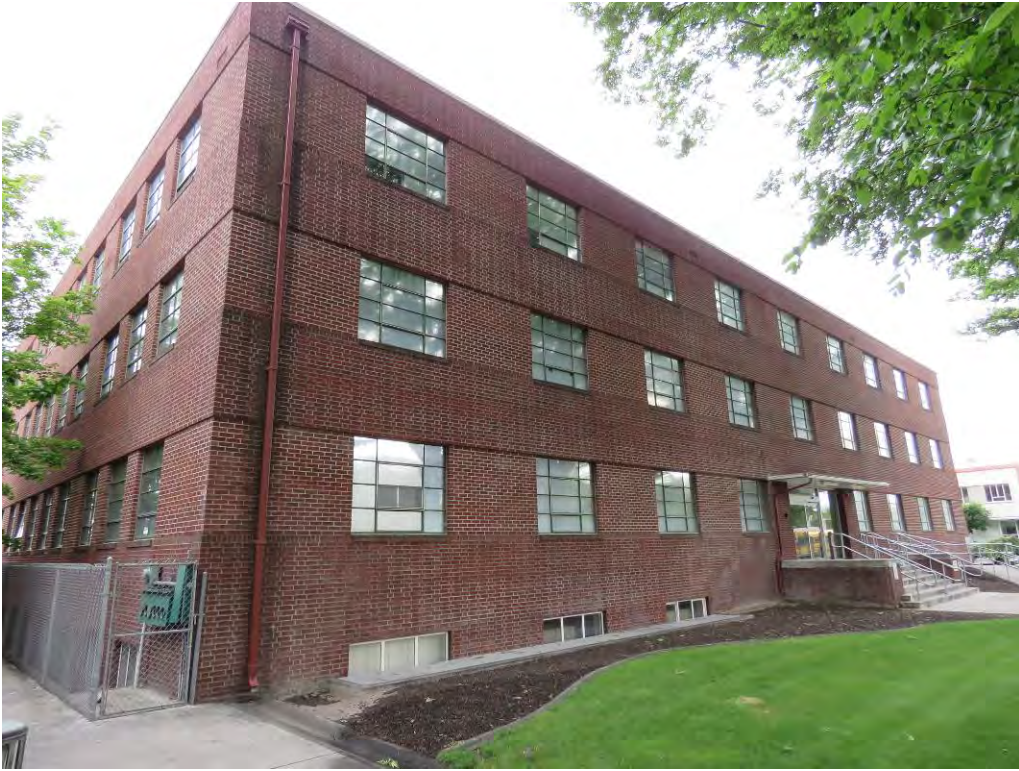
Photo No. 2 – Columbia Basin Project Irrigation Division Headquarters Office – Oblique view of North and Front Elevations.
