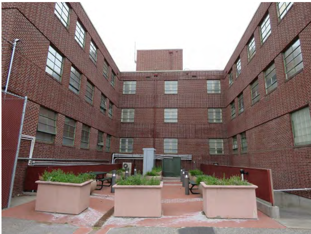
Photo No. 7 – Columbia Basin Project Irrigation Division Headquarters Office – Detail of the courtyard space within the U of the building's rear elevation.
