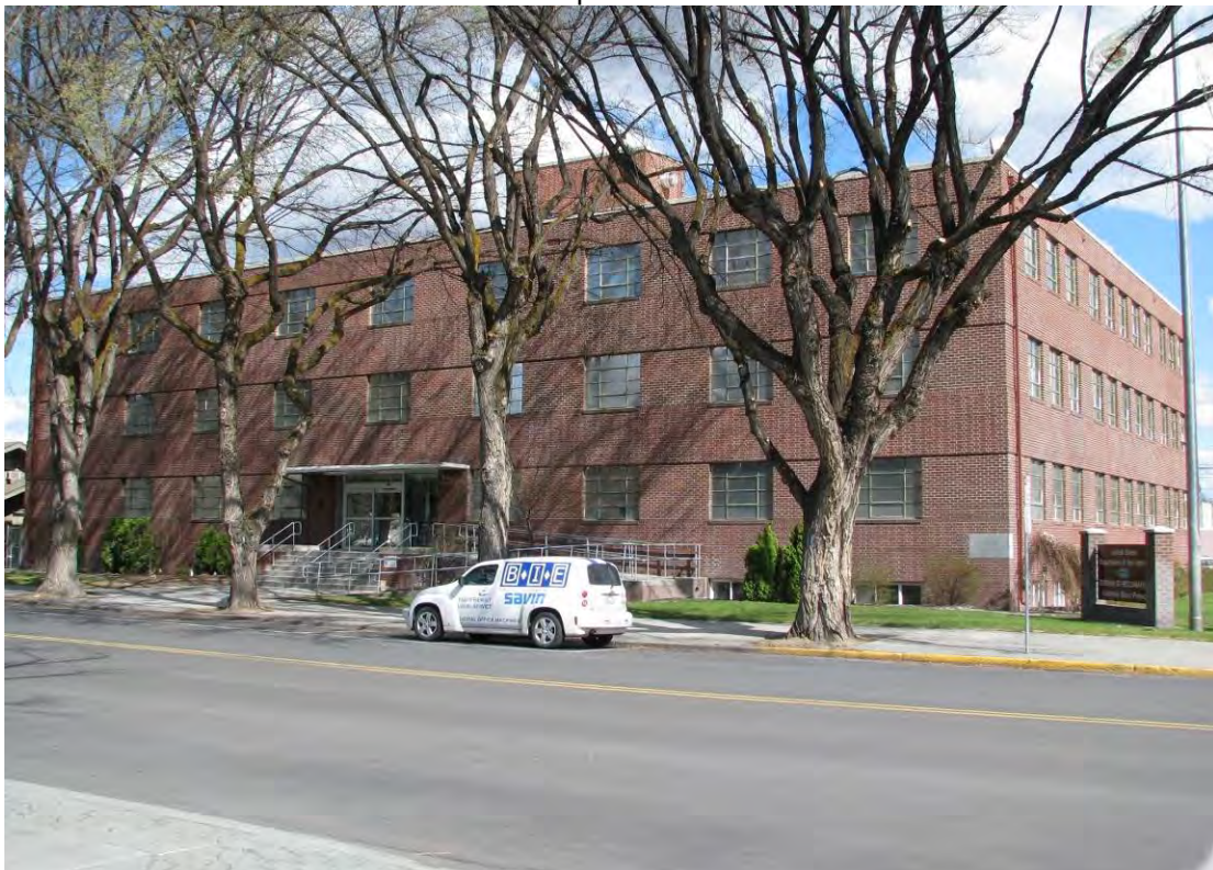
Columbia Basin Project Irrigation Division Headquarters Office – 2012 digital photograph by Kelsey J. Doncaster.
