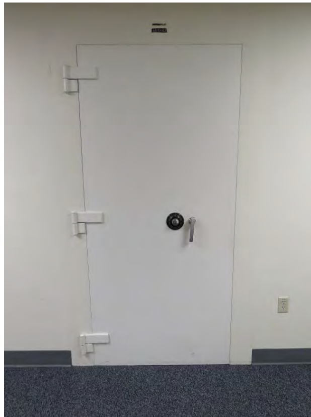
Photo No. 14 – Columbia Basin Project Irrigation Division Headquarters Office – Vault on the first-floor south side.
