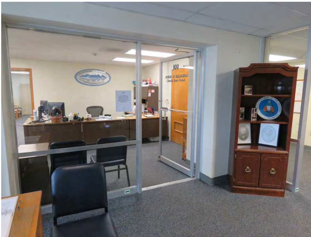
Photo No. 12 – Columbia Basin Project Irrigation Division Headquarters Office – View in First floor lobby looking north at 1960 remodel of glass and steel where a wall had been.
