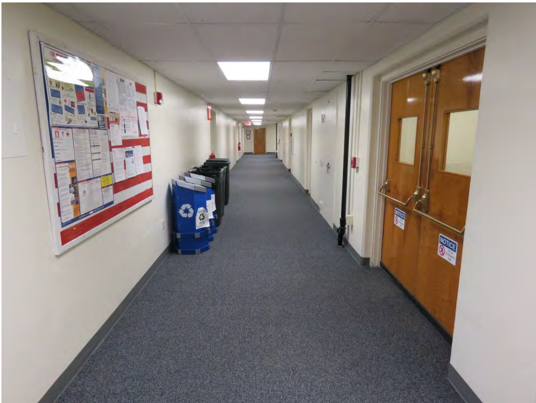
Photo No. 18 – Columbia Basin Project Irrigation Division Headquarters Office – Basement looking north.
