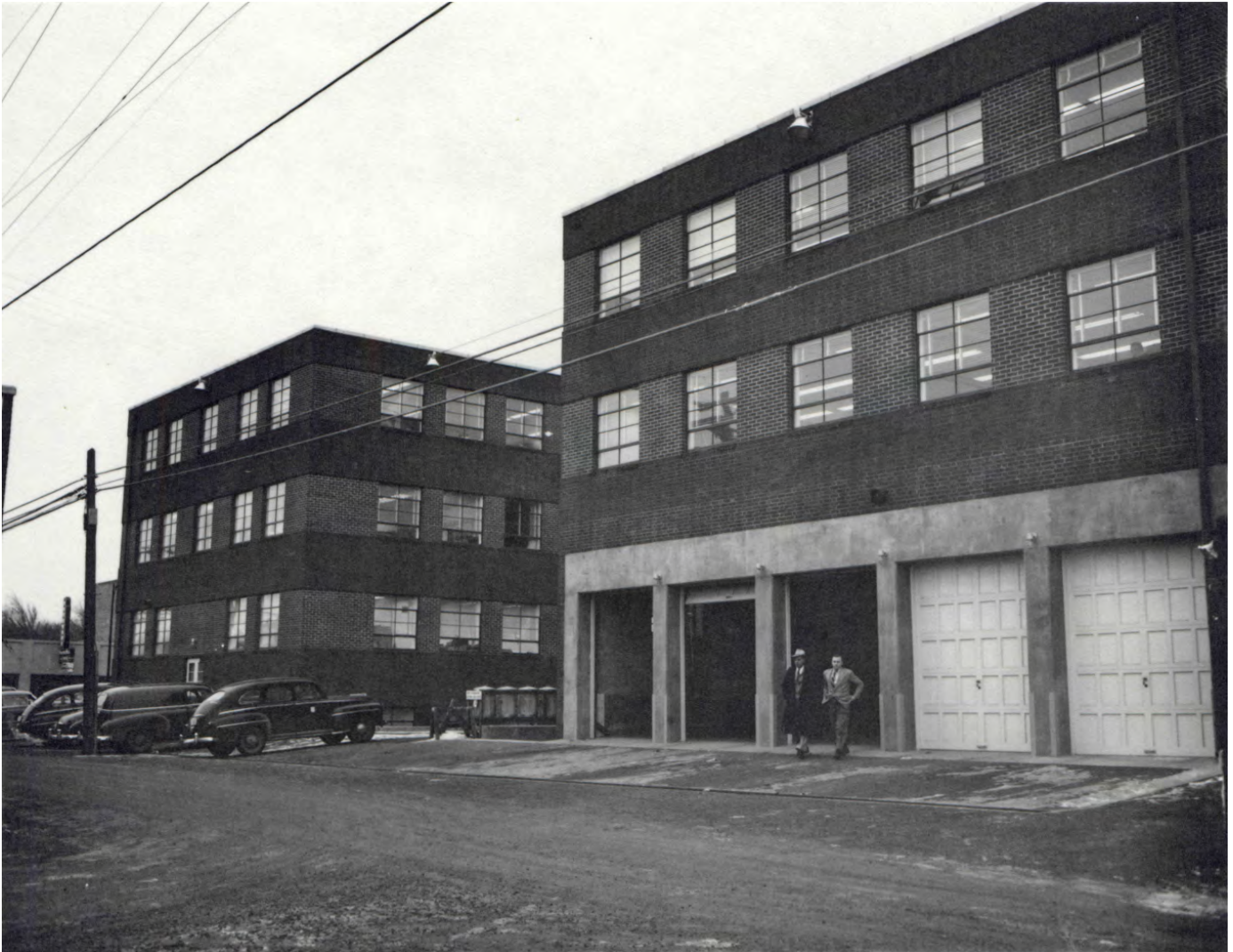
Rear view of the completed Ephrata Office Building. Note the contrast in colored mortar used in masonry. Reclamation Photograph No. 31300, December 17, 1951.
