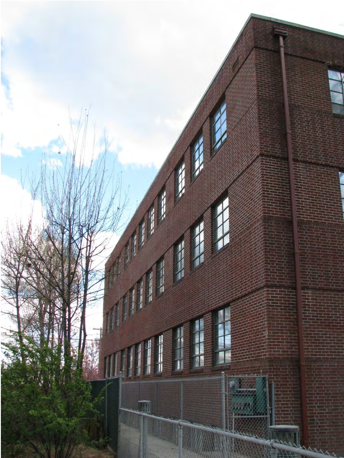
Photo No. 9 – Columbia Basin Project Irrigation Division Headquarters Office – Oblique view of North and a little of the Front Elevations. Photograph taken in 2012 by Kelsey J. Doncaster.
