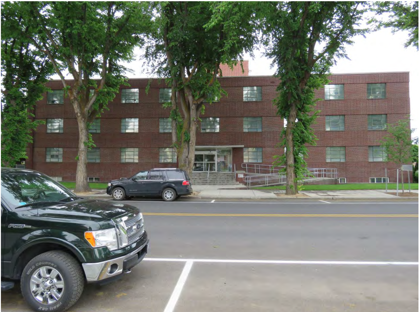
Photo No. 1 – Columbia Basin Project Irrigation Division Headquarters Office – Front Elevation.
