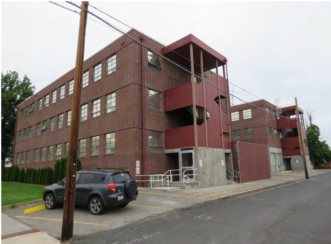
Photo No. 6 – Columbia Basin Project Irrigation Division Headquarters Office – Oblique view of South and Rear Elevations. Note non-historic emergency exit stairs on the rear elevation.
