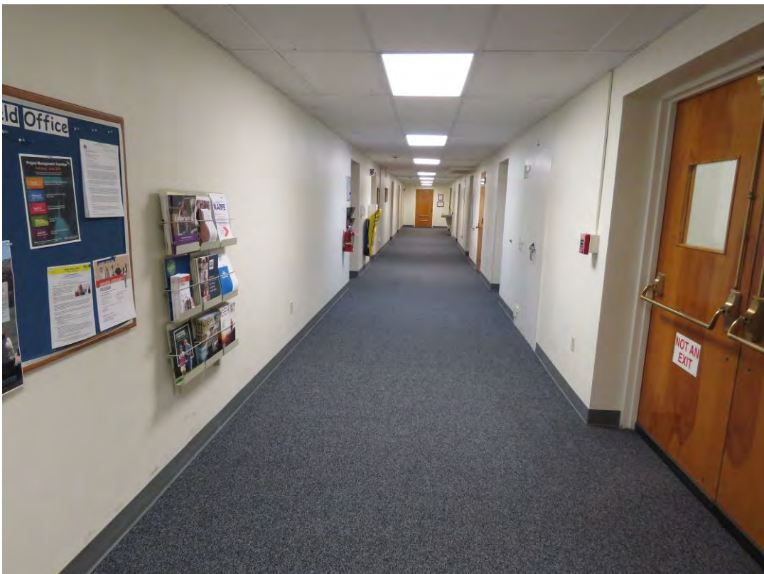
Photo No. 16 – Columbia Basin Project Irrigation Division Headquarters Office – Second Floor
