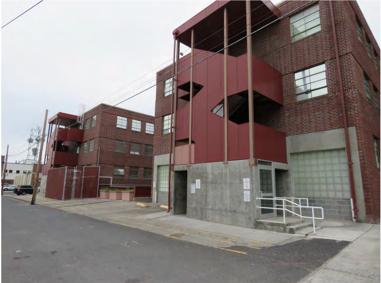
Photo No. 8 – Columbia Basin Project Irrigation Division Headquarters Office – Oblique view of North and Rear Elevations. Compare with historic Reclamation photograph from 1951.
