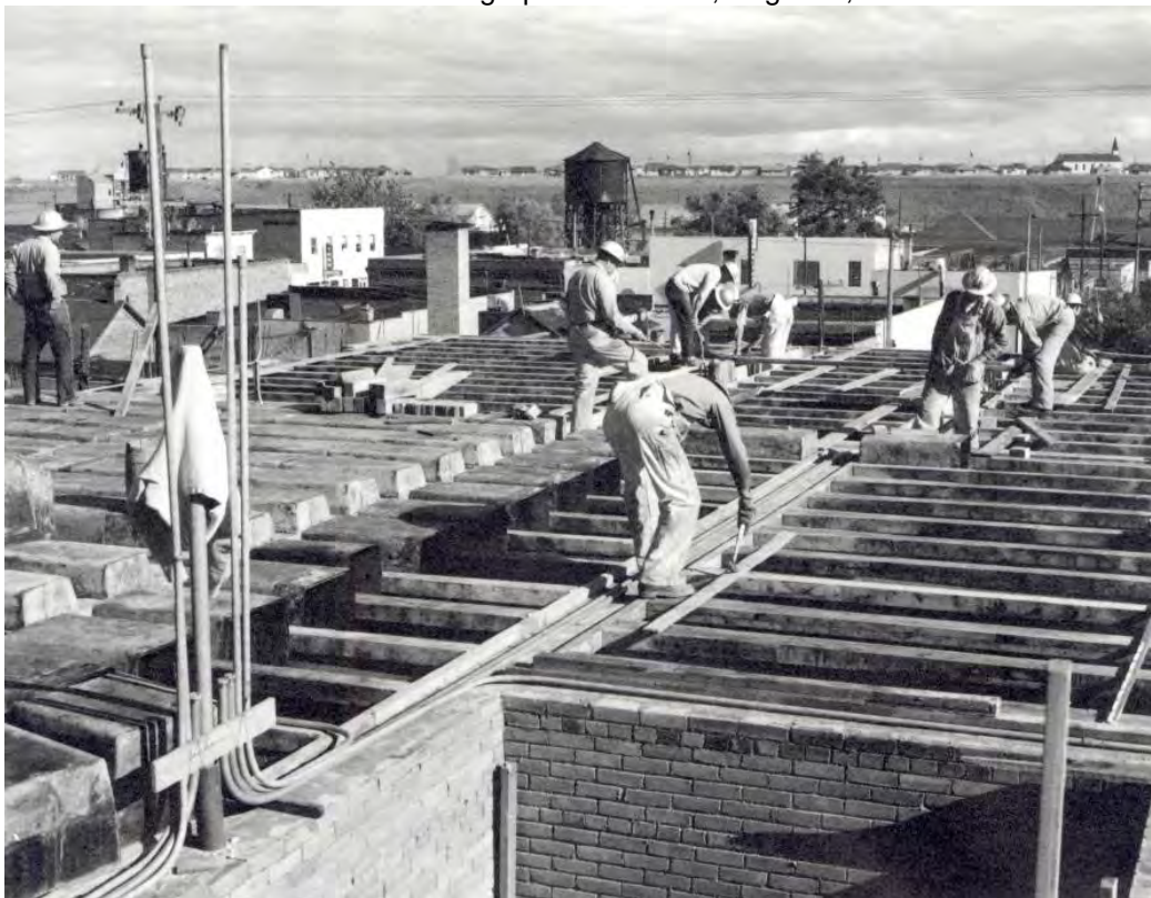
Third floor framing for pan joists. Reclamation Photograph No. 4-4488, October 10, 1950.
