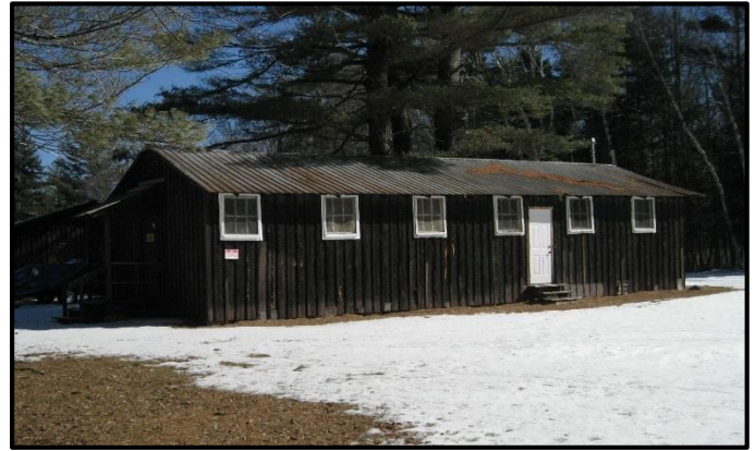
Figure 15. CCC Barracks #1 (later, 4-H Camp Speculator Cabins 9-10), 2016, looking east.
