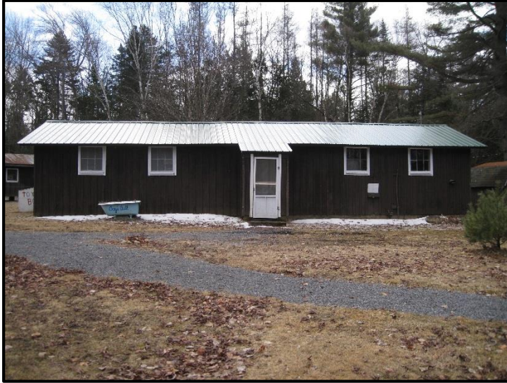
Figure 11. Lavatory (now Boys Bath House), Façade, 2016.
