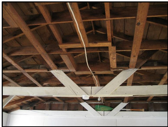
Figures 16-17. Interior, CCC Barracks #1 (4-H Camp Speculator Cabins 9-10), 2016. Note windows, open truss system, and framed vent for the stovepipe.
