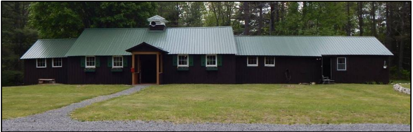
Figure 31. Recreation Hall, 2016. Photo from Jim Tavares.
