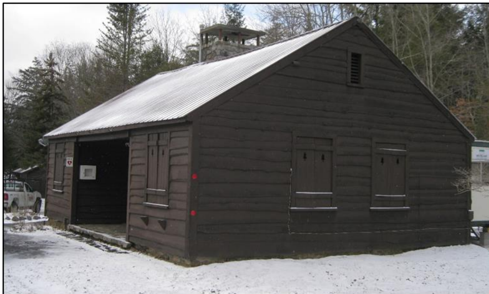
Figure 45 and 46. Superintendent's Cabin and shutter detail, Lewey Lake Campground, 2016.
