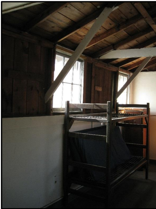
Figures 16-17. Interior, CCC Barracks #1 (4-H Camp Speculator Cabins 9-10), 2016. Note windows, open truss system, and framed vent for the stovepipe.
