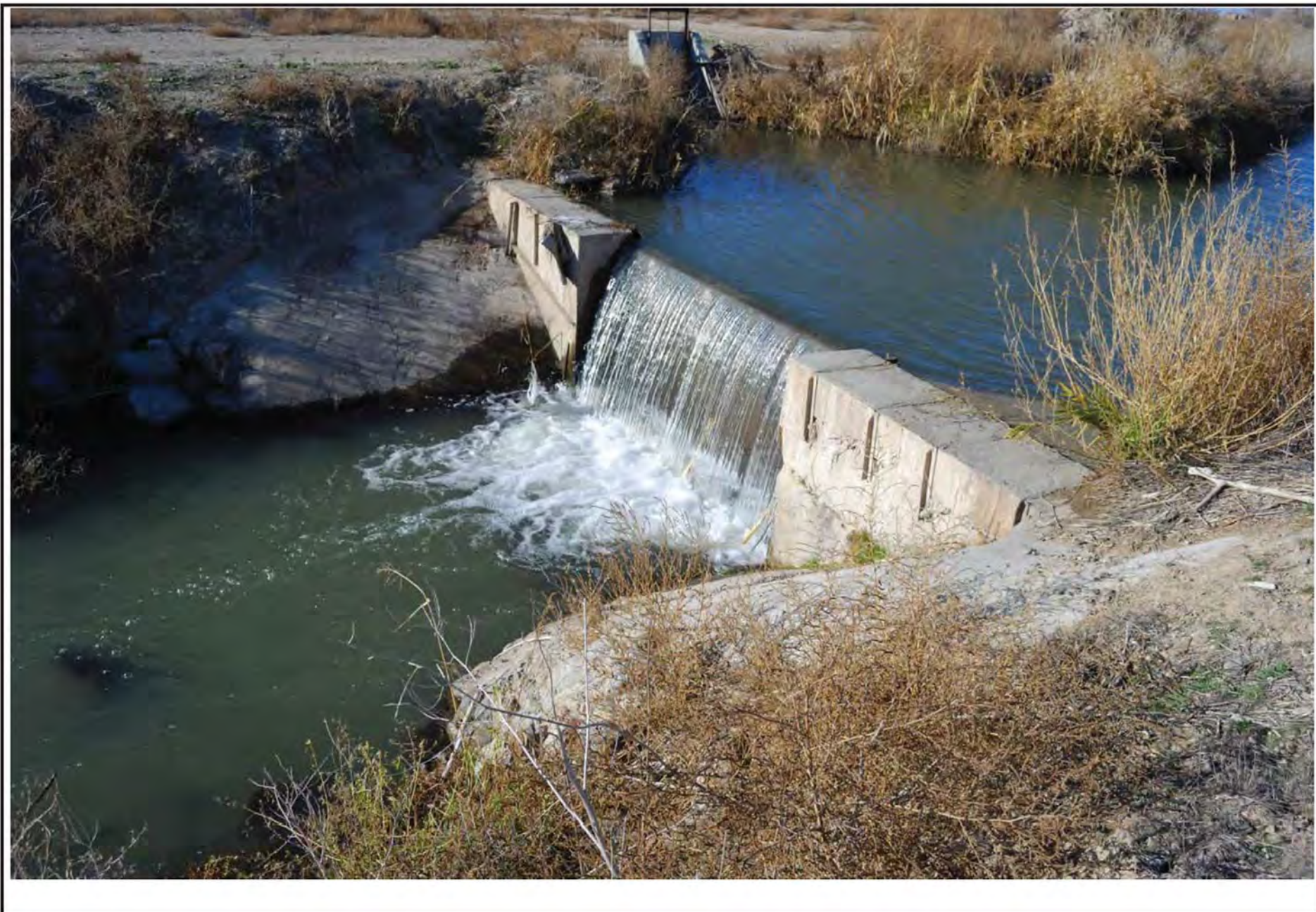
Figure 5 Check Structure, Vale Project, Malheur County
