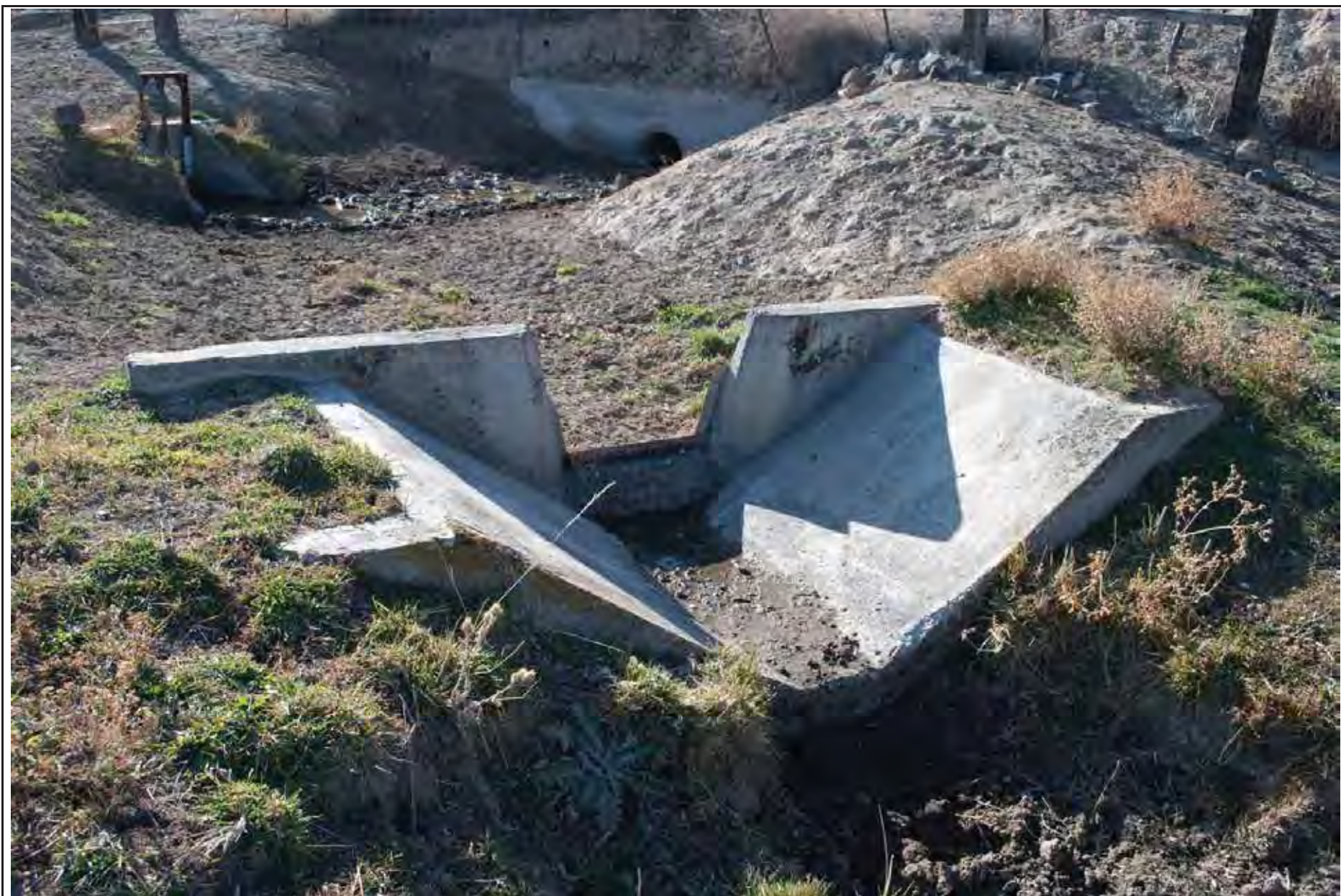
Figure 24 Cipoletti Weir, Vale Project, Malheur County
