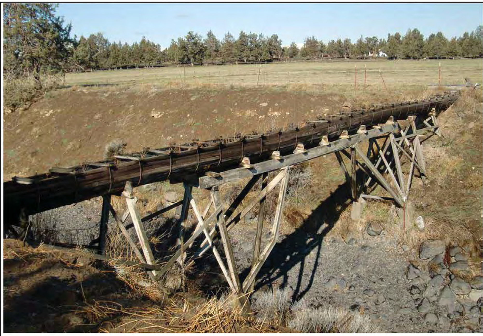
Figure 11 Wood Flume, Central Oregon Project, Deschutes County
