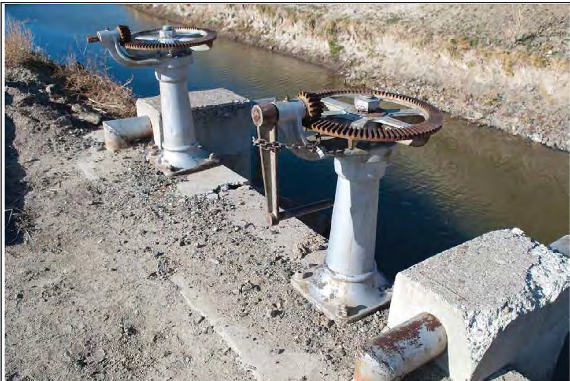
Figure 22 Pedestal Lift Headgates, Vale Project, Malheur County
