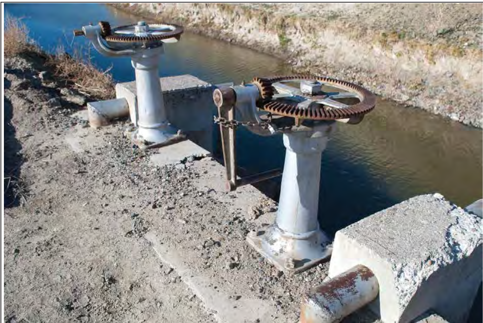
Figure 22 Pedestal Lift Headgates, Vale Project, Malheur County
