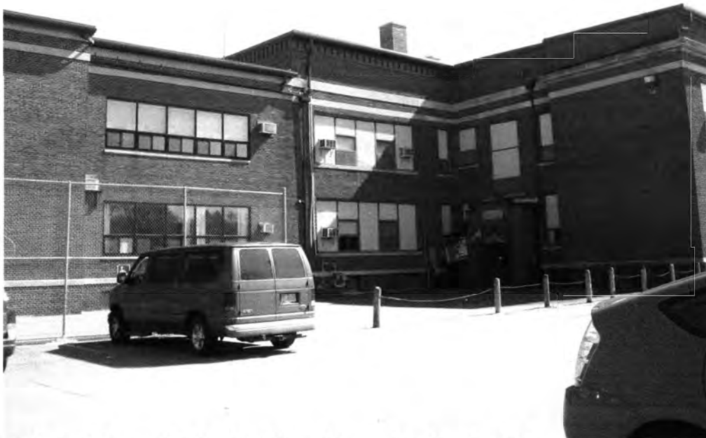
Rear of original Roosevelt School building, View to the SE with 1968 gymnasium addition to left
