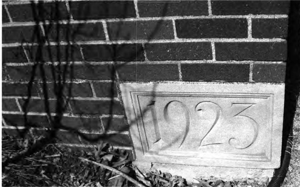
Cornerstone of original Roosevelt School building, View to the North
