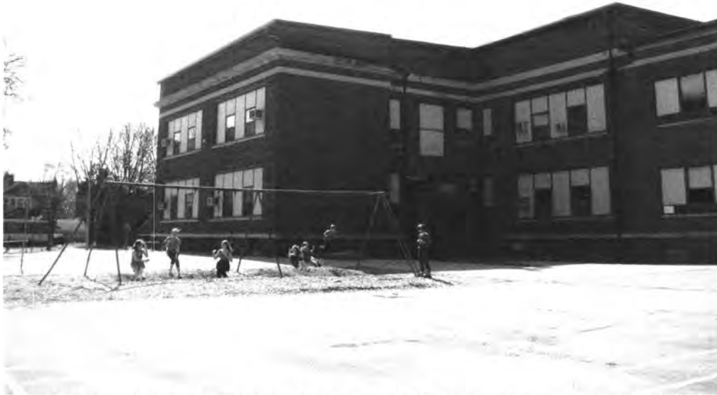
Rear of original Roosevelt School building, View to the SSW with 1968 gymnasium addition at far right.
