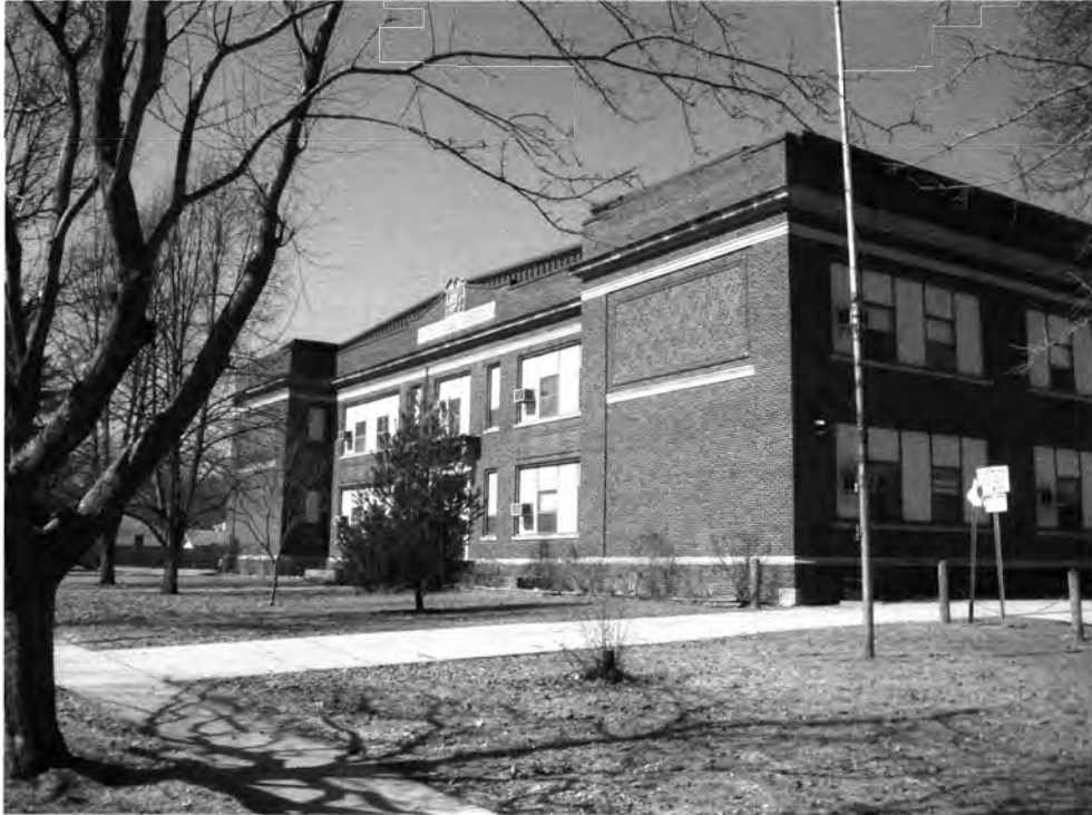
Original Roosevelt School building, View to the NW
