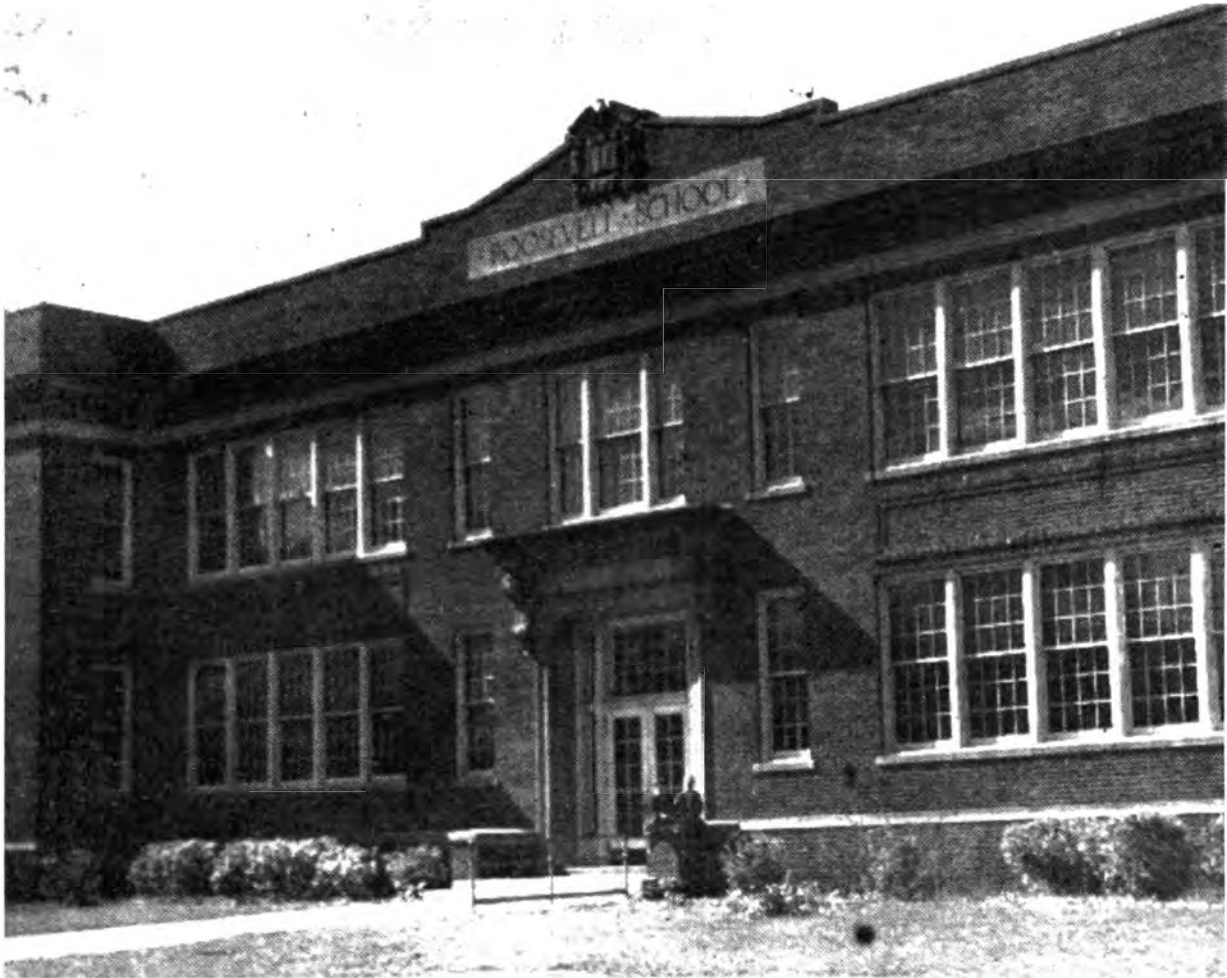
Roosevelt School, 1930s. Source: Ames Centennial Inc. 1964
