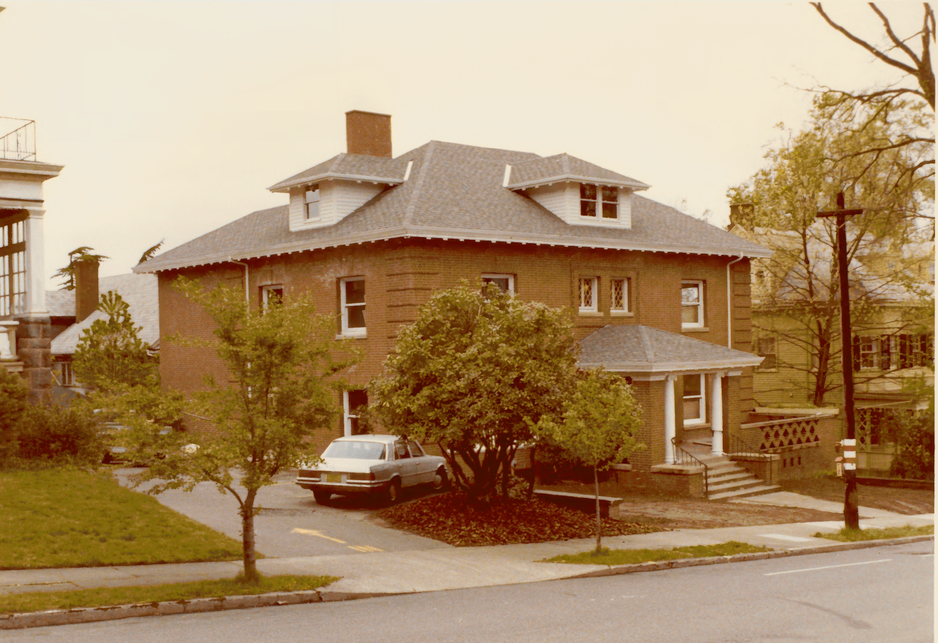
Charles F. Adams House restoration project nearing completion. May 1980
