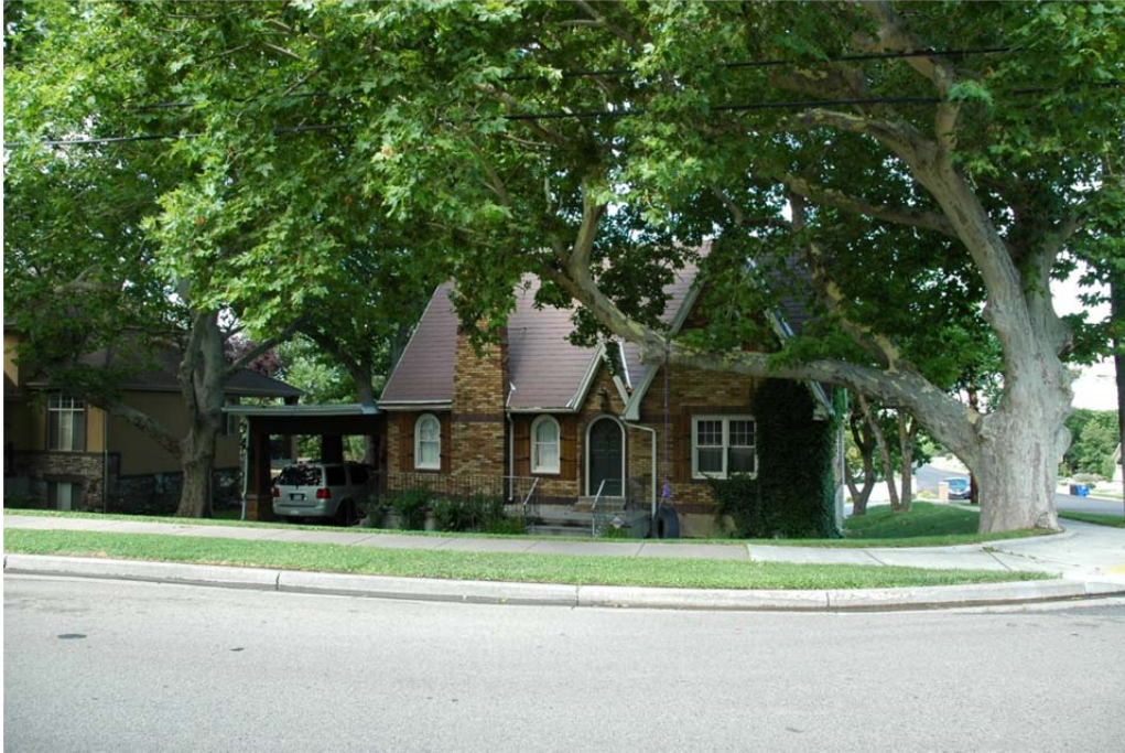
Photograph 1 East elevation of farmhouse on Main Street. Camera facing southwest.
