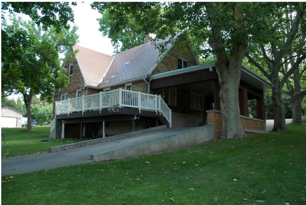
Photograph 6 South and west elevations of farmhouse. Camera facing northeast.
