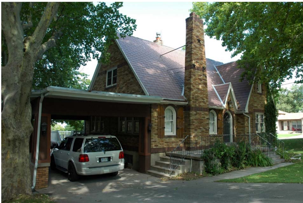
Photograph 4 East and south elevations of farmhouse. Camera facing northwest.
