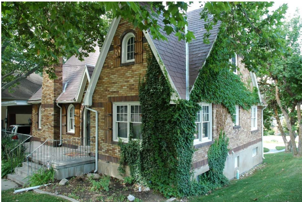
Photograph 10 East and north elevations of farmhouse. Camera facing southwest.
