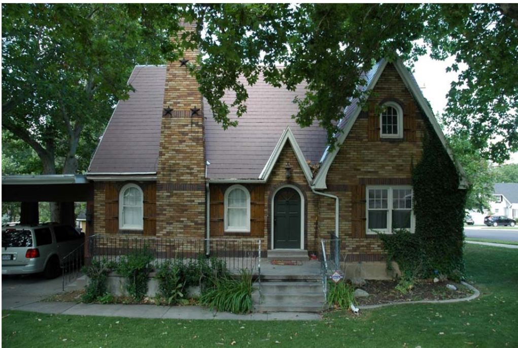
Photograph 2 East elevation of farmhouse. Camera facing west.
