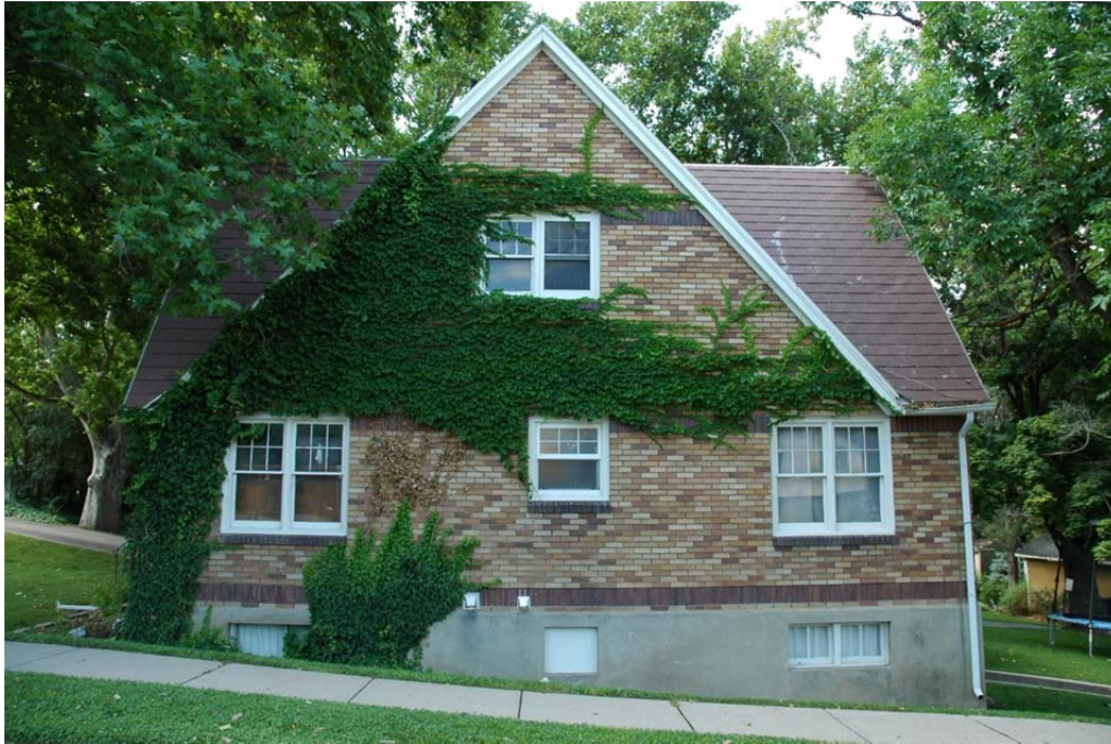
Photograph 9 North elevation of farmhouse. Camera facing south.
