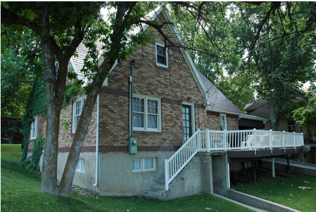
Photograph 8 North and west elevations of farmhouse. Camera facing southeast.
