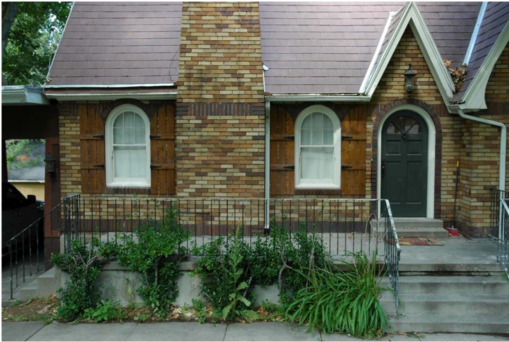
Photograph 3 East elevation of farmhouse, porch detail. Camera facing west.
