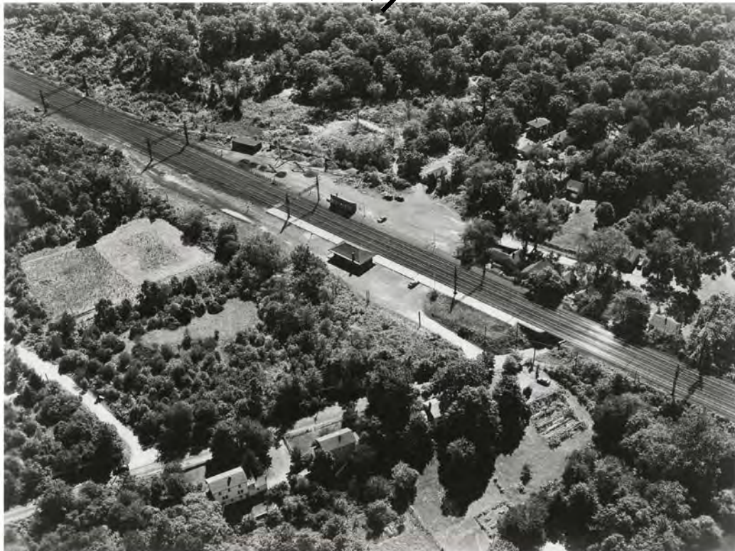
Figure 8. Rowayton Depot Historic District. Second depot building, aerial view southeast c.1950. Lisa Wilson Grant Collection.
