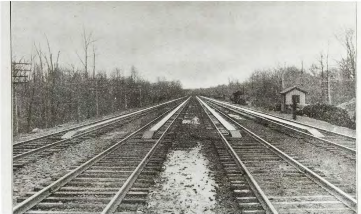
Figure 11. View west showing water tanks between tracks in 1909. (Rowayton Historical Society)
