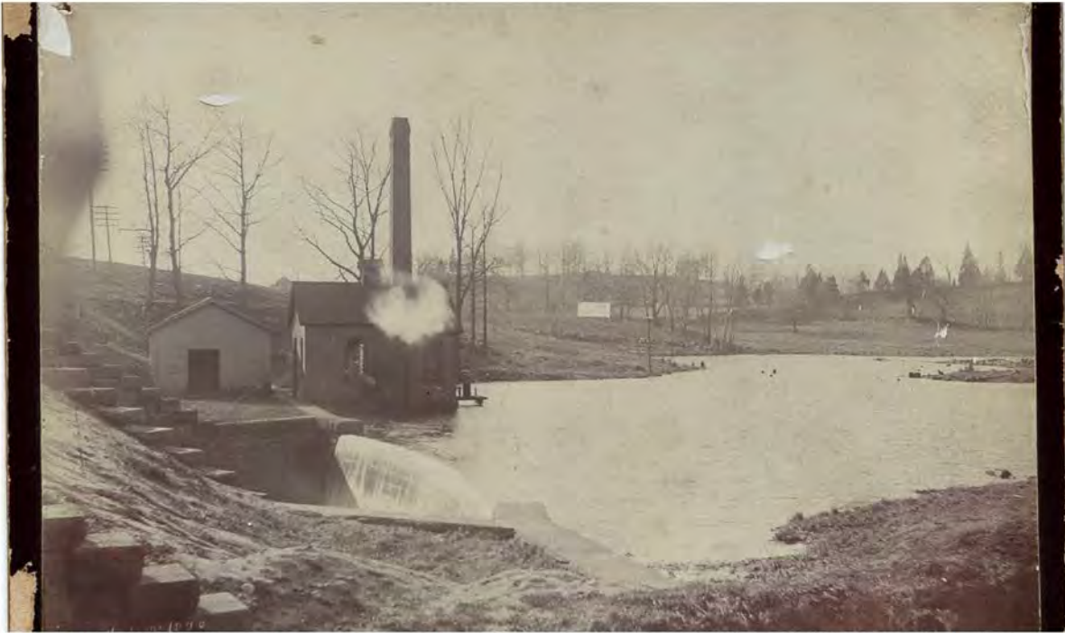
Figure 10. View west, showing pumping station at Chasmer's Pond, March 10, 1900. (Lisa Wilson Grant Collection)
