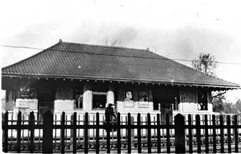
Figure 8. Second depot building, view north c. 1910. (Thomas J. Dodd Research Center, University of Connecticut)
