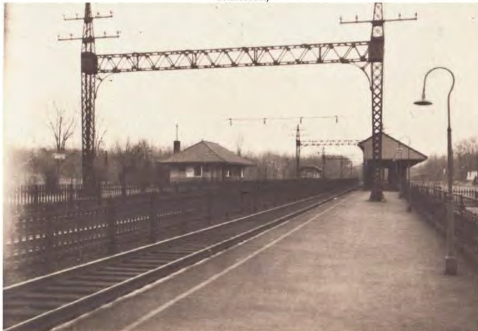
Figure 9. Showing station on north side of tracks , along with platform and shelter on south side of tracks, View northeast c. 1930. (Thomas J. Dodd Research Center, University of Connecticut)
