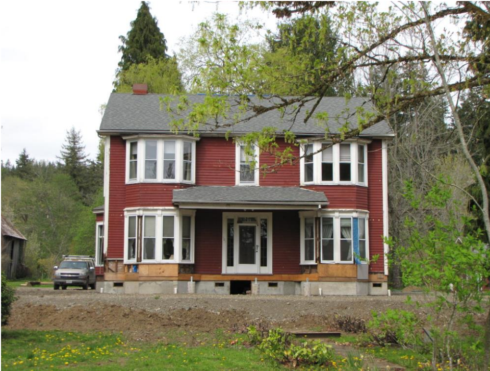
Photo #1 of 11 Hamilton-Worthington House - Main/South Façade (Nicholas Vann, Photographer)
