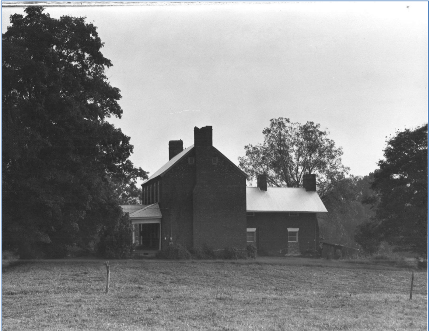
Figure 6: 1976 view of Lea House at Richland, southwest elevation.
