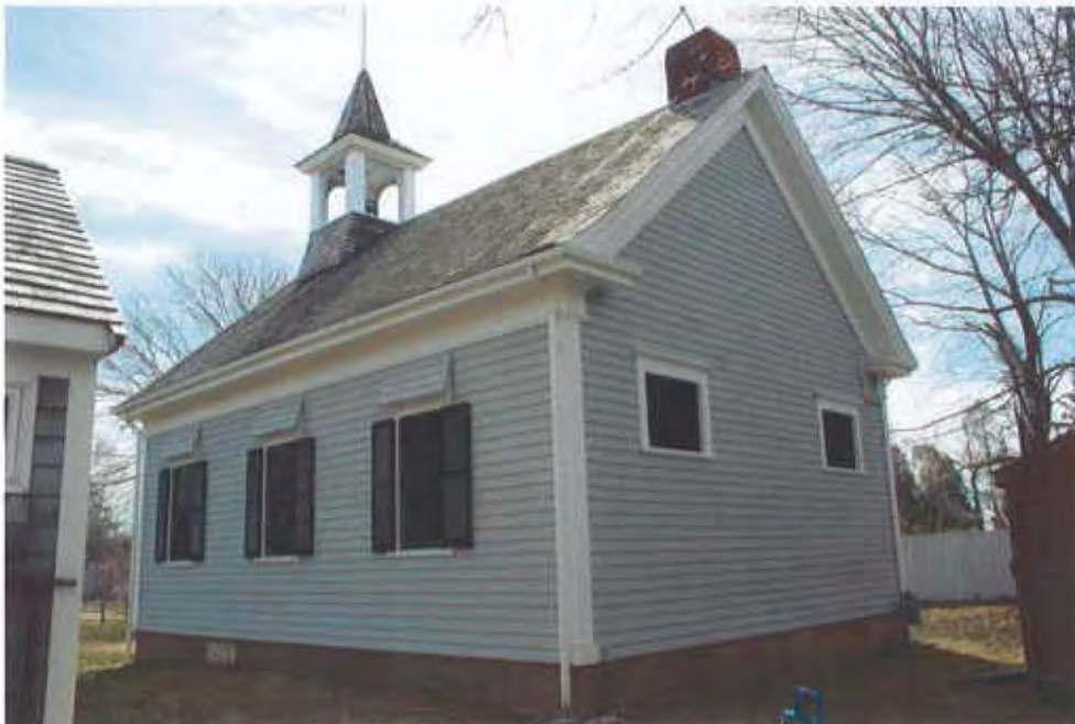
Photo 2. Schoolhouse; north (side) and west (rear) elevations, camera facing southeast.
