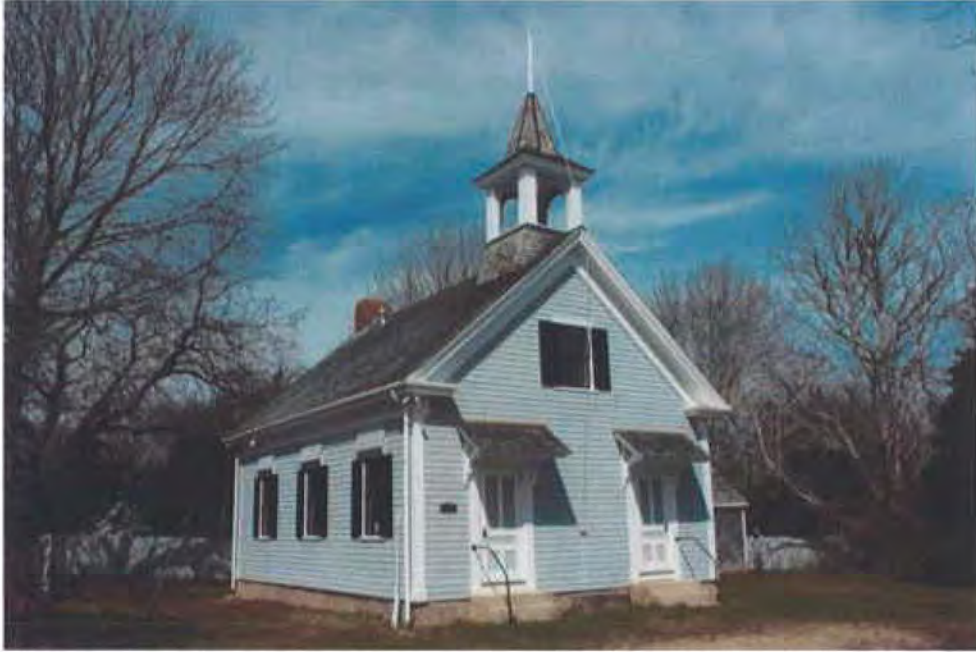
Photo 1. Schoolhouse: East façade and south elevation. Camera facing northwest.
