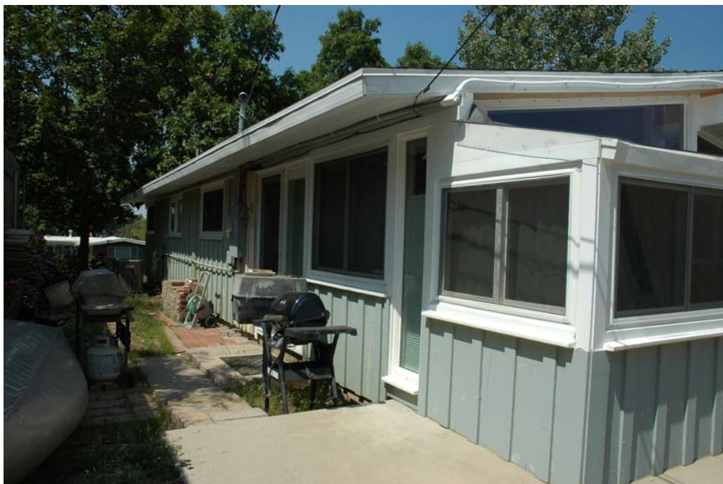
Photograph 6 South elevation of Fish-Baughman House. Camera facing west.
