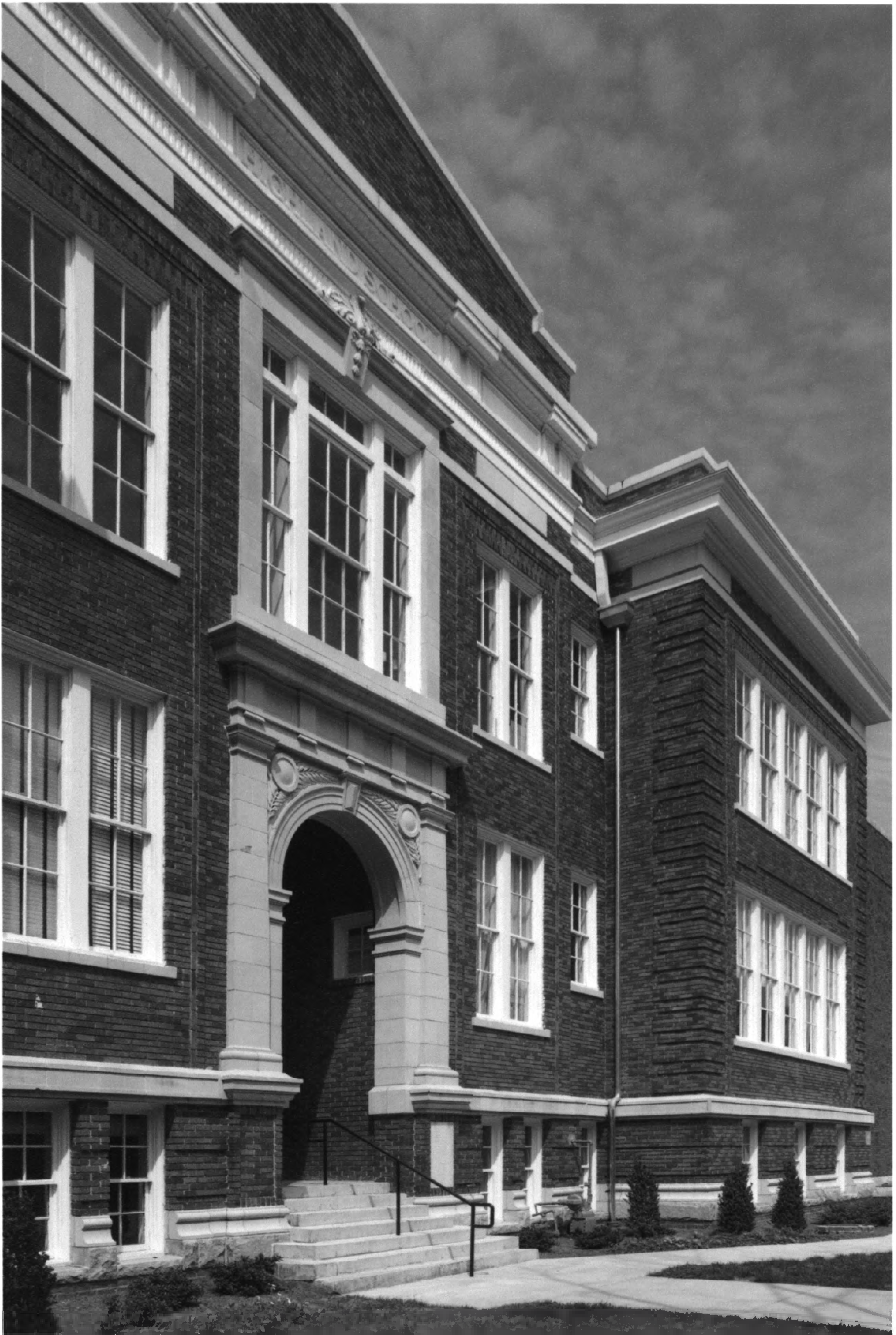
Highland School Atlanta, Fulton County, Georgia Photograph 3 of 16
