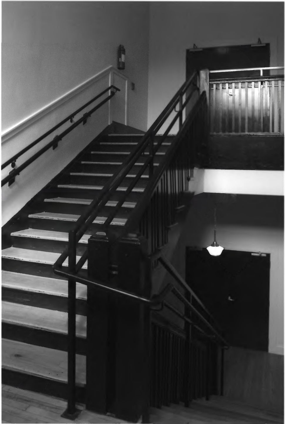
Highland School Atlanta, Fulton County, Georgia Photograph 16 of 16
