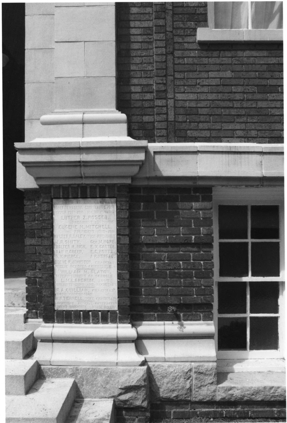
Highland School Atlanta, Fulton County, Georgia Photograph 5 of 16
