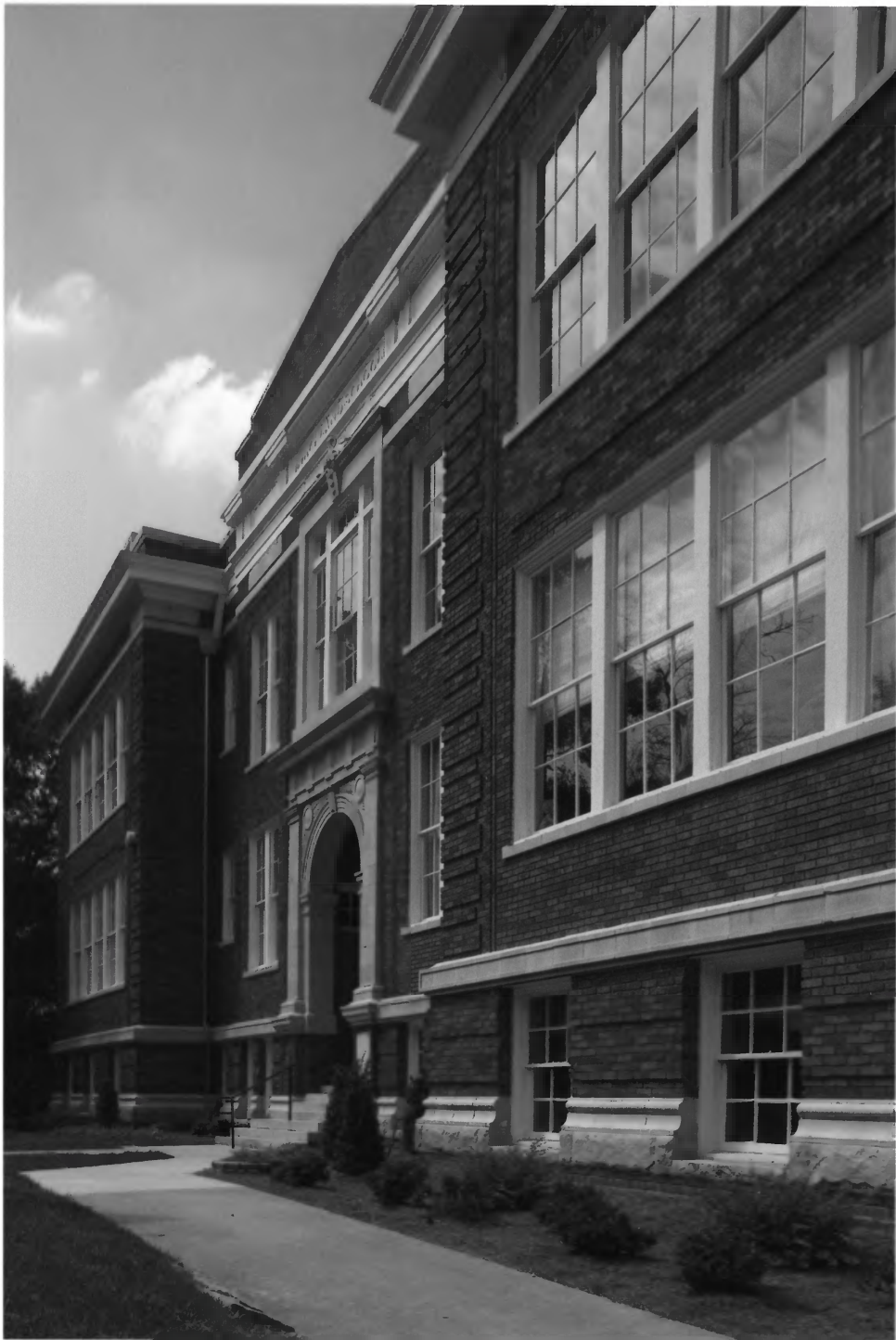
Highland School Atlanta, Fulton County, Georgia Photograph 4 of 16
