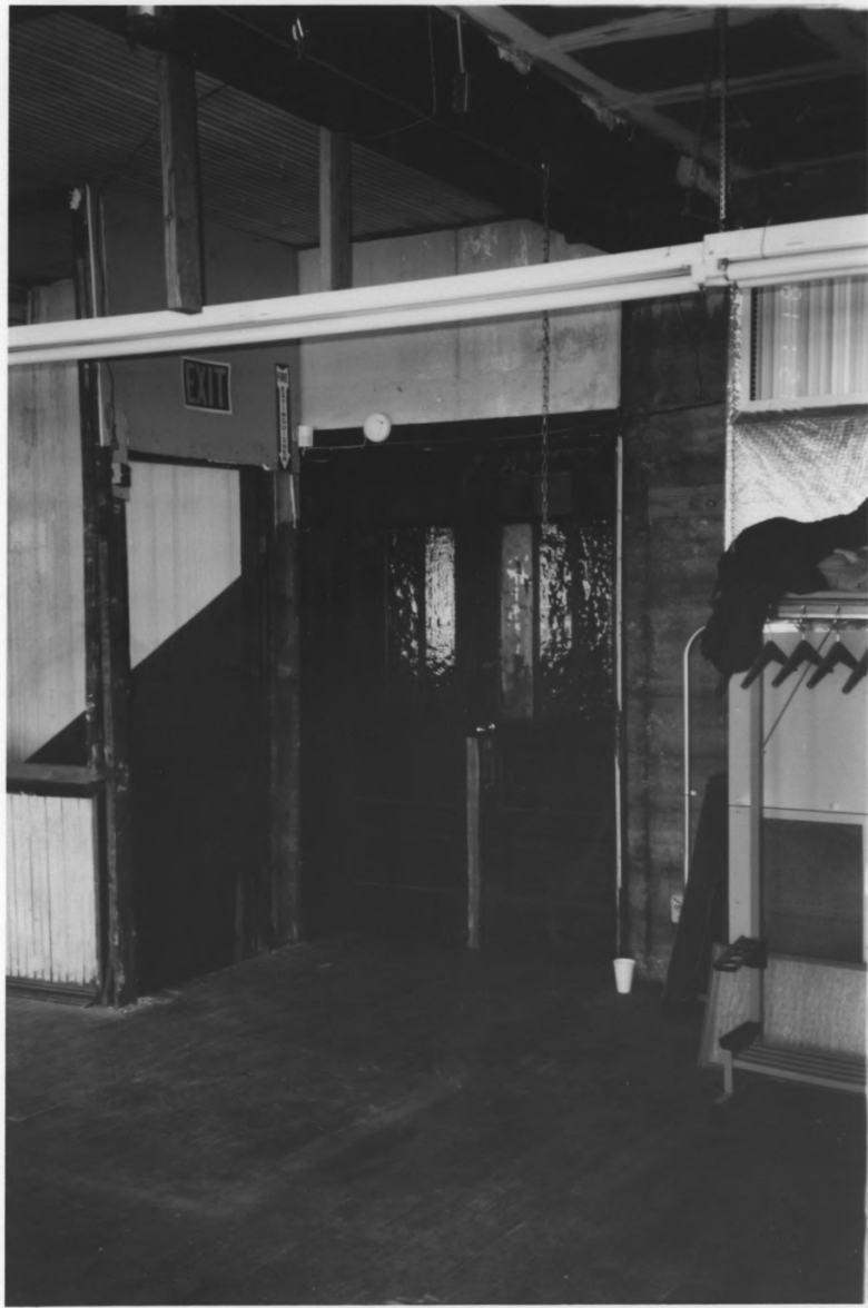
Mollyneux Chevrolet Company / Rockwood Fire Department Building Rene Co. TN
