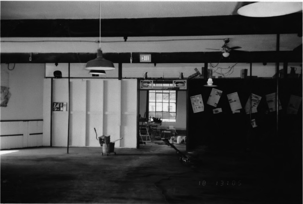
Molynex Chevrolet Company / Rockwood Fire 17 of 27 Department Building Boone Co
