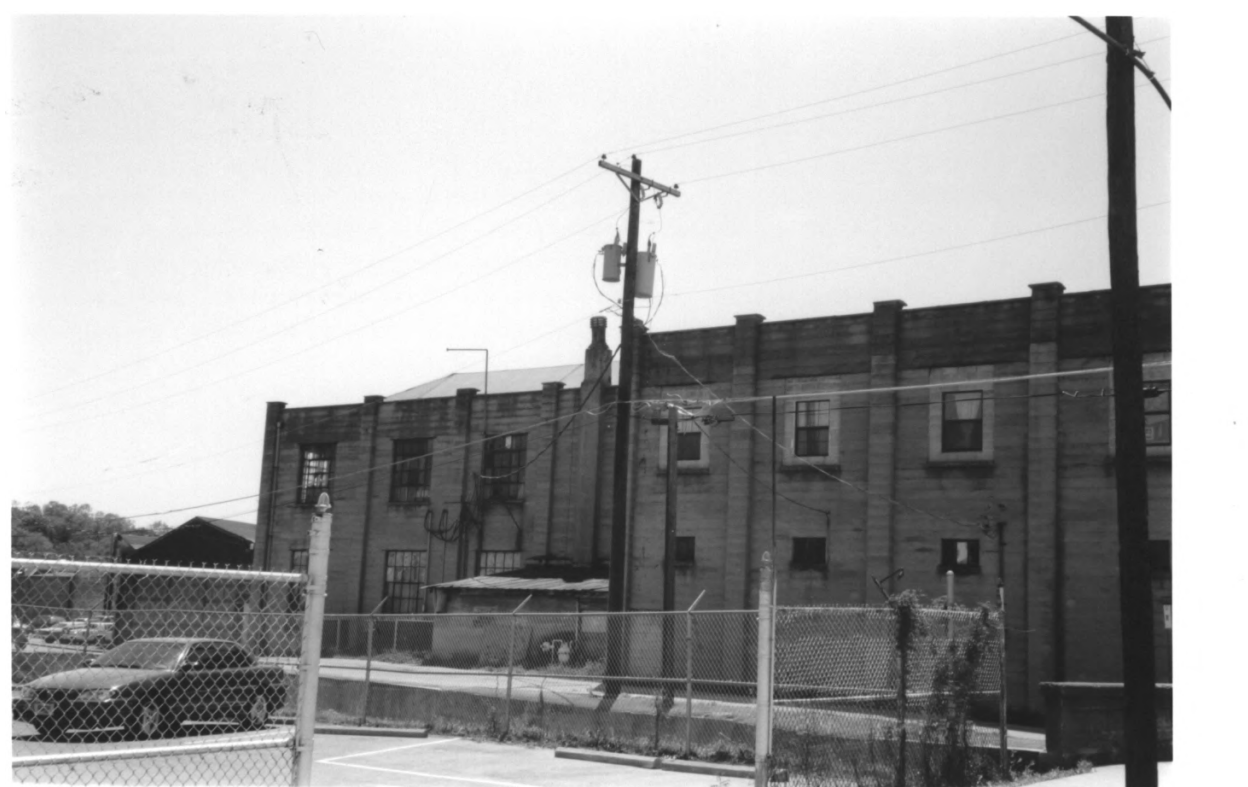
Molyneux Chevrolet Company/ Rockwood Fire Department Building Roane Co. 5 of 27
