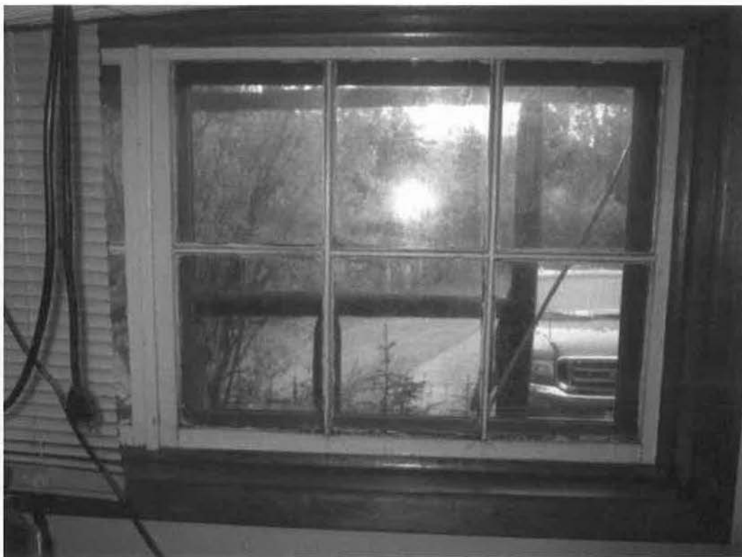
Figure 82- Window #3, from window schedule (Figure 5 Figure 6). (NPS Photo, August 2012).
