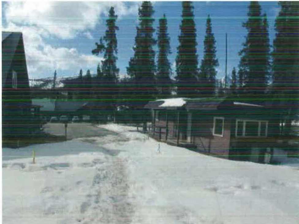
Figure 12- B141 is building on right side of photo, proposed relocation of P-22- overview south. Taken from headquarters trail.
