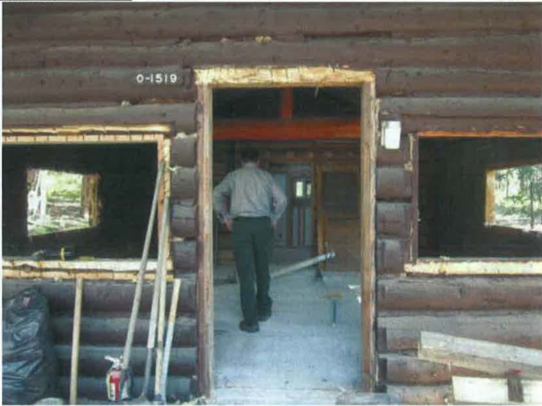
Figure 99- After removal of modern interior, windows, and door (NPS Photo, August 2013).
