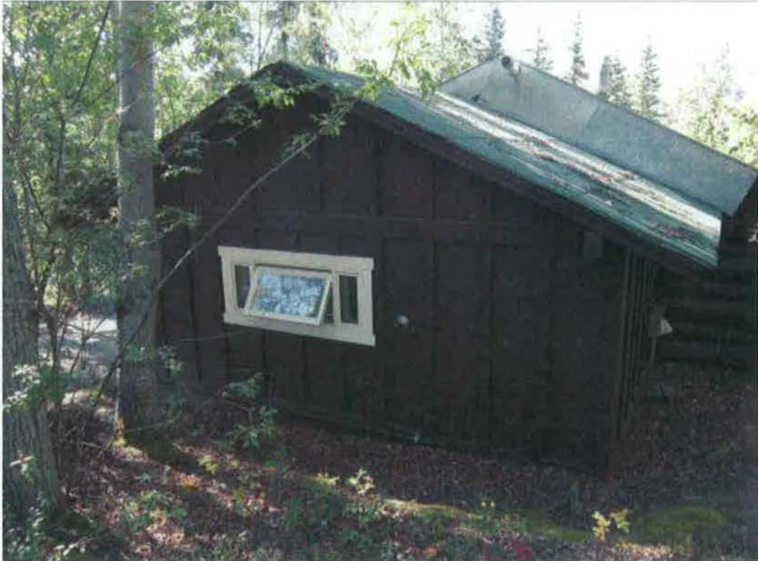
Figure 66- 1979 addition, N elevation. (NPS Photo, August 2012).
