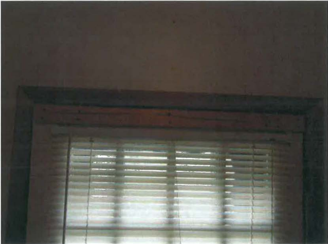
Figure 78- Reinforcement added at top of entry door. (NPS Photo, August 2012)
