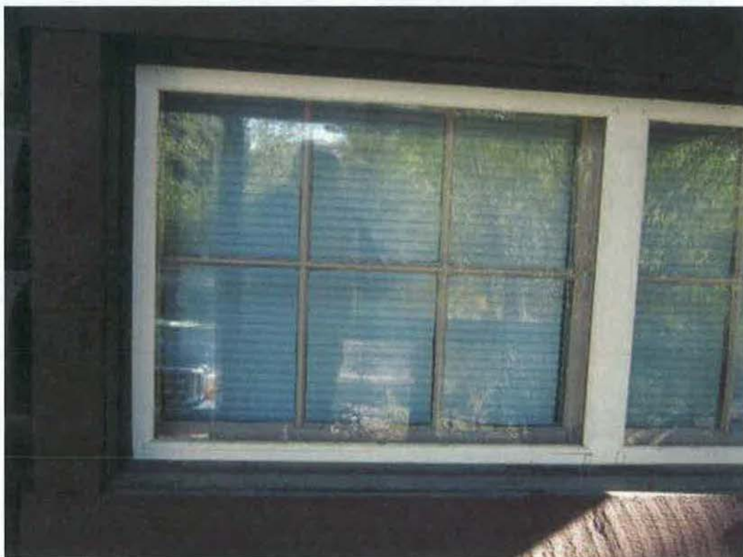
Figure 47- Window #3, from window schedule (Figure 5 Figure 6). (NPS Photo, August 2012).
