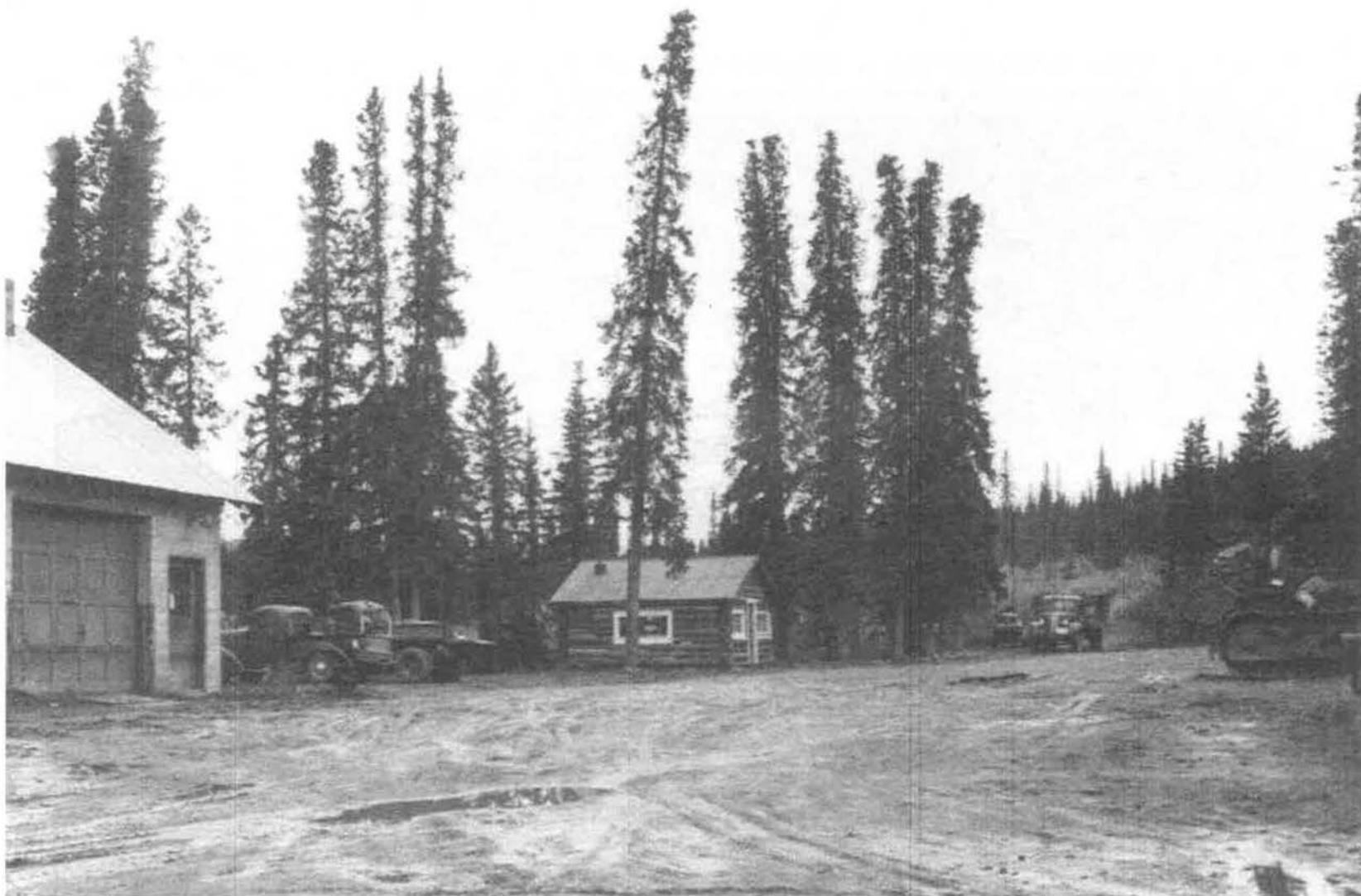
Figure 21- View of P-22 at second location after its first move in 1950. Building 118 is in the foreground on the left, looking to the southwest (DENA 3-18, Denali National Park and Preserve Museum Collection, September 12, 1950)
