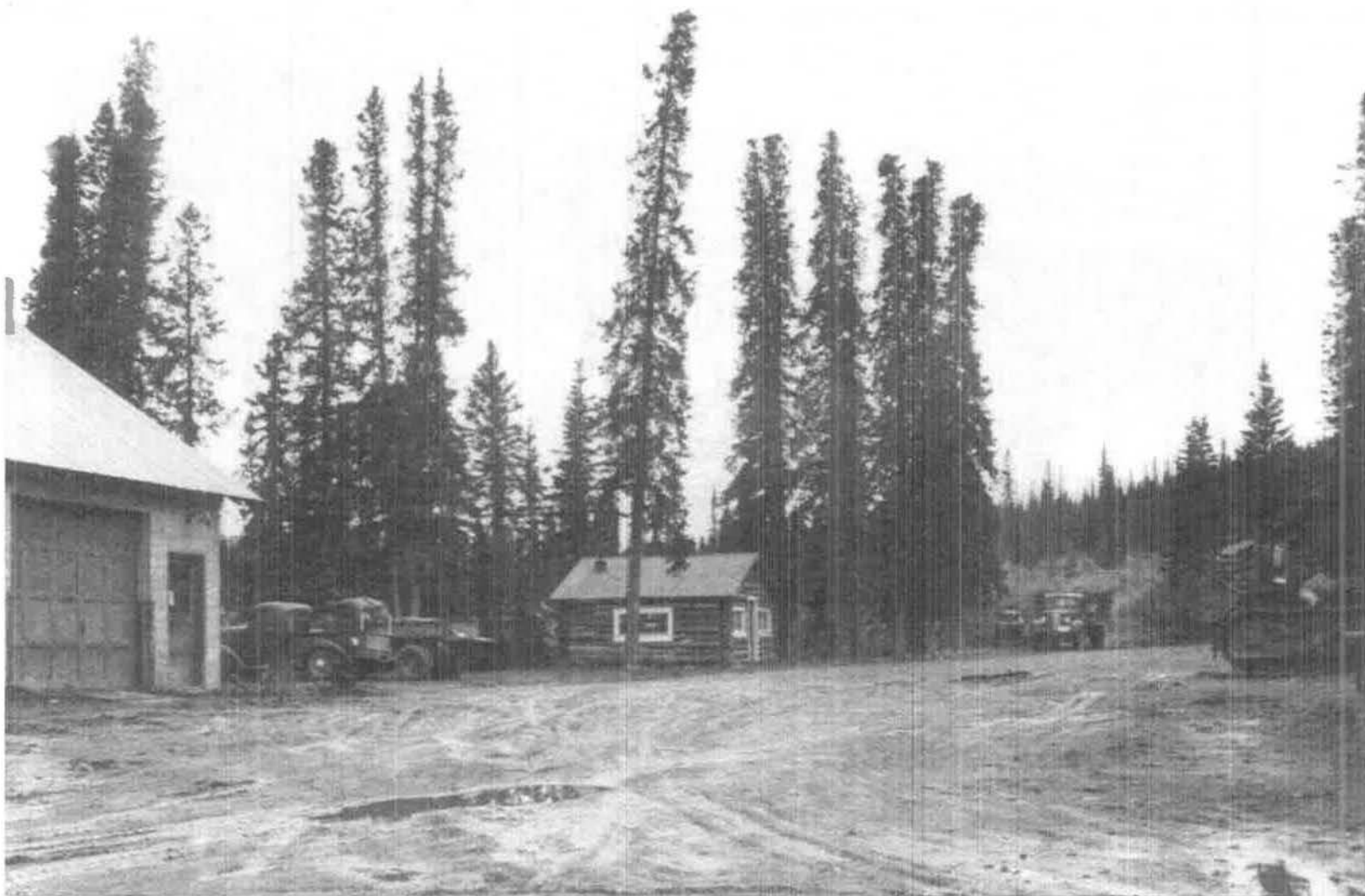
Figure 30- View of P-22 at second location after its first move in 1950. Building 118 is in the foreground on the left (DENA 3-18, Denali National Park and Preserve Museum Collection, September 12, 1950)
