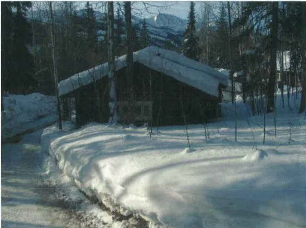
Figure 71- N elevation of addition – note hillside sloping into addition. NPS Photo, February 2012).
