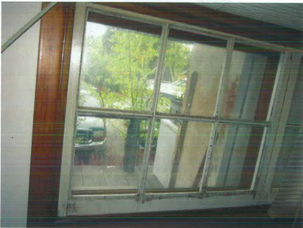
Figure 81- Window #2, from window schedule (Figure 5 Figure 6). (NPS Photo, August 2012).
