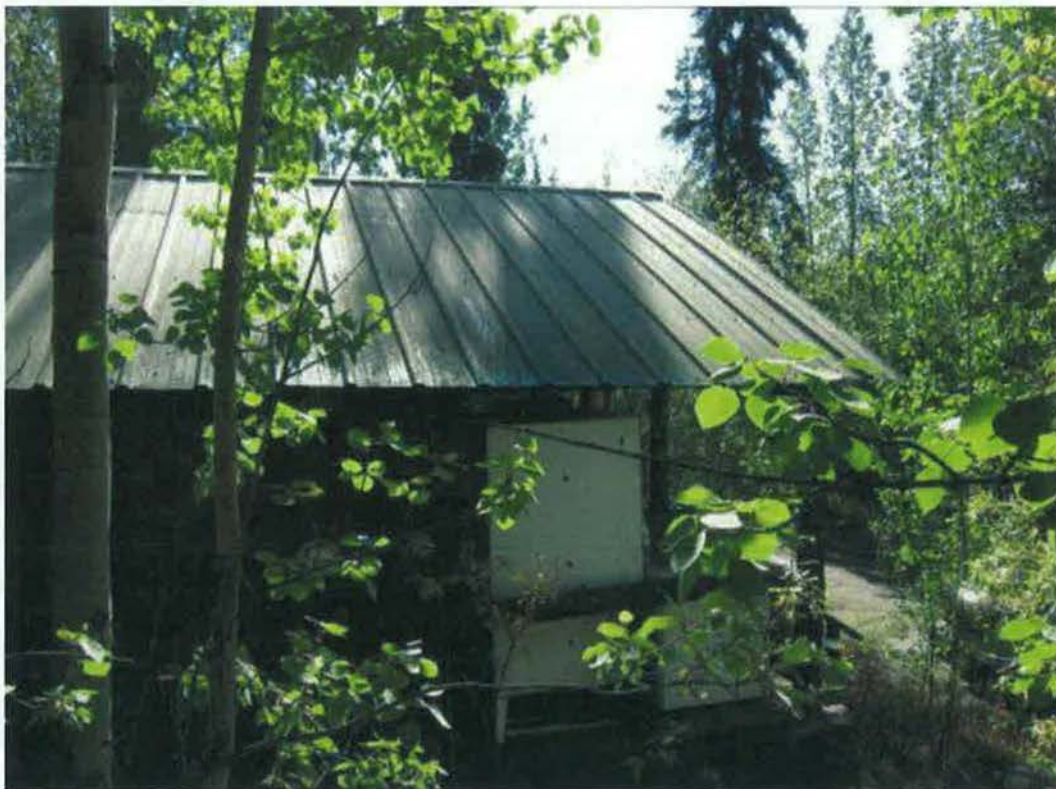
Figure 58- West elevation and roof. (NPS Photo, August 2012).
