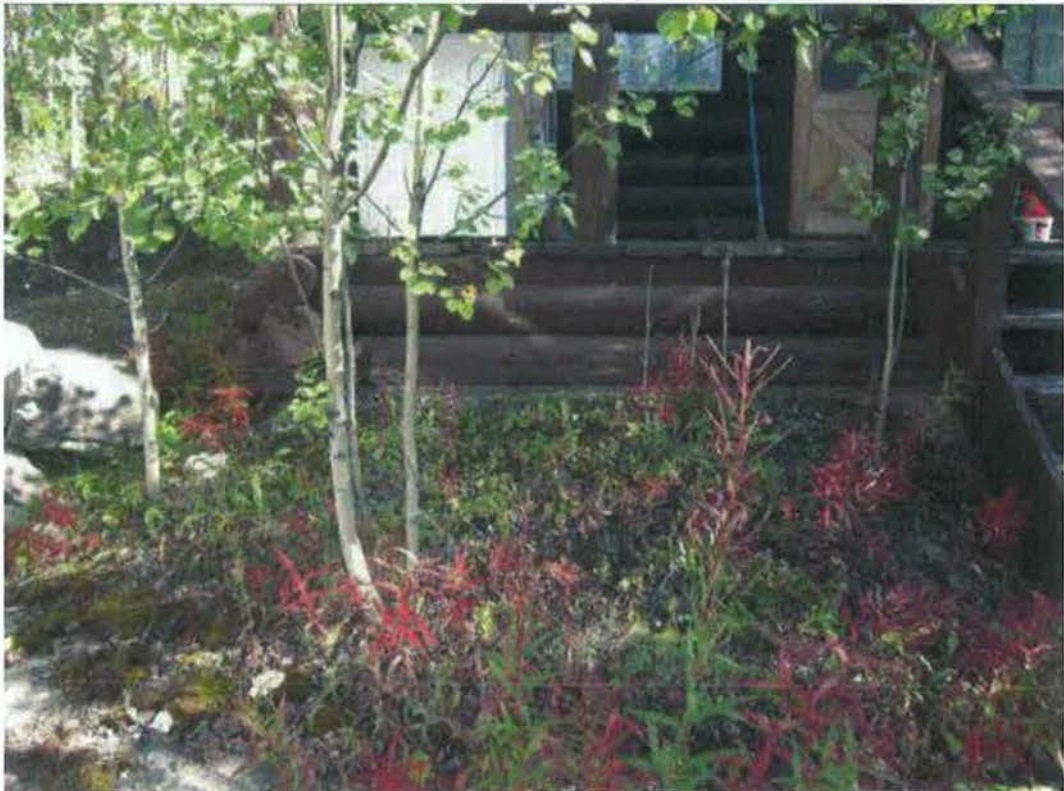
Figure 39- W end of S elevation of porch. (NPS Photo, August 2012).
