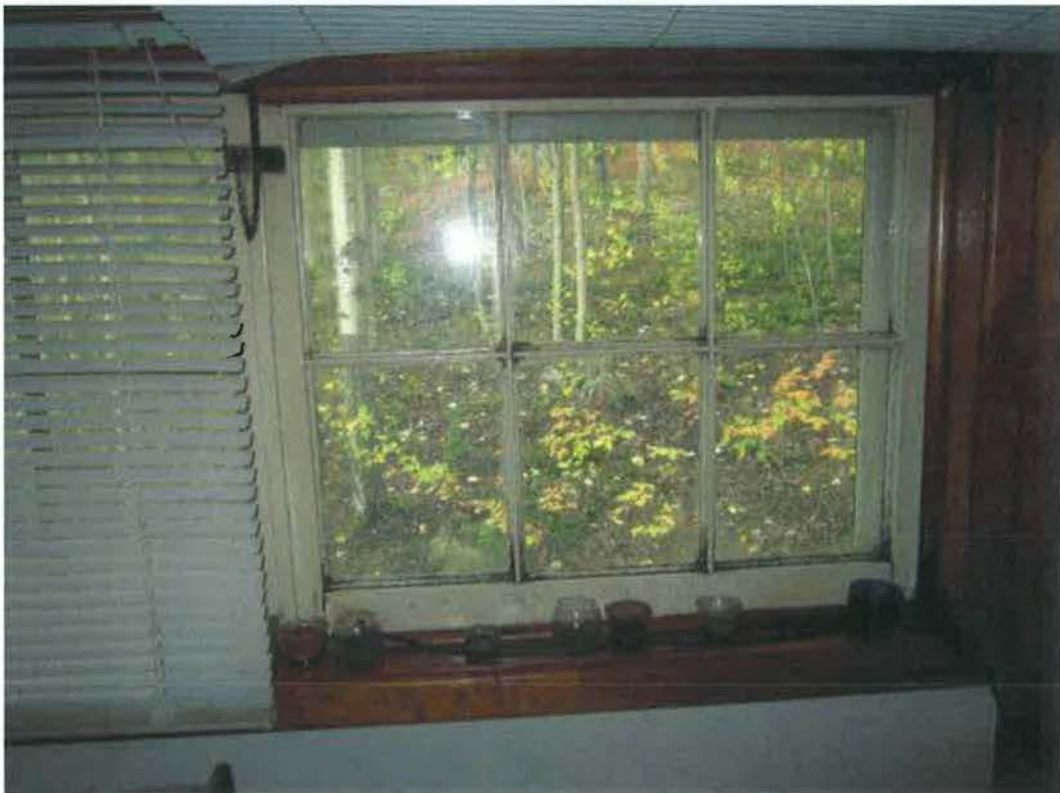
Figure 91- Window #8, from window schedule (Figure 5 Figure 6). (NPS Photo, August 2012).
