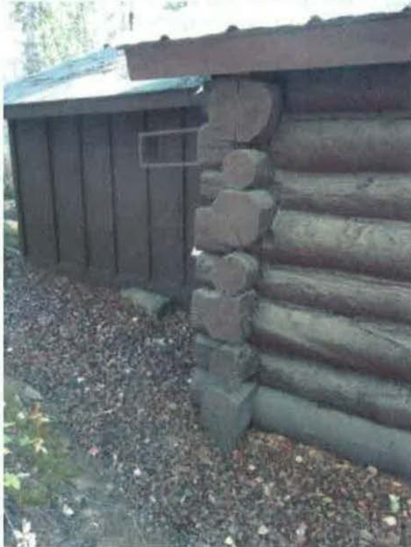
Figure 63- NW elevation of original building. (NPS Photo, August 2012).
