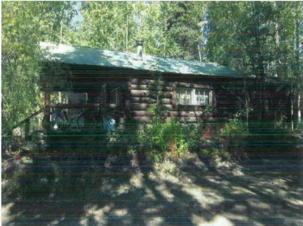
Figure 69- East elevation. (NPS Photo, August 2012).
