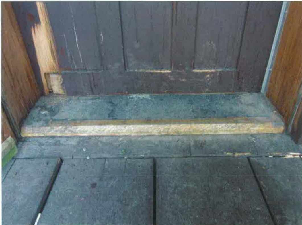
Figure 55- Threshold. (NPS Photo, August 2012).
