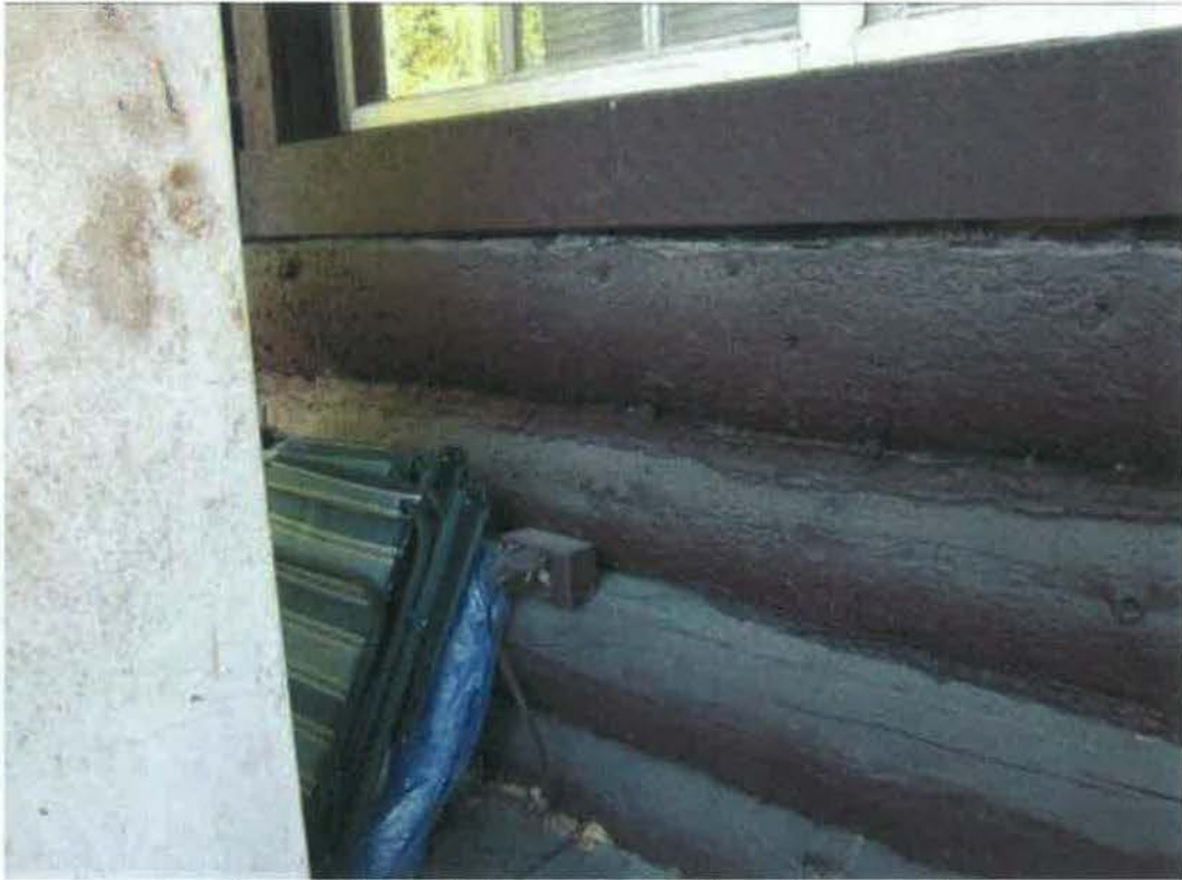
Figure 50- Electrical Outlet. (NPS Photo, August 2012).
