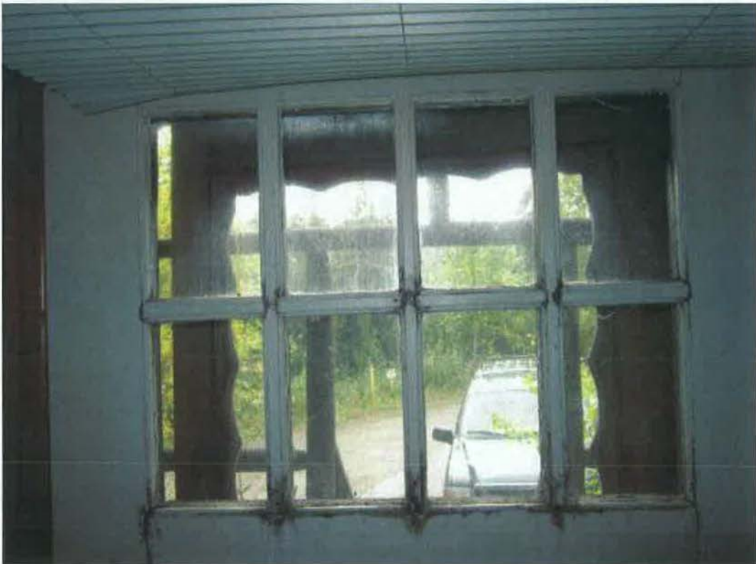
Figure 75- Entry door lites. (NPS Photo, August 2012)
