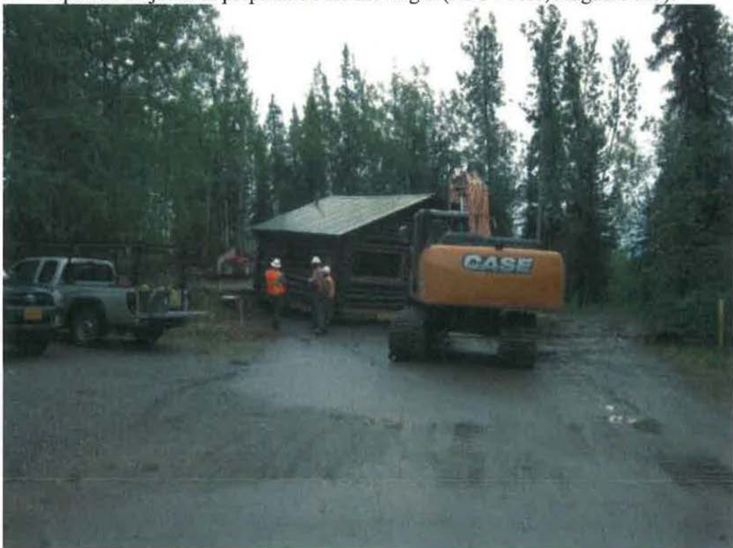
Figure 104- P-22 being moved off its foundation (NPS Photo, September 2013).
