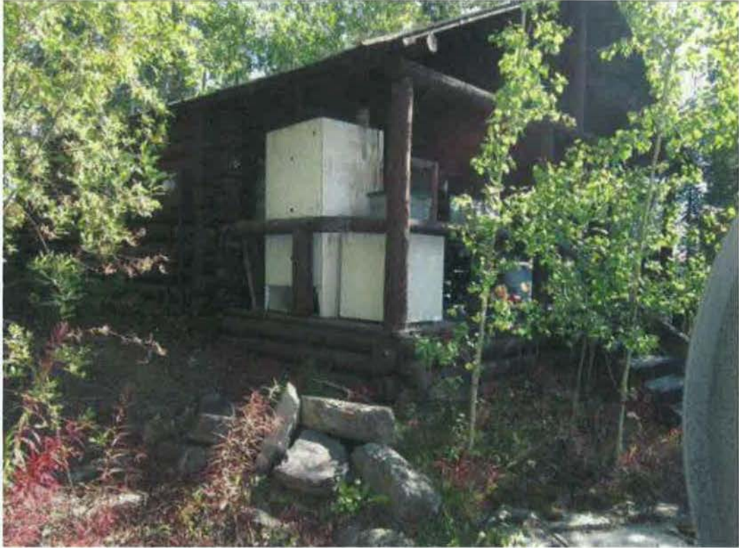
Figure 38- SW elevation. (NPS Photo, August 2012).
