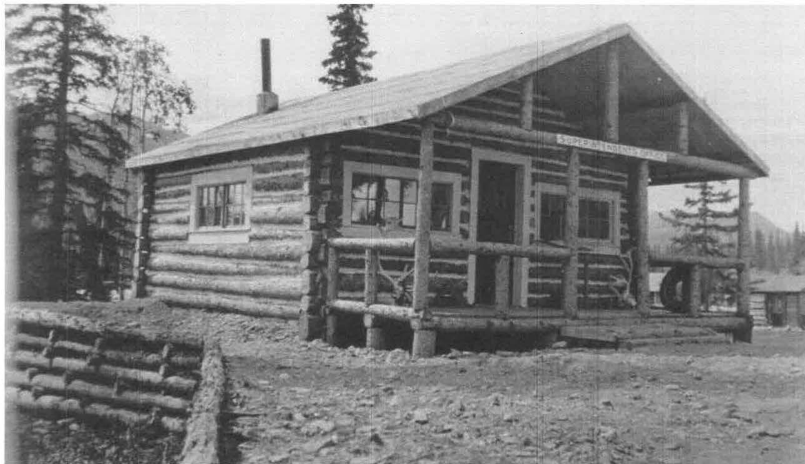
Figure 25- View of P-22 at original location looking southwest (Candace Waugaman Collection, 1920's).
