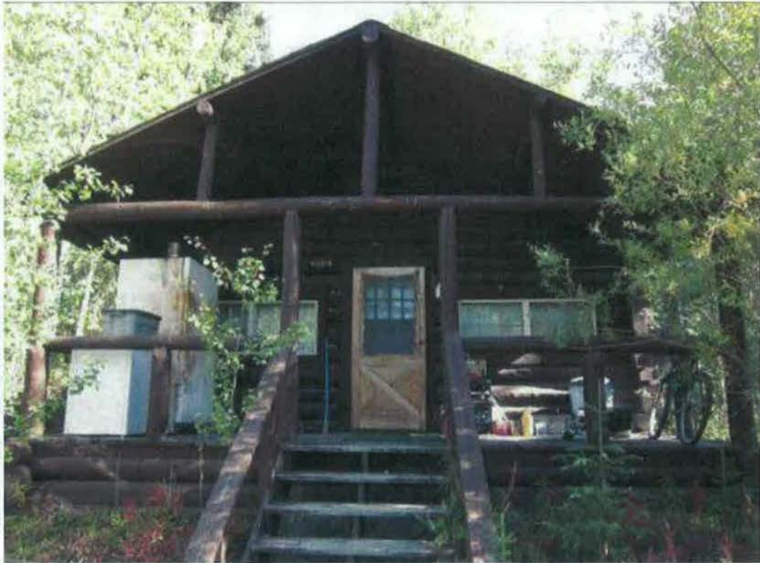
Figure 42- S elevation. (NPS Photo, August 2012).
