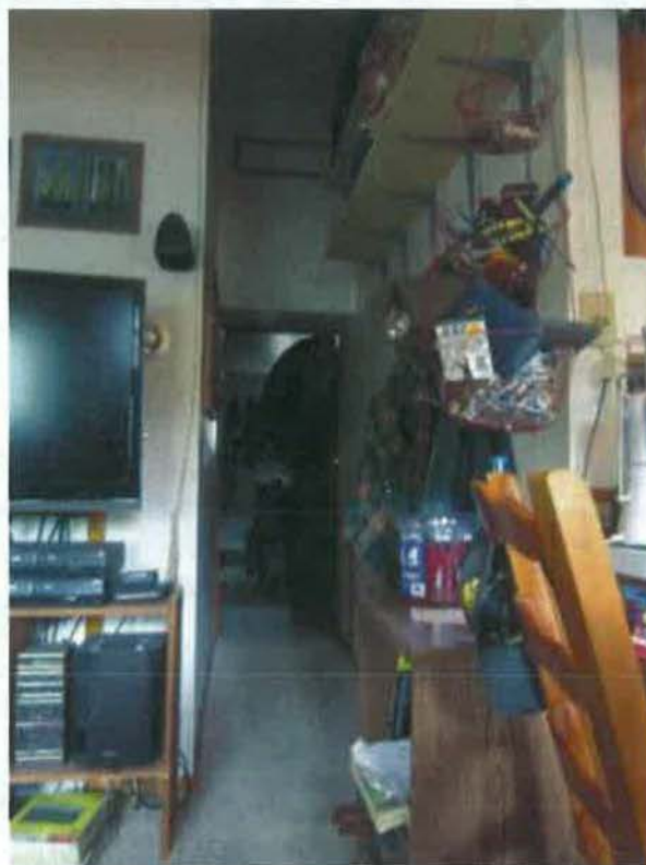
Figure 96- Hall leading to rear addition. (NPS Photo, August 2012).
