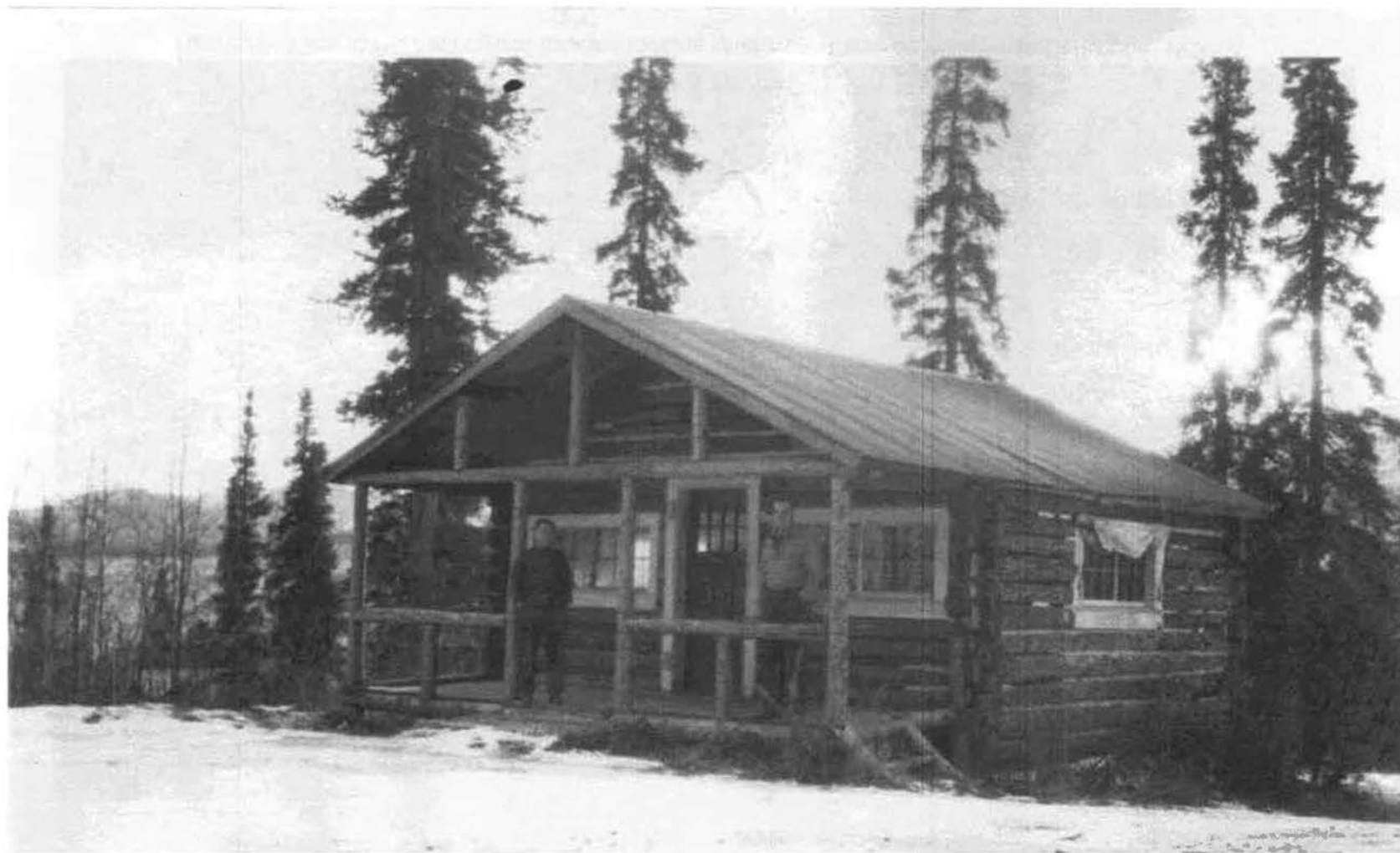
Figure 23-Original location of P-22 with the structure in “unfavorable” and “unsightly” appearance (November 1940, Denali National Park and Preserve Museum Collections). Note access to the porch from the west which will be duplicated after the proposed relocation.
