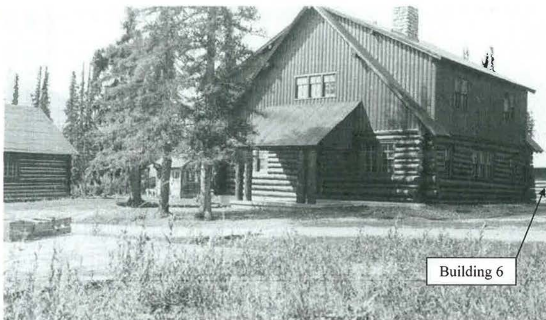
Figure 14- 1934 Photo of Building 21 with Building 6 in the background (DENA 3 26, Denali National Park and Preserve Museum Collection)
