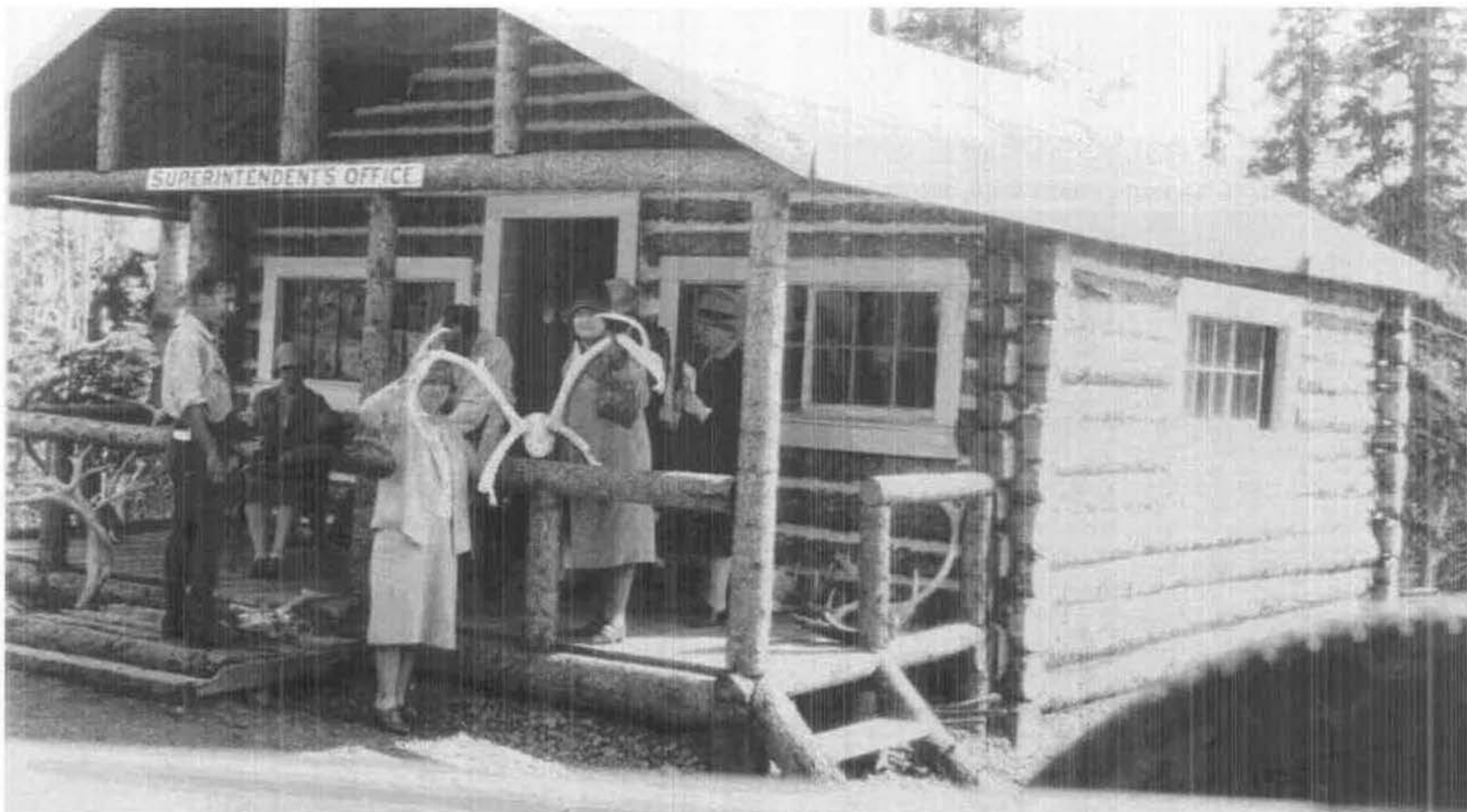
Figure 26- View of P-22 at original location looking southeast (DENA 14976, Haskell Photo, Denali National Park and Preserve Museum Collection, 1927). Note access to the porch from the west which will be duplicated after the proposed relocation.
