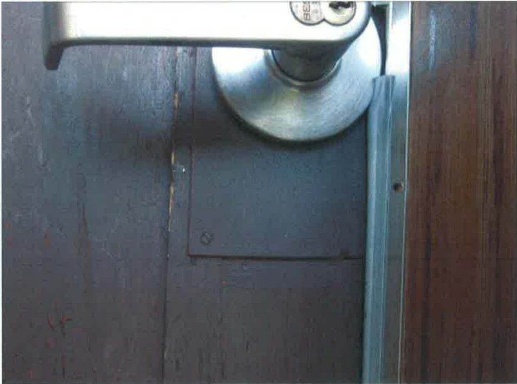
Figure 54-Entry Door hardware. (NPS Photo, August 2012).
