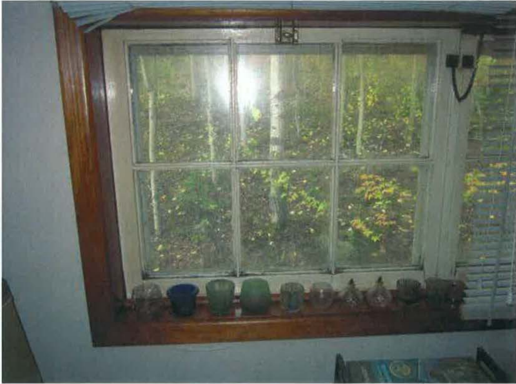
Figure 90- Window #9, from window schedule (Figure 5 Figure 6). (NPS Photo, August 2012).
