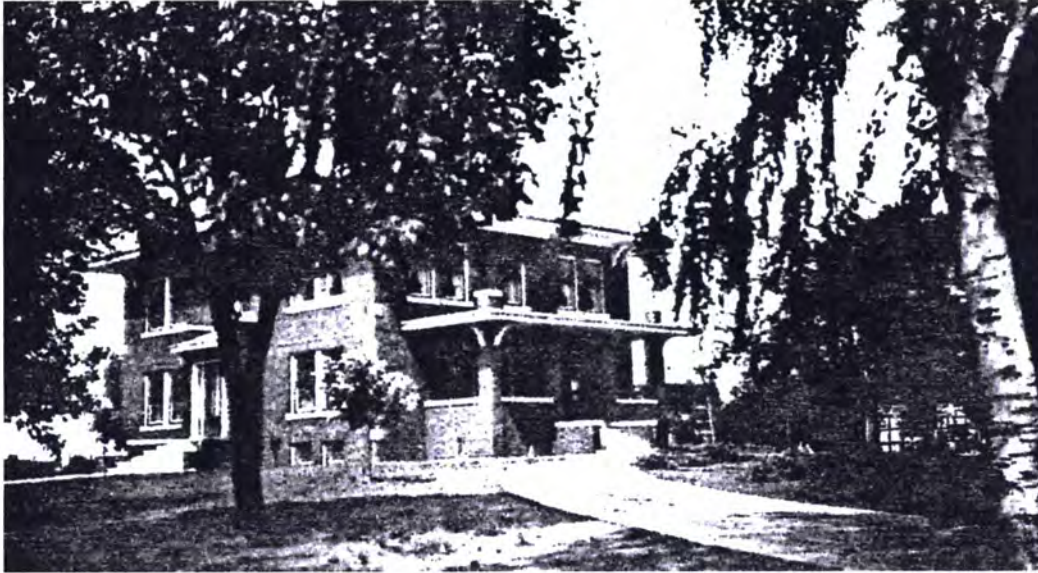
Figure 13 Façade and south elevations, circa 1920 (Courtesy of Bonnie Brown Martin)
