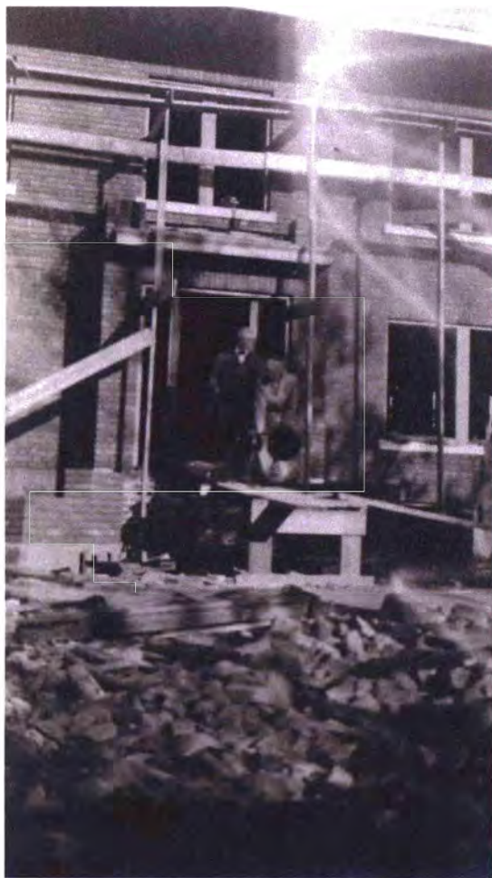
Figure 9 J.T. and Mollie Crozier at their front door during construction, 1918 (Courtesy of Bonnie Brown Martin)
