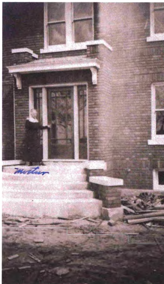
Figure 10 Mollie Crozier at the front door with the completed entry steps, 1918 (Courtesy of Bonnie Brown Martin)
