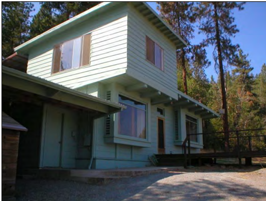
Figure 14: The "Little House," Looking North, with c1963 Addition, 2009 (Pacifica Collection)
