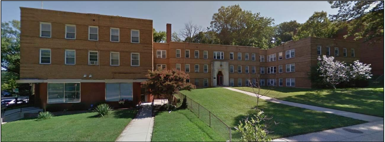
Apartment building at 3300 Pennsylvania Avenue, S.E., designed by Evan J. Conner in 1939. It is very similar in plan to that of Duvall Manor, however Conner designed the building in the Art Deco, rather than the Colonial Revival, style.
