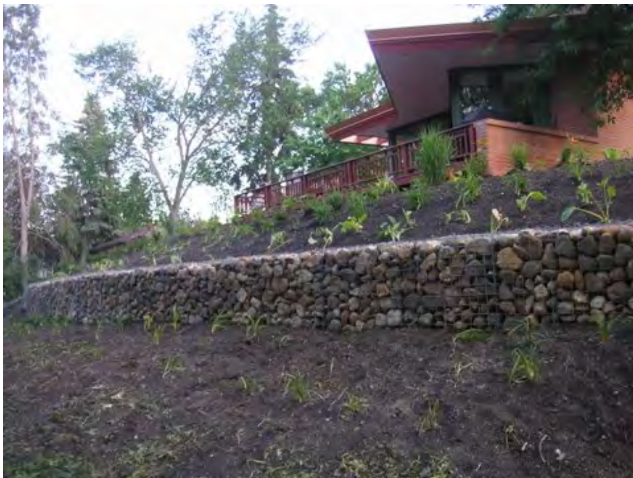
Flood levee and plantings done in 2012, taken June 25, 2012.
