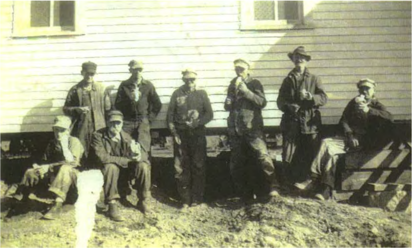
Figure 4. Men digging the new basement for the church in 1938. From left to right in the 1938 church photo of the local parishioners' hand-digging the basement are: Ottenus Bakke, Carl Gilbertson, Morris Sorum, Alfred Anderson, Louis Gjelfe, George Rekansrud, Wil Rud (Rood), and Harry Sorum. (Source: Mel Anderson, Waverly, Iowa)
