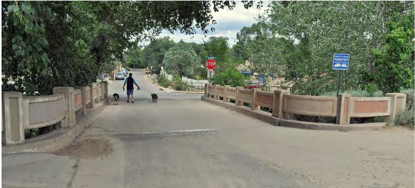
Photo 2 of 6: Bridge deck and railing, photographer looking north.
