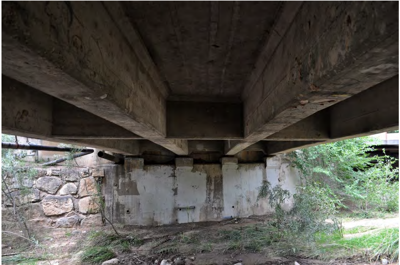
Photo 5 of 6: Deck-girders and north abutment, photographer looking north.
