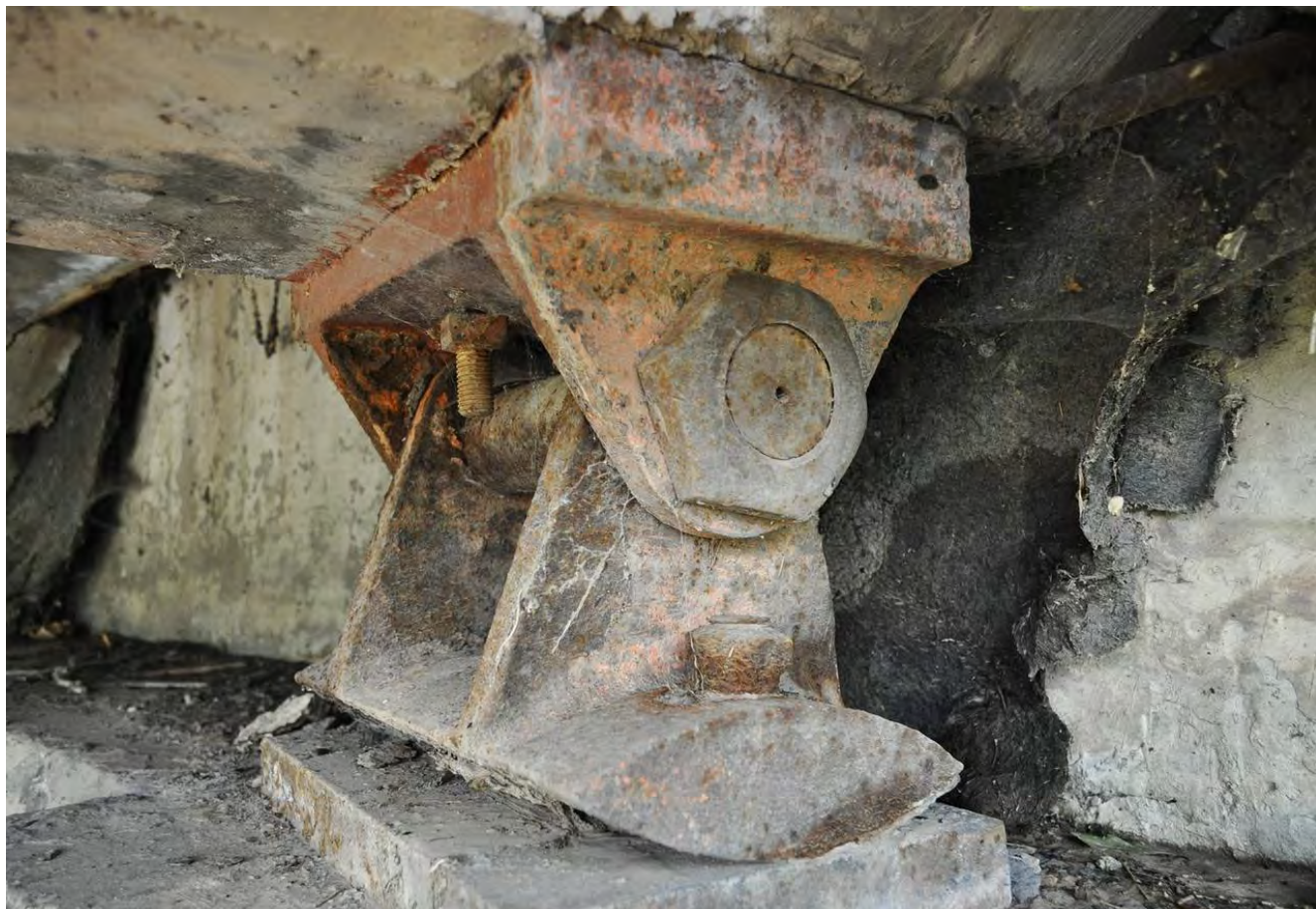
Photo 6 of 6: Pin-type cast-steel rocker bearing assembly, photographer looking southeast.
