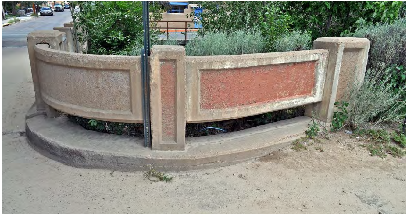
Photo 3 of 6: Curved section of railing, photographer looking north.
