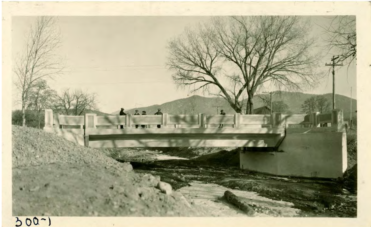
300-1 "Canyon Road Bridge, Santa Fe," 1928. New Mexico State Highway and Transportation Photograph Collection, Image No. 74006 Box SN 24203, folder 283 to 300 Courtesy of the New Mexico State Records Center and Archives 1205 Camino Carlos Rey, Santa Fe, New Mexico 87507
