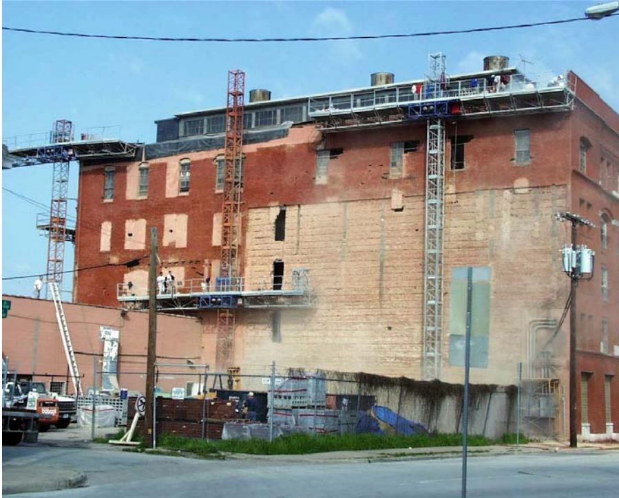
South façade after window openings were cut in, by contractor for Spray-O-Bond Masonry Repair March 2001
