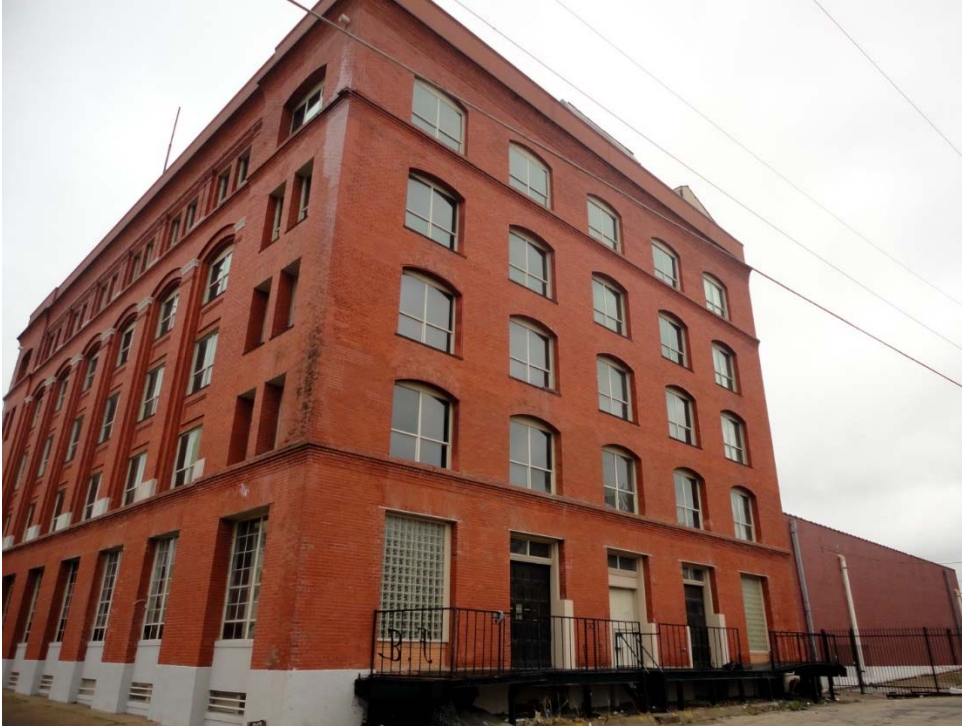
Photo 3 North and west facades
