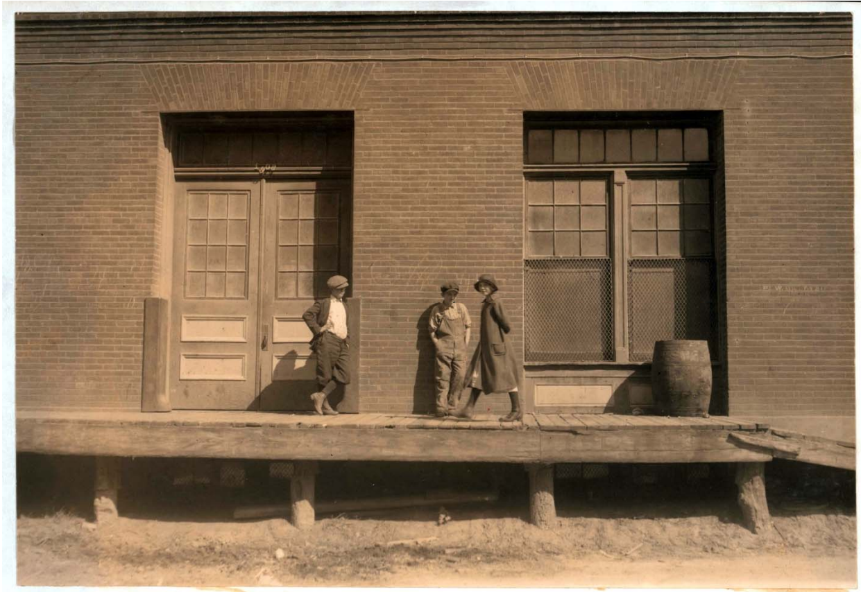
Hughes Bros. workers, loading dock on west façade, photo taken October 1913.
