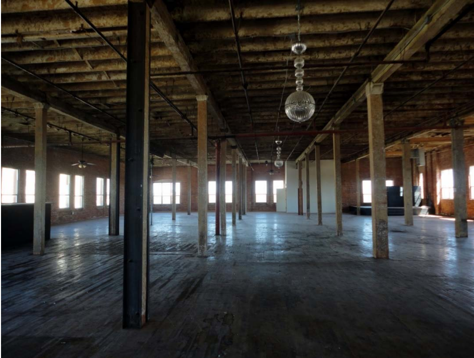
Photo 15 Floor 5 camera facing east
