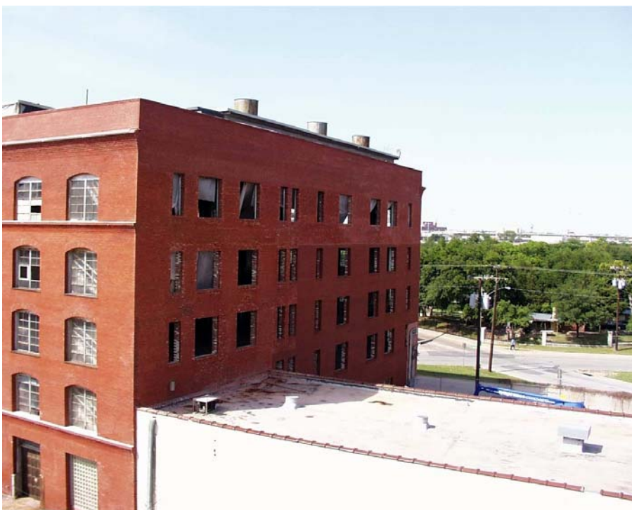
South façade after window openings were cut in, by contractor for Spray-O-Bond Masonry Repair March 2001
