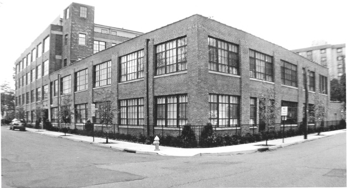
Interstate Hosiery Mills, Inc. Mill Building, Twp. of Bloomfield, Essex County, NJ
