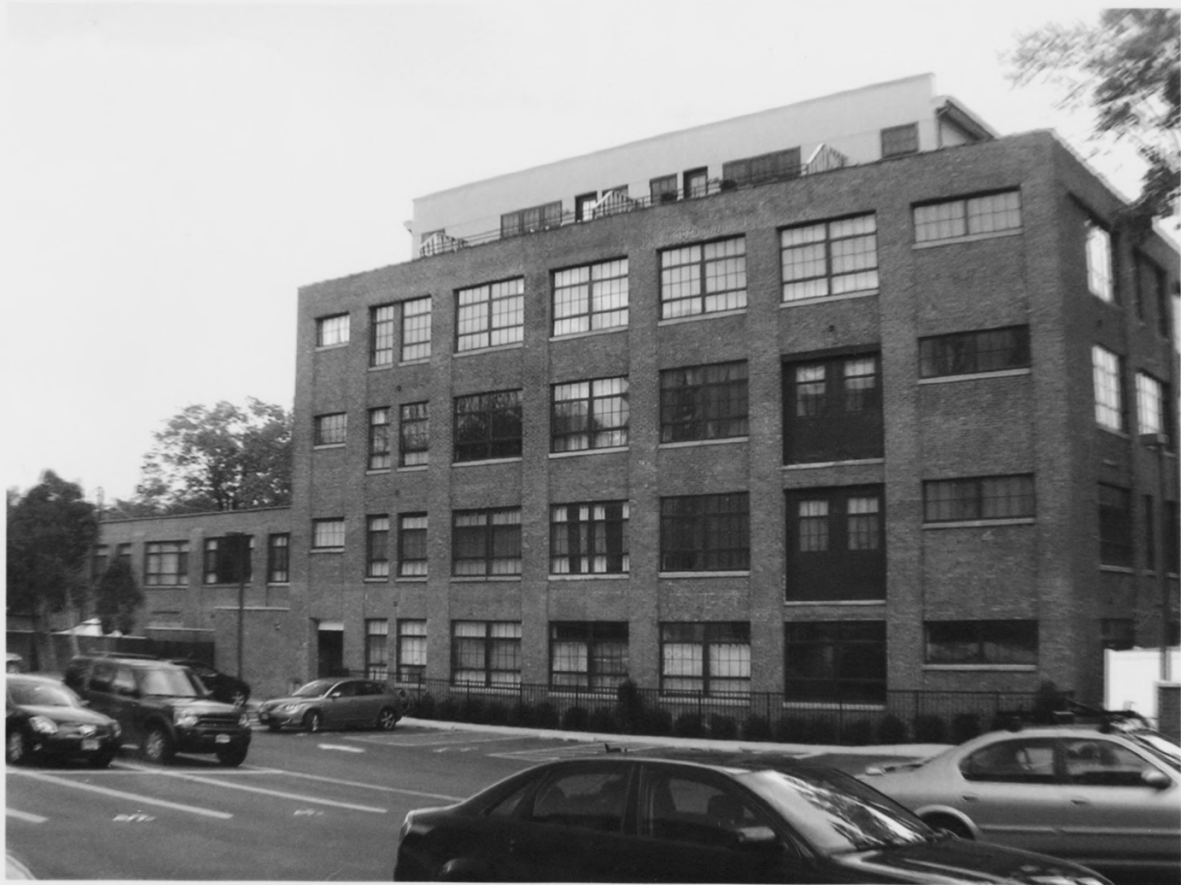
Interstate Hosiery Mills, Inc. Mill Building, Twp. of Bloomfield, Essex County, NJ
