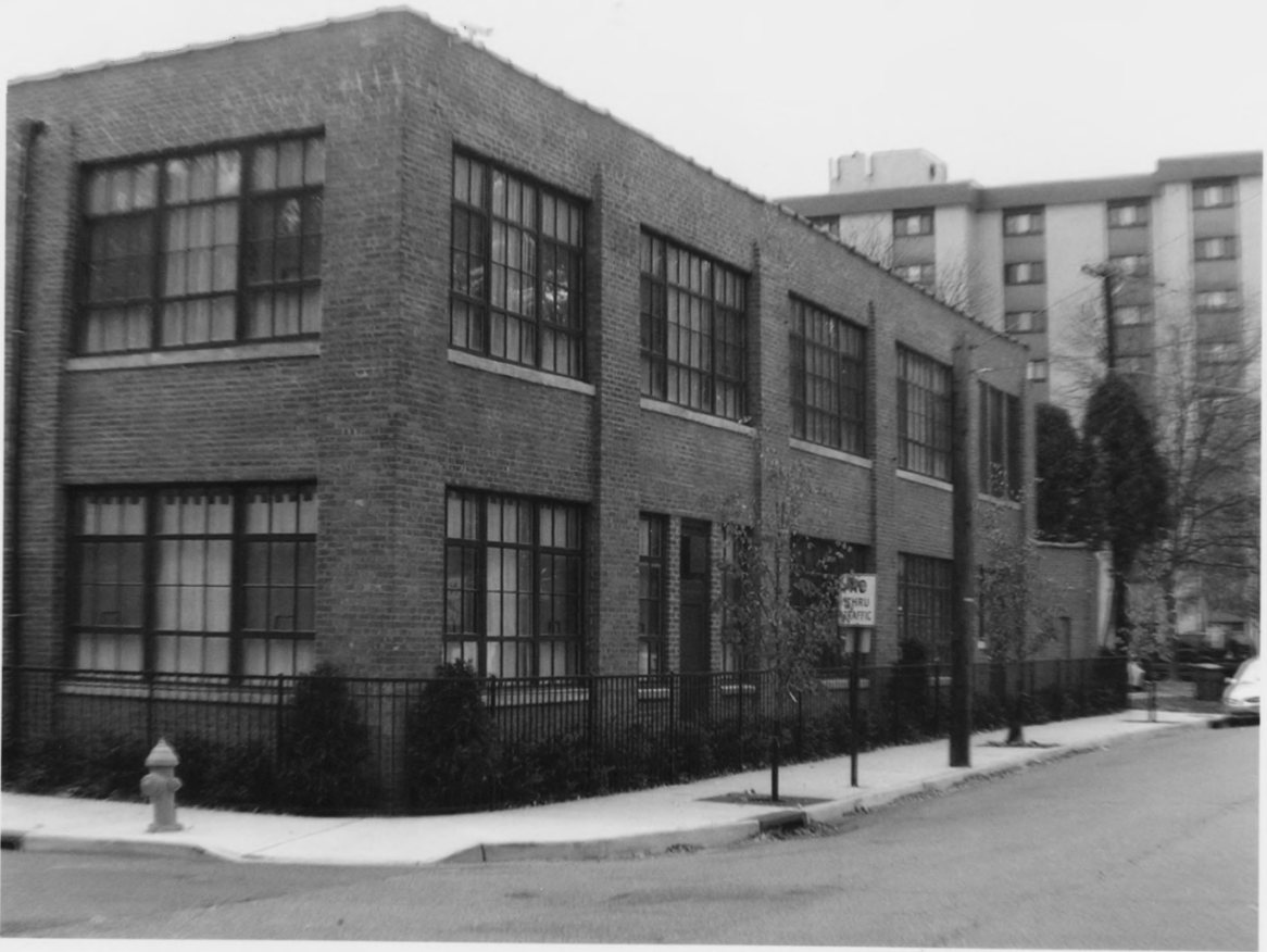
Interstate Hosiery Mills, Inc. Mill Building, Twp. of Bloomfield, Essex County, NJ
