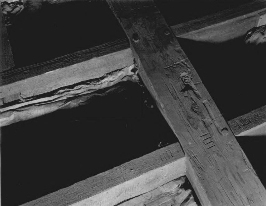
Photographer: James R. Lockhart Negative Filed: Georgia Department of Natural Resources Date: November, 1981 Detail of joist Description (10 of 16): construction in attic, showing Roman Numerals.
