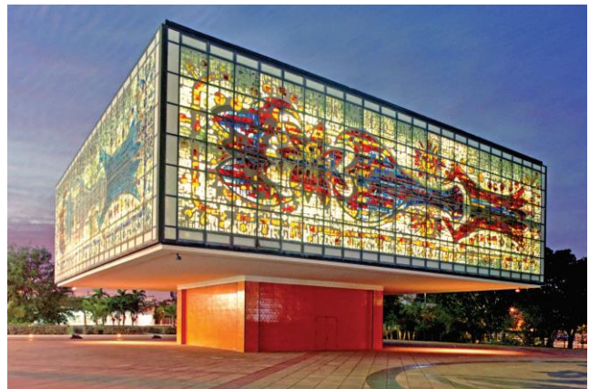
Figure 12: 1973 nighttime photograph of the Bacardi Imports Administration Annex, illuminated. Source: The Bacardi Archive
