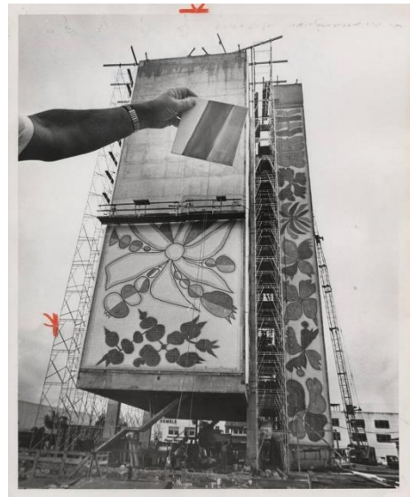
Figure 9: 1963 Miami Herald photograph of the Bacardi Imports Tower under construction, with the tilework underway on the south side of the building. Source: Miami Herald
