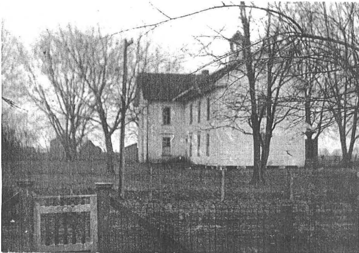
Figure 1: 1895 addition on east side of main building. Date: Unknown. Source: Jill Williamson, Harrisburg Community Betterment Association, Personal Collection
